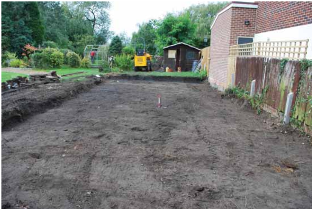
Plate 2. Site post- excavation of turf, facing west
