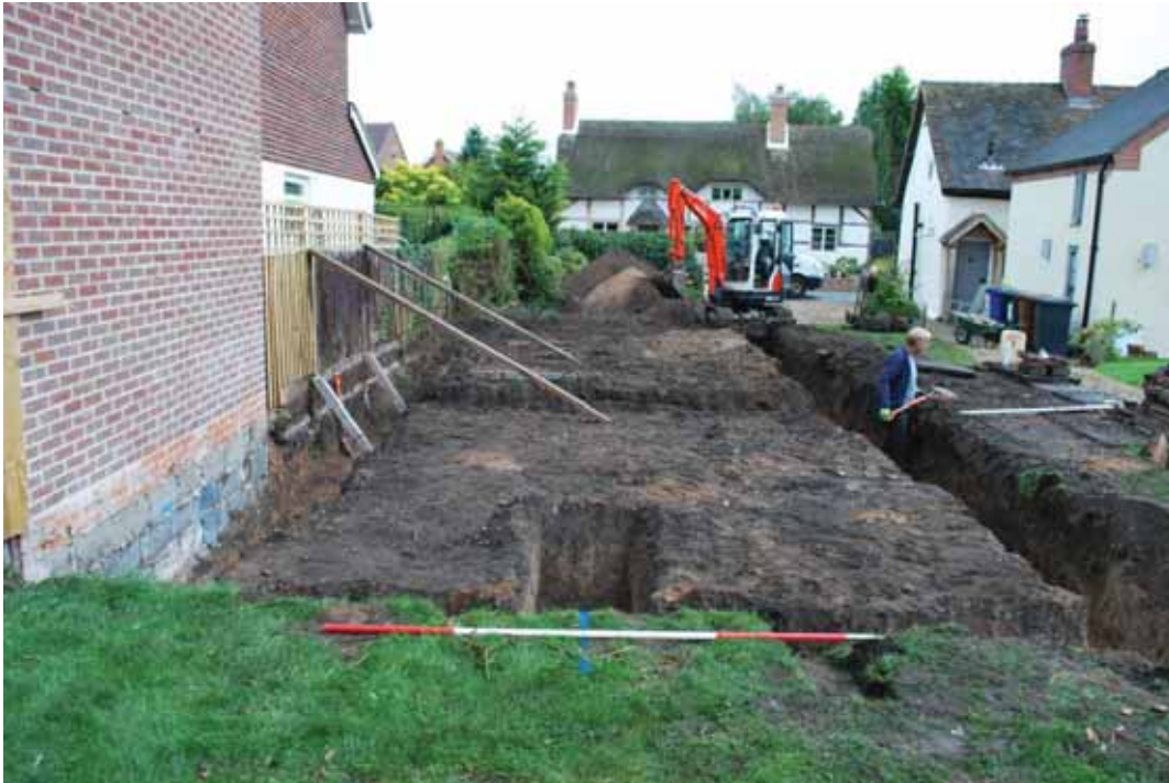
Plate 3. Site post excavation of foundation trenches, facing east
