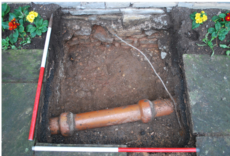
Plate 14: Test Pit 5. Metallised Surface 508. Looking West
