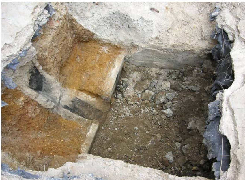
Photo 11, Trench 7, looking south. 19/20th-century backfilled basement and associated coal chute, truncating natural gravels.
