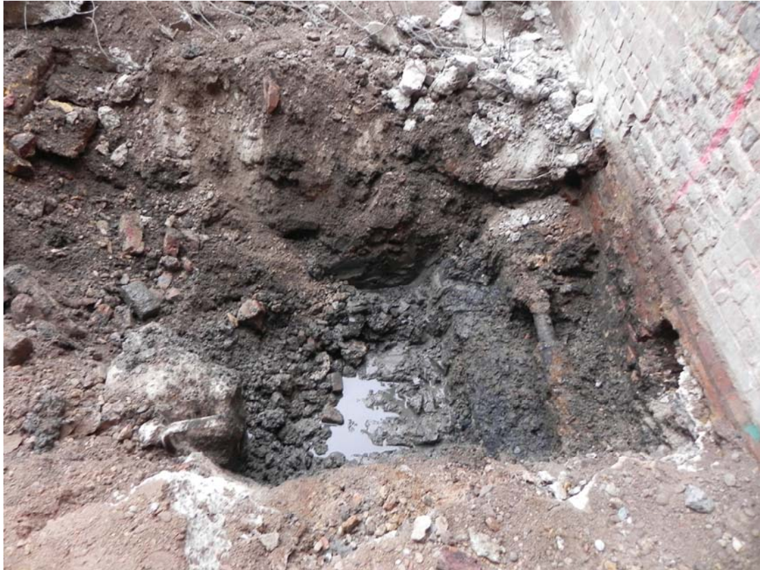
Test Pit TP/F4, looking south, showing wall foundations [31]
