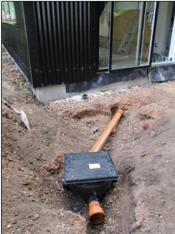
Plate 13 General view showing completed new drainage trench and new drains laid at northeast corner of new office building, looking south
