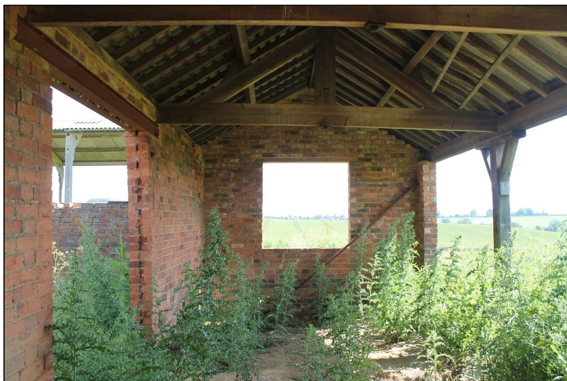
Plate 26 Interior of Room 5, looking south
