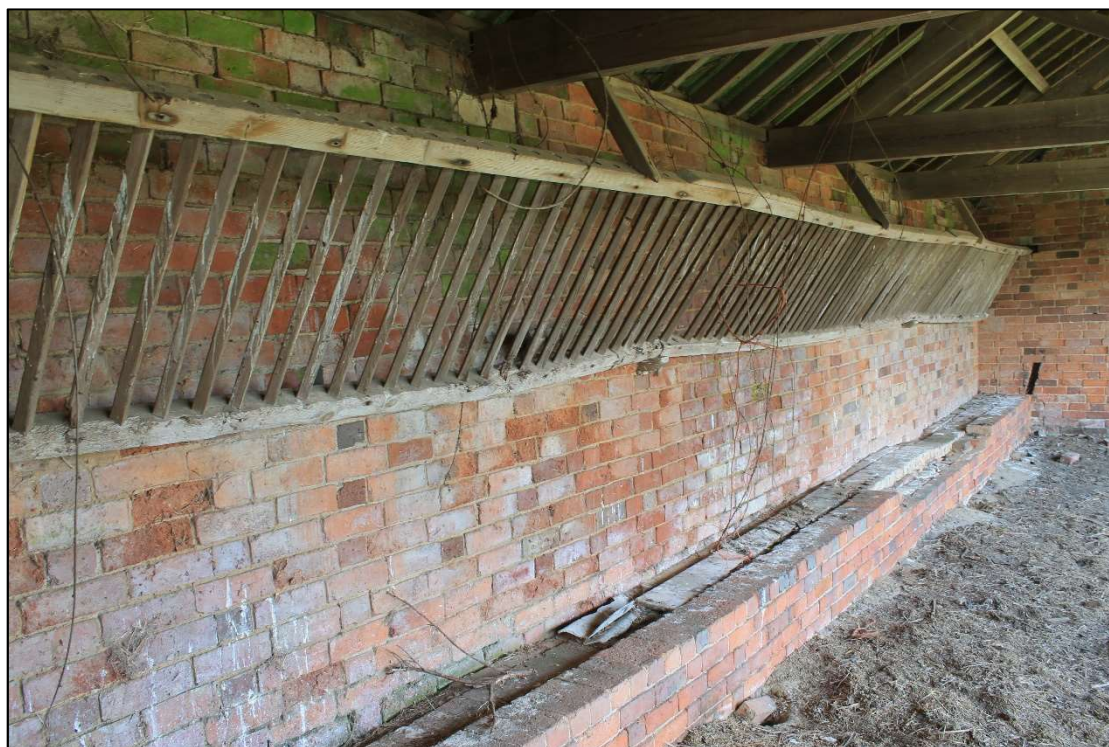
Plate 10 Hay rack and manger along north wall of cattle shelter, Room 2, looking northeast
