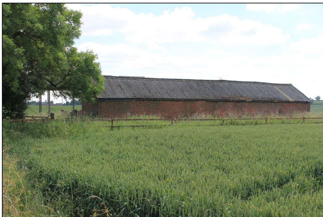
Plate 4 Plain north elevation of brick structure, looking southwest
