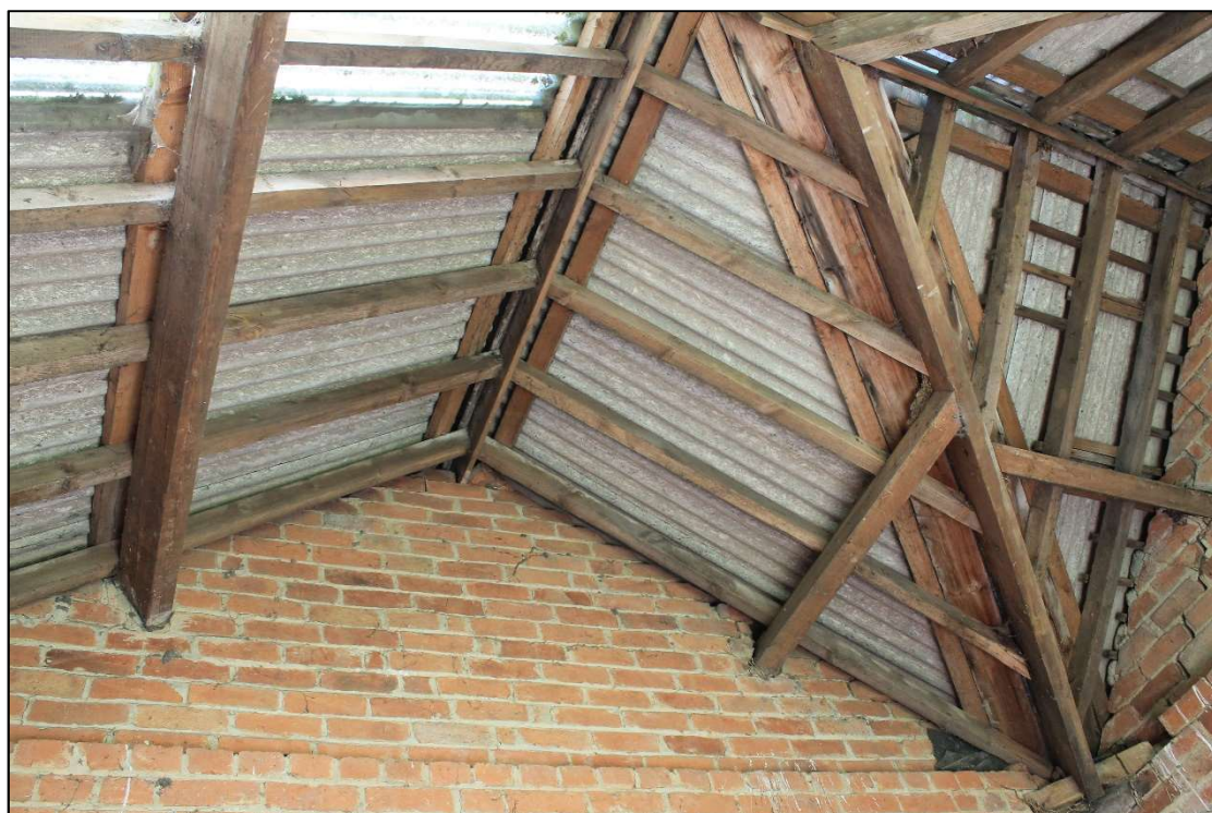
Plate 29 Detail of roof structure in Room 4, looking east
