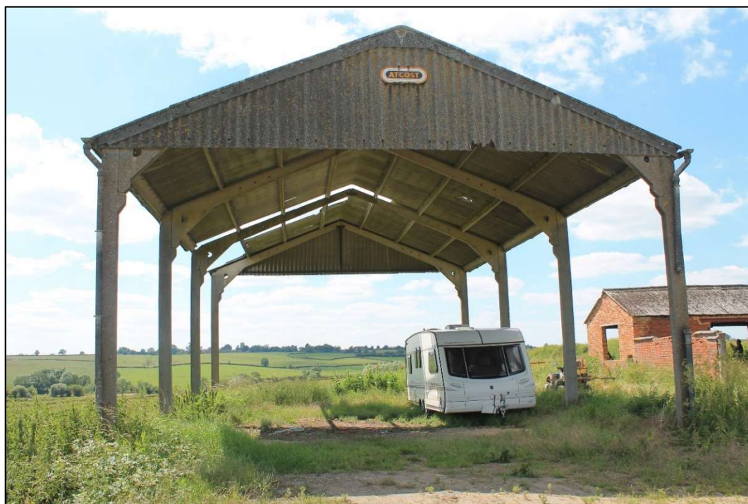
Plate 32 East gable of Dutch Barn, Room 1, looking west
