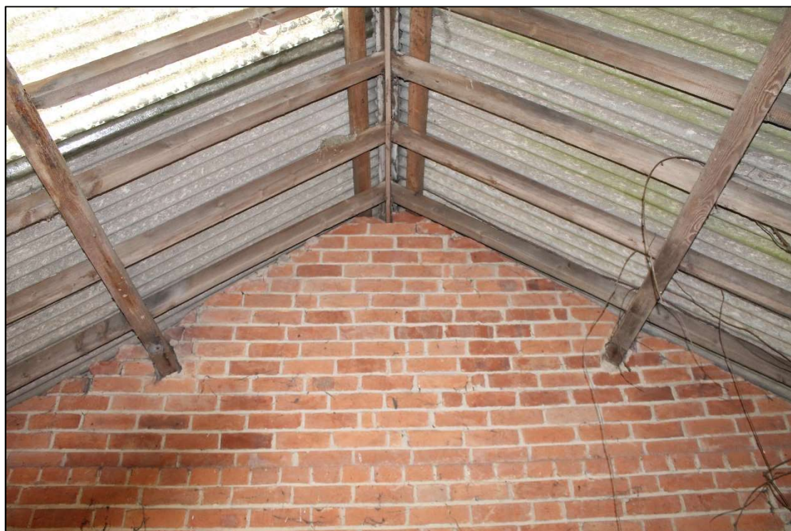
Plate 21 Detail of roof structure in Room 3, looking west
