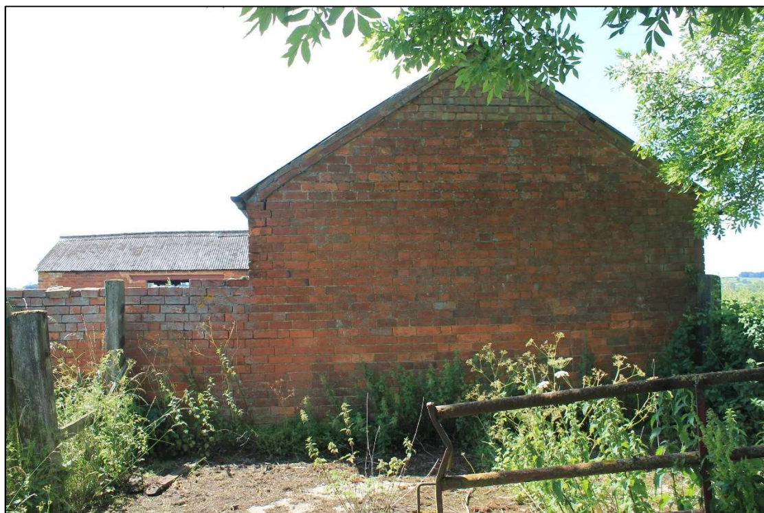
Plate 5 East gable of cattle shelter, Room 2, looking west
