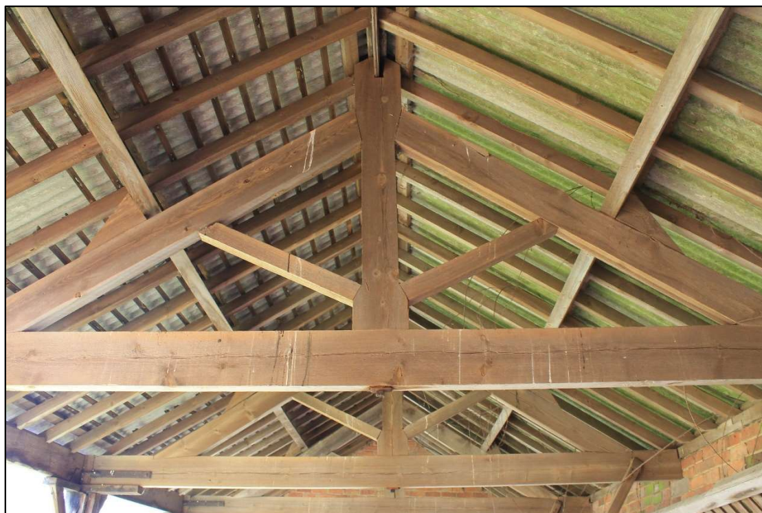
Plate 9 Detail of roof structure of cattle shelter, Room 2, looking west
