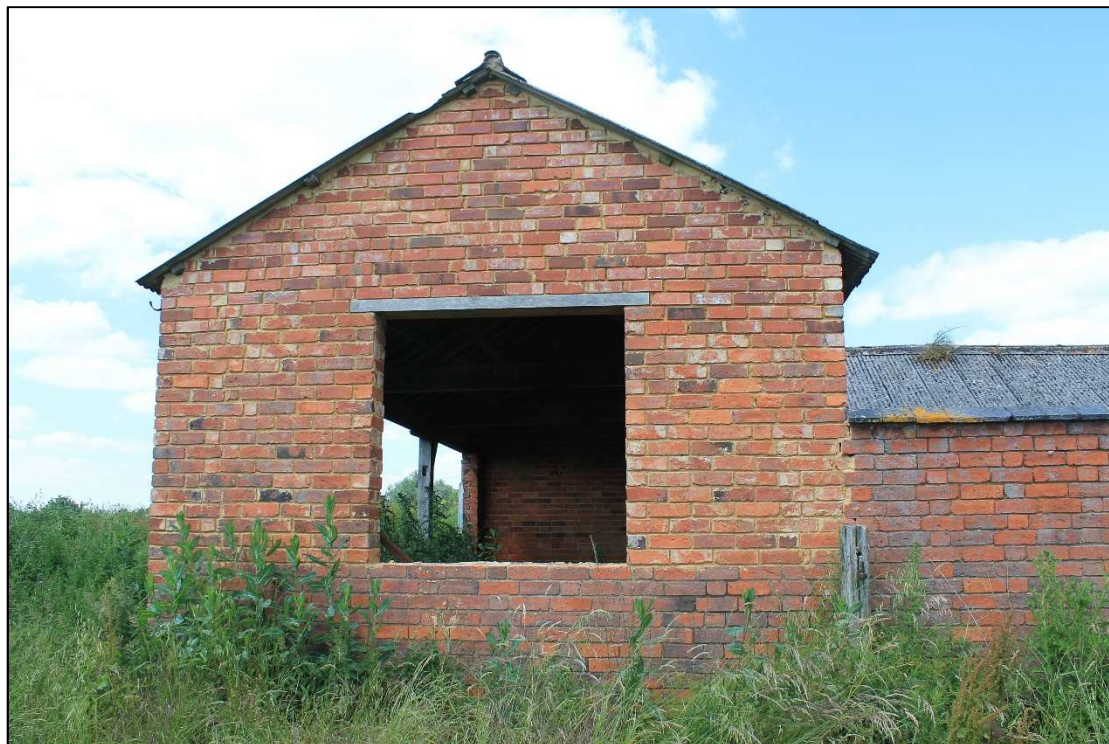
Plate 24 Substantially-rebuilt south gable of Room 5, looking north
