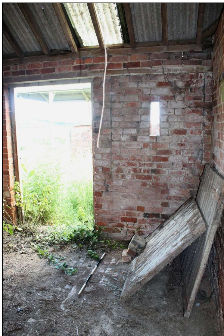
Plate 17 Interior of Room 3, showing brick floor, blocked window and inserted breather slit, looking south, Scale 1m
