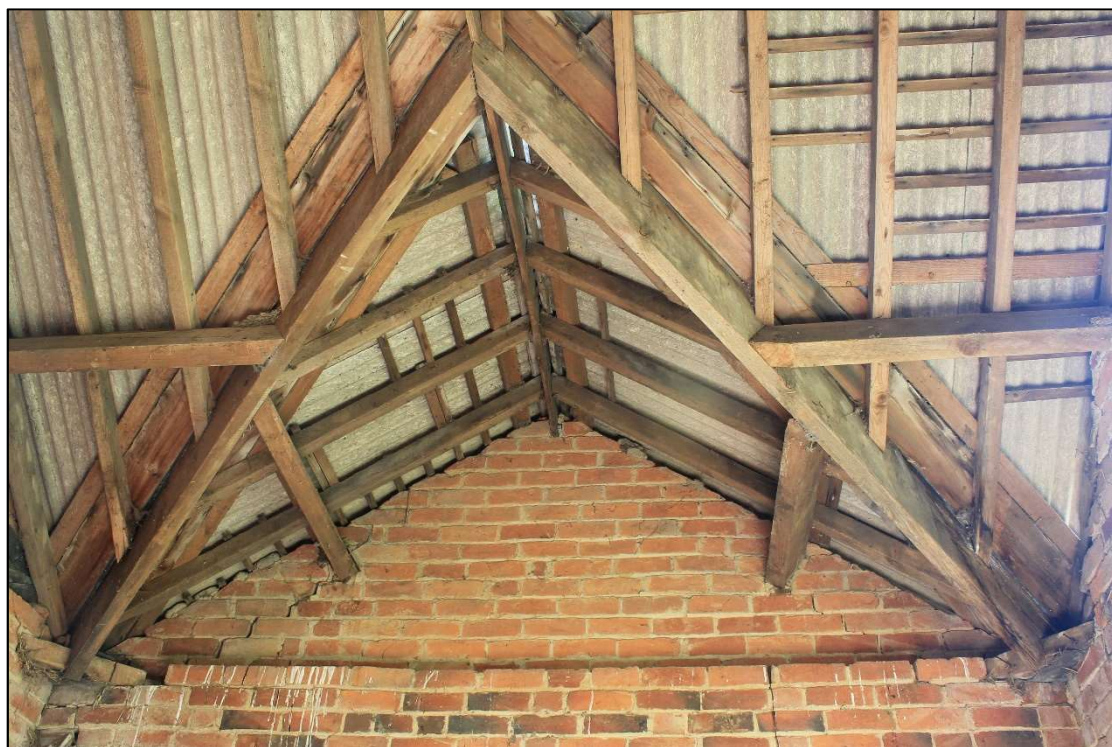
Plate 28 Detail of roof structure in Room 4, looking south
