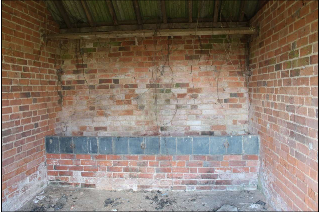
Plate 18 Brick manger with iron tethering rings and remnants of hay rack inside Room 3, looking north
