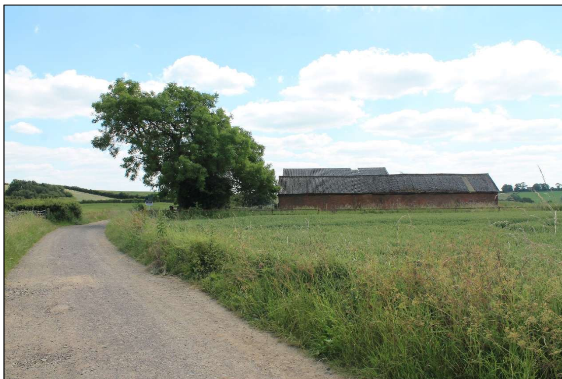
Plate 1 General view of recorded buildings, looking south along lane
