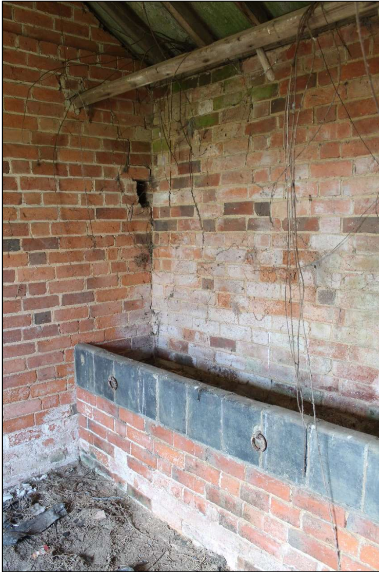
Plate 19 Detail of brick manger, iron tethering rings and remnants of hay rack in Room 3, looking northwest
