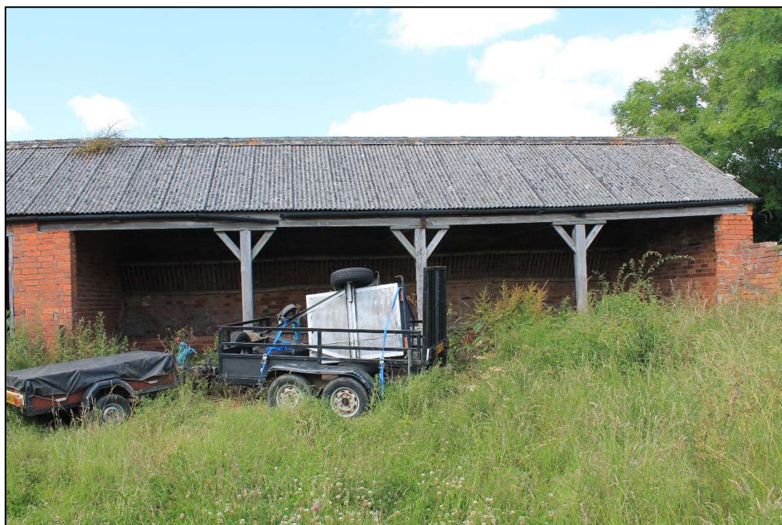
Plate 6 South elevation of cattle shelter, Room 2, looking north
