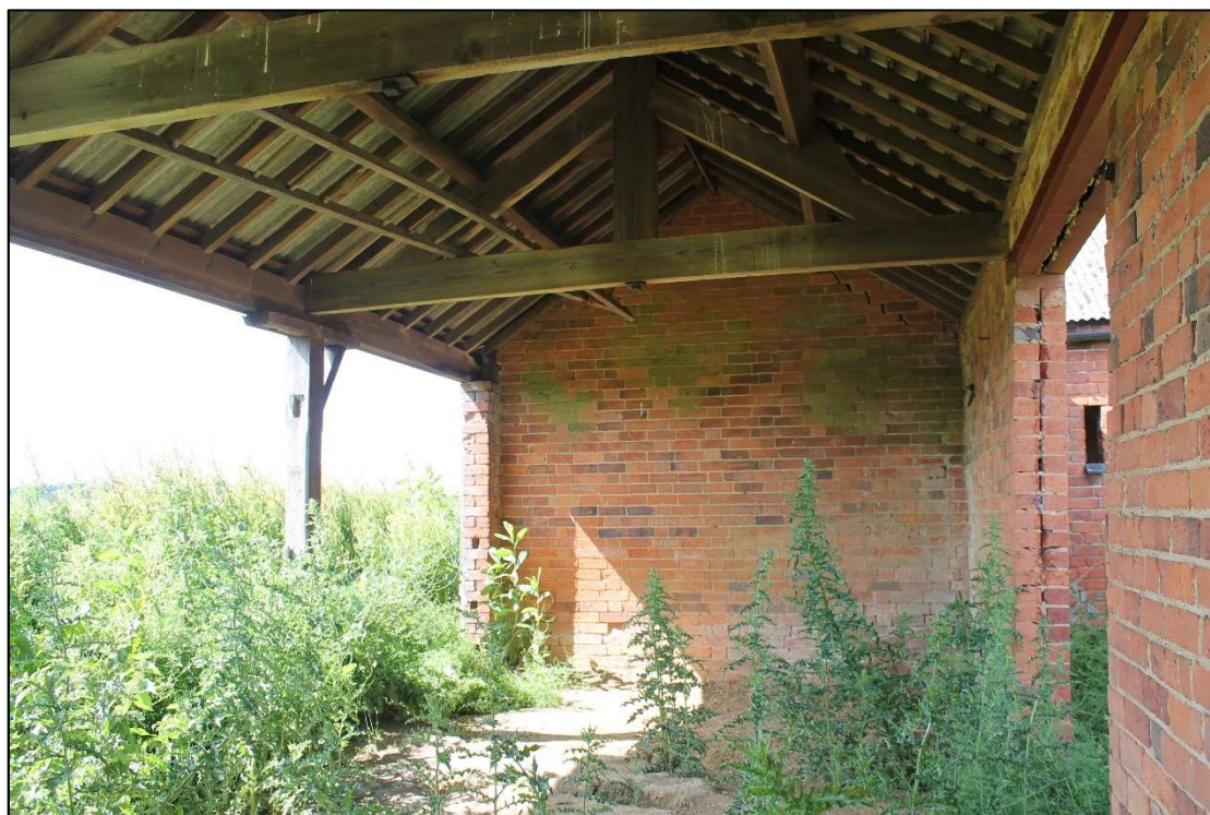
Plate 25 Interior of Room 5, looking north
