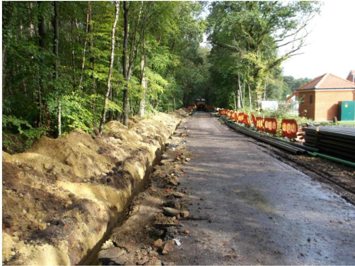
Plate 1: General view of Area 1, looking north-east
