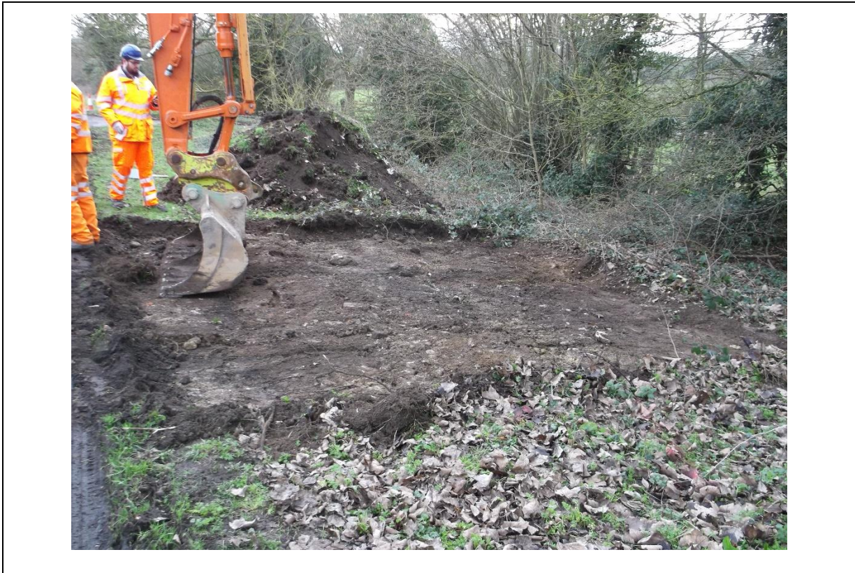
Plate 1: Topsoil Strip of Manhole 01 looking south
