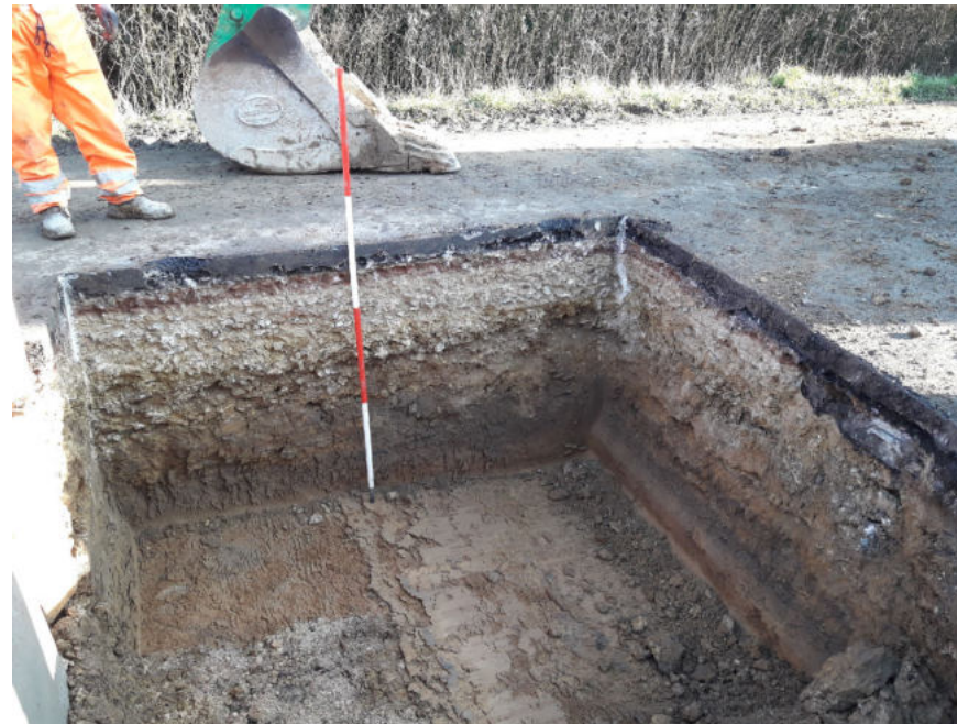
Plate 6: West facing section of Manhole 03
