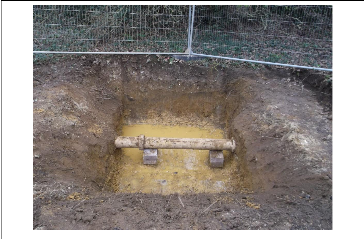
Plate 2: Post-excavation shot of Manhole 01 showing stratigraphy looking south-west
