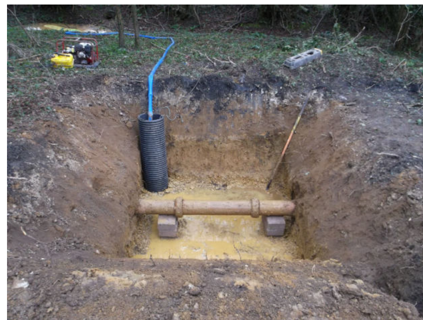
Plate 8: North facing section of Manhole 04
