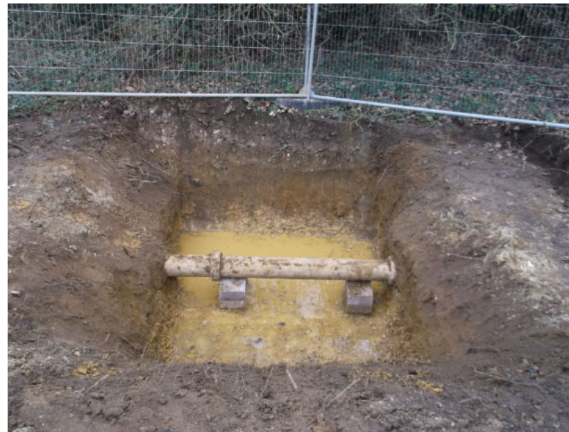
Plate 2: North-east facing section of Manhole 01
