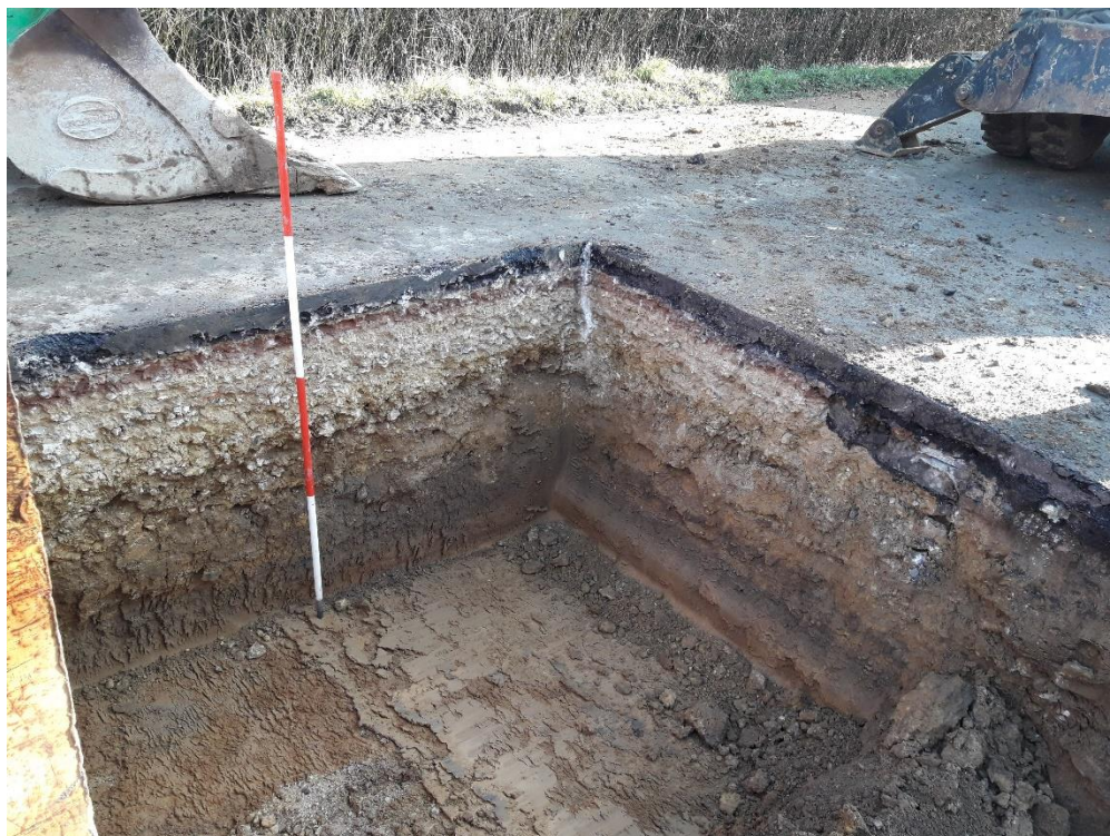
Plate 6: Oblique working shot of Manhole 03 showing stratigraphy looking east
