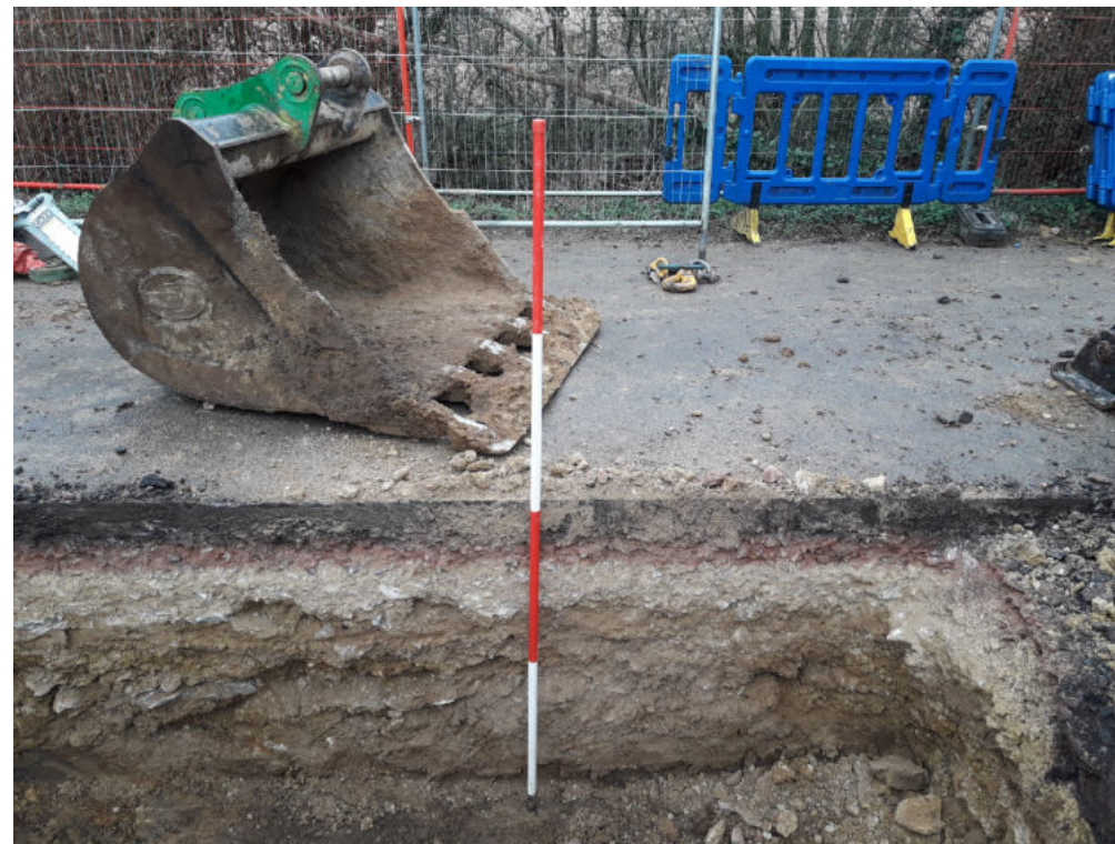
Plate 9: South-west facing section of the sewer trench
