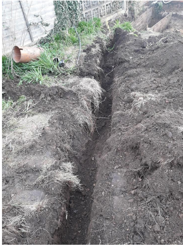
Plate 7: North-west facing view of the new drainage trench connecting the new extension to rear of the house to the new soakaway in the rear garden.
