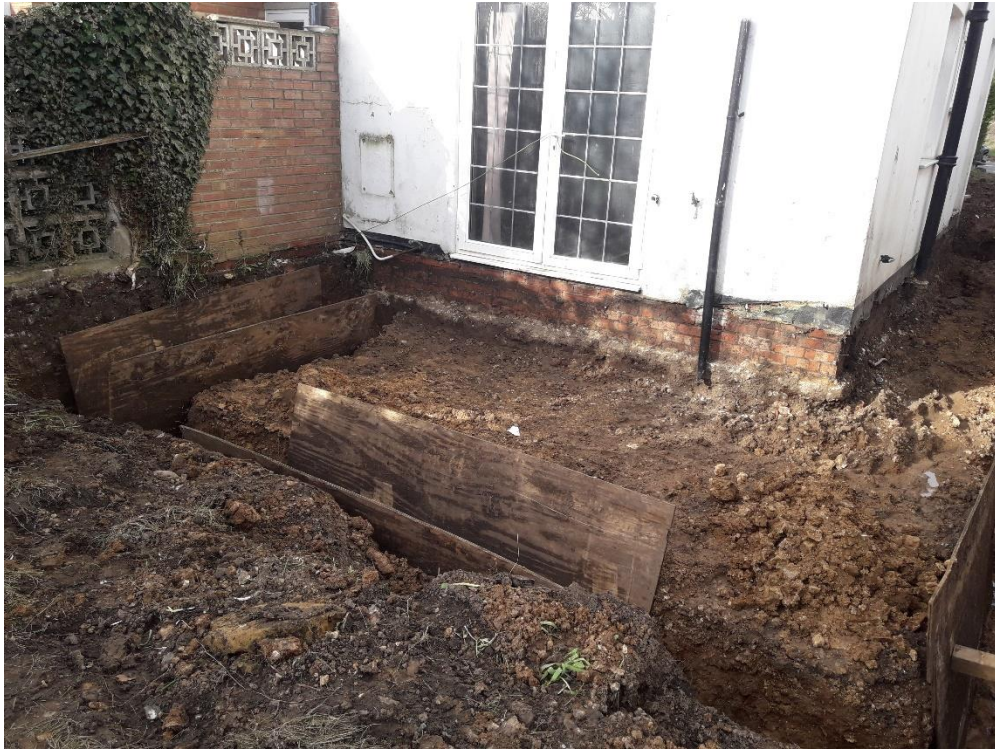
Plate 5: North-west facing view of the excavated area and footing trenches to the rear of the house.
