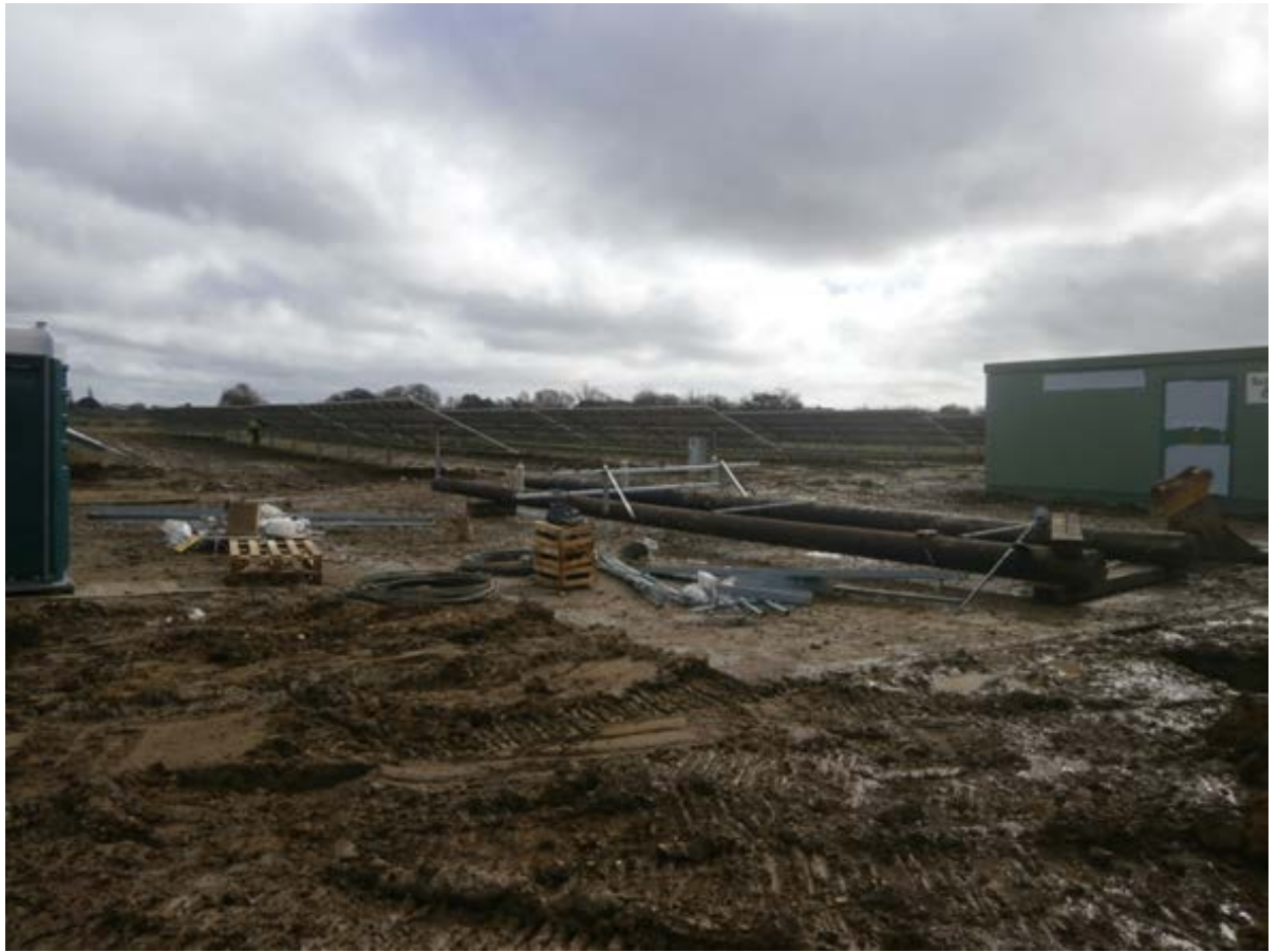
Plate 10: General shot of the solar farm development looking south.
