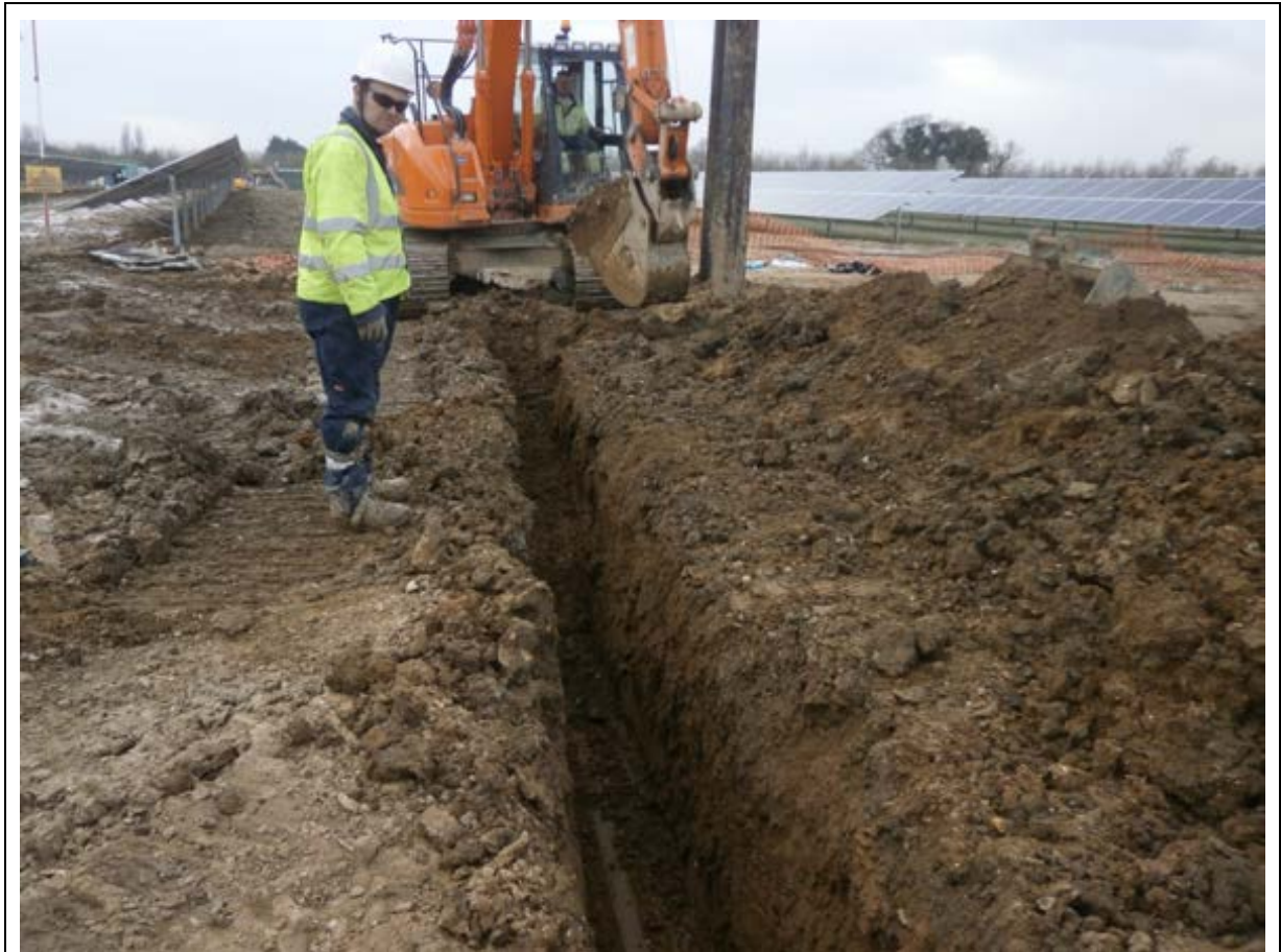
Plate 7: General shot looking north-west of the new cable trench being excavated.
