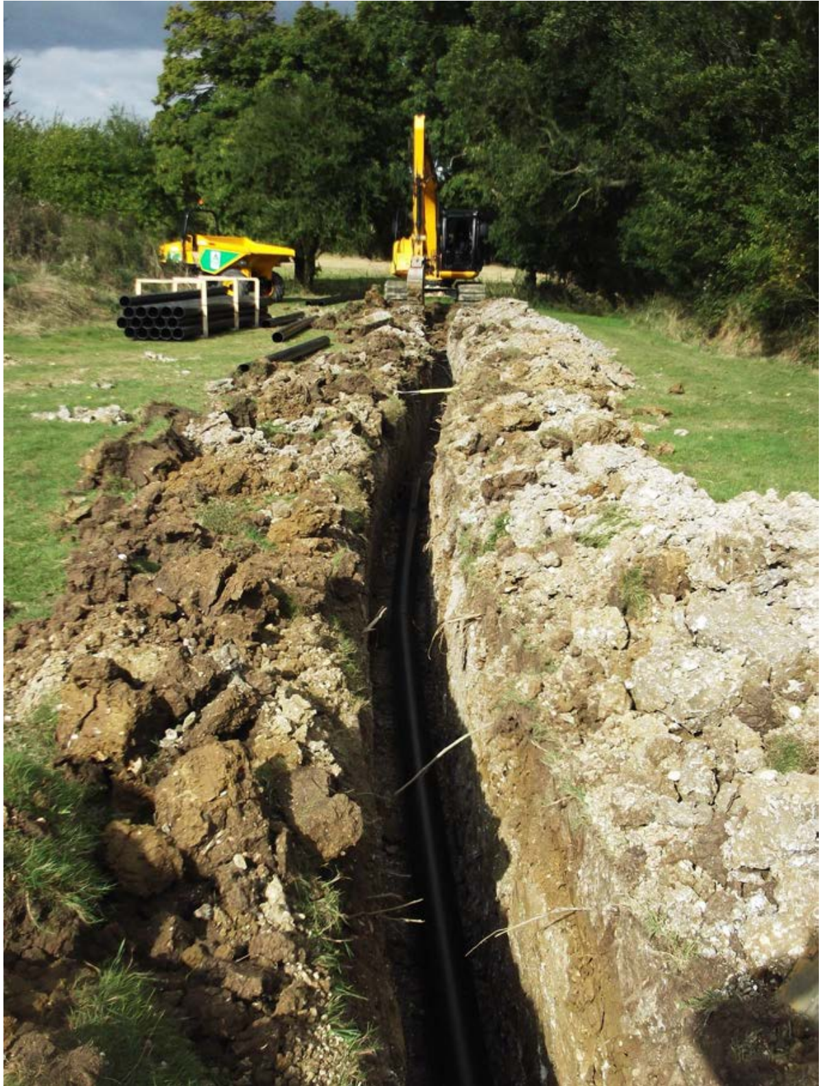
Plate 5: View of the Trench 1 being excavated to the north-east of Friar's Farm, looking west.
