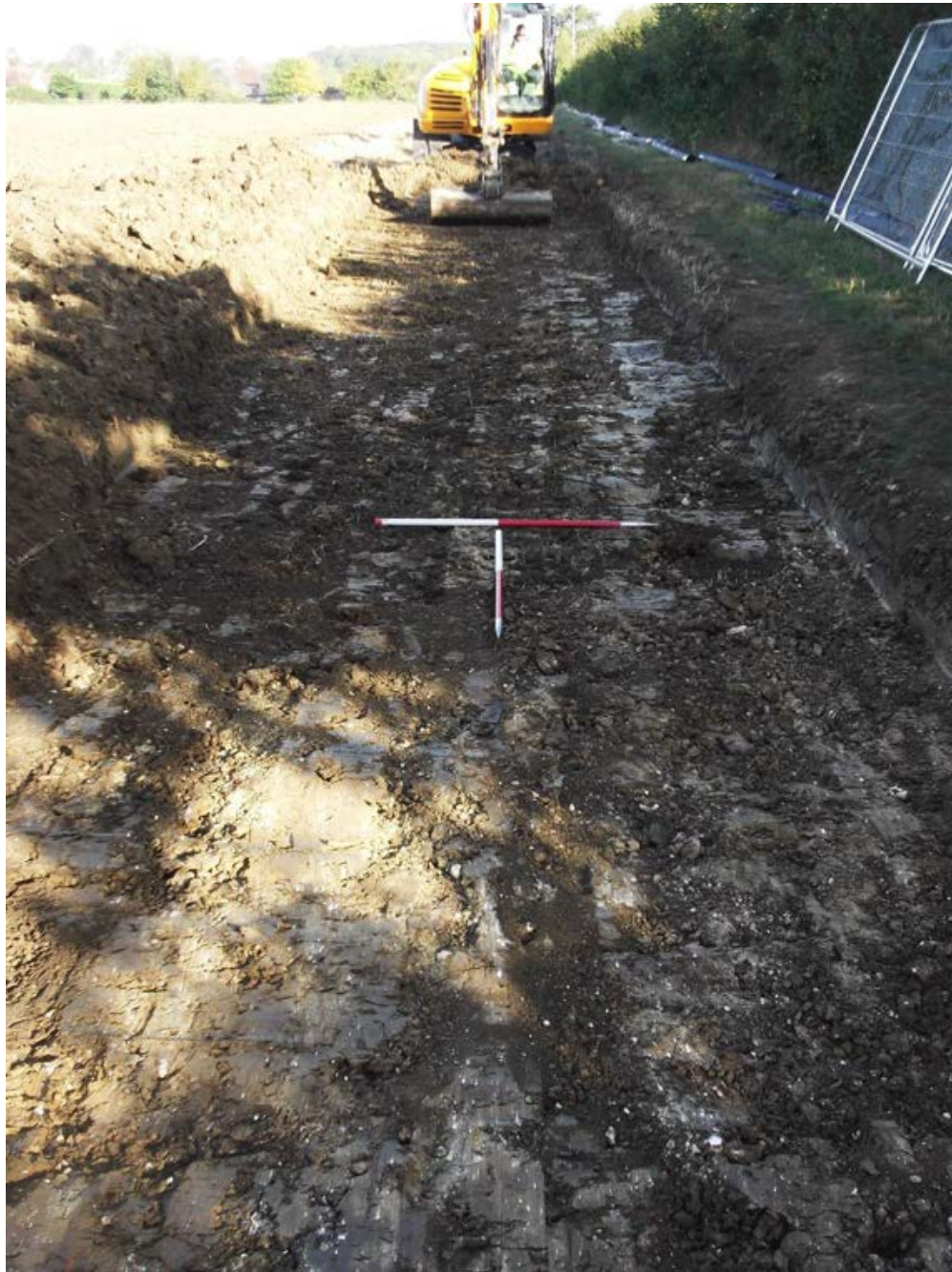
Plate 2: General shot of the easement trench to the south of Friar's Farm, looking north-west.
