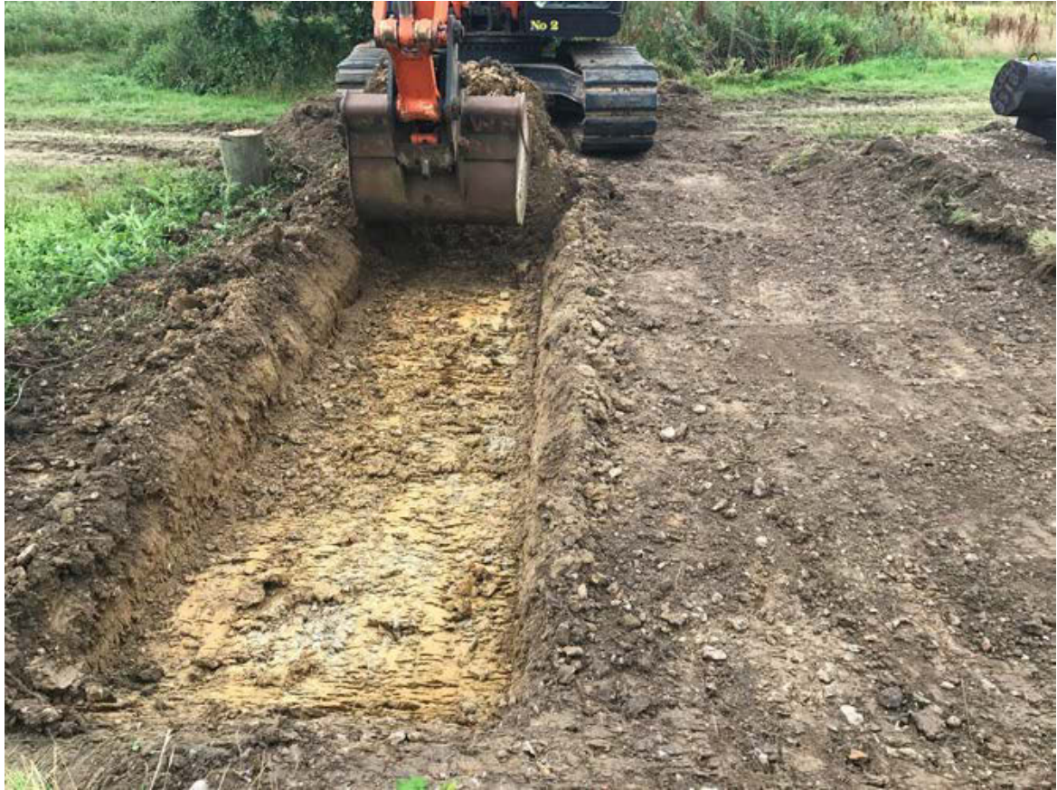
Plate 5: General shot of trench being excavated at Pole 27, looking south-east.
