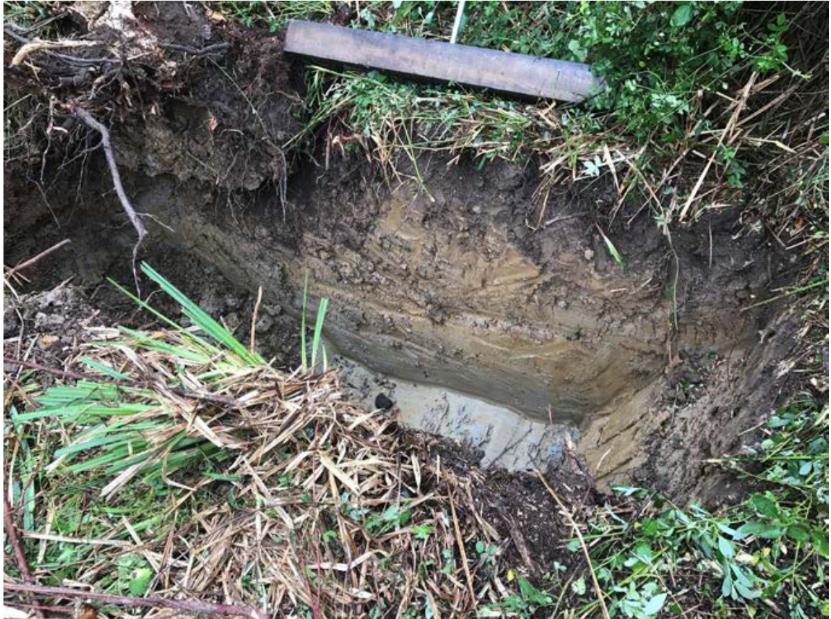
Plate 4: General shot of a stay hole at Pole 32, looking south-west.
