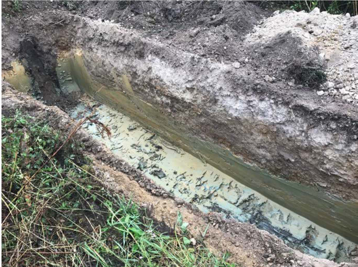
Plate 2: General shot of trench at Pole 26, looking north-east.
