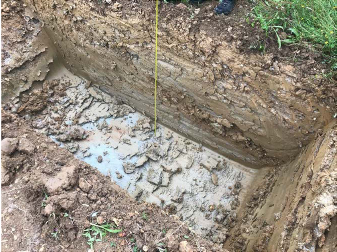
Plate 3: General shot of a stay hole at Pole 29, looking north-east.
