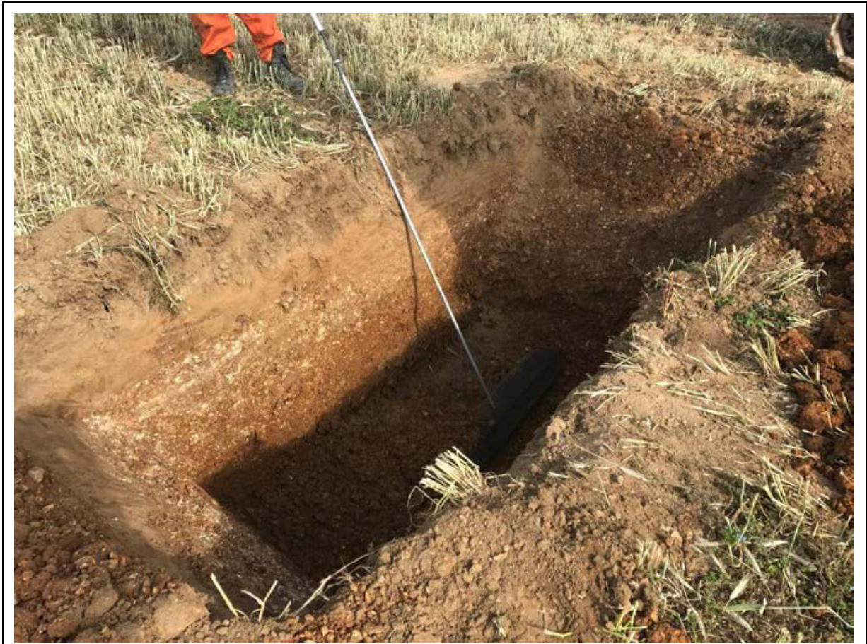
Plate 1: General shot of a stay hole at Pole 24, looking north-west.
