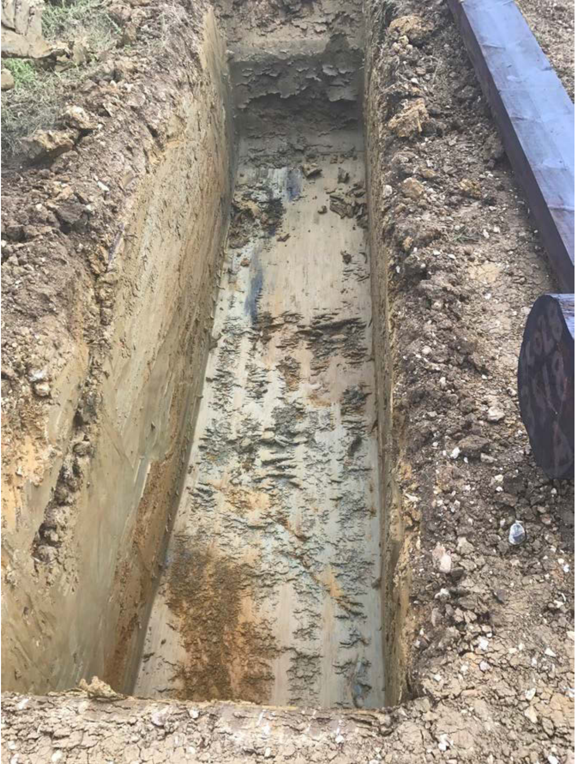
Plate 6: View of excavated trench adjacent to Pole 28 and Palaeochannel (2803) at its base, looking south-east.
