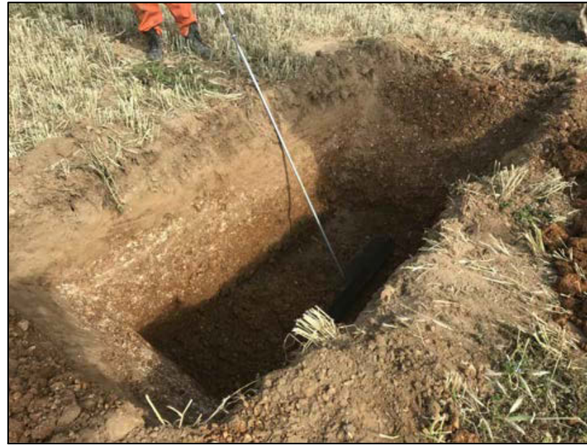
Plate 1: General shot of of stay hole at Pole 24, looking north-west
