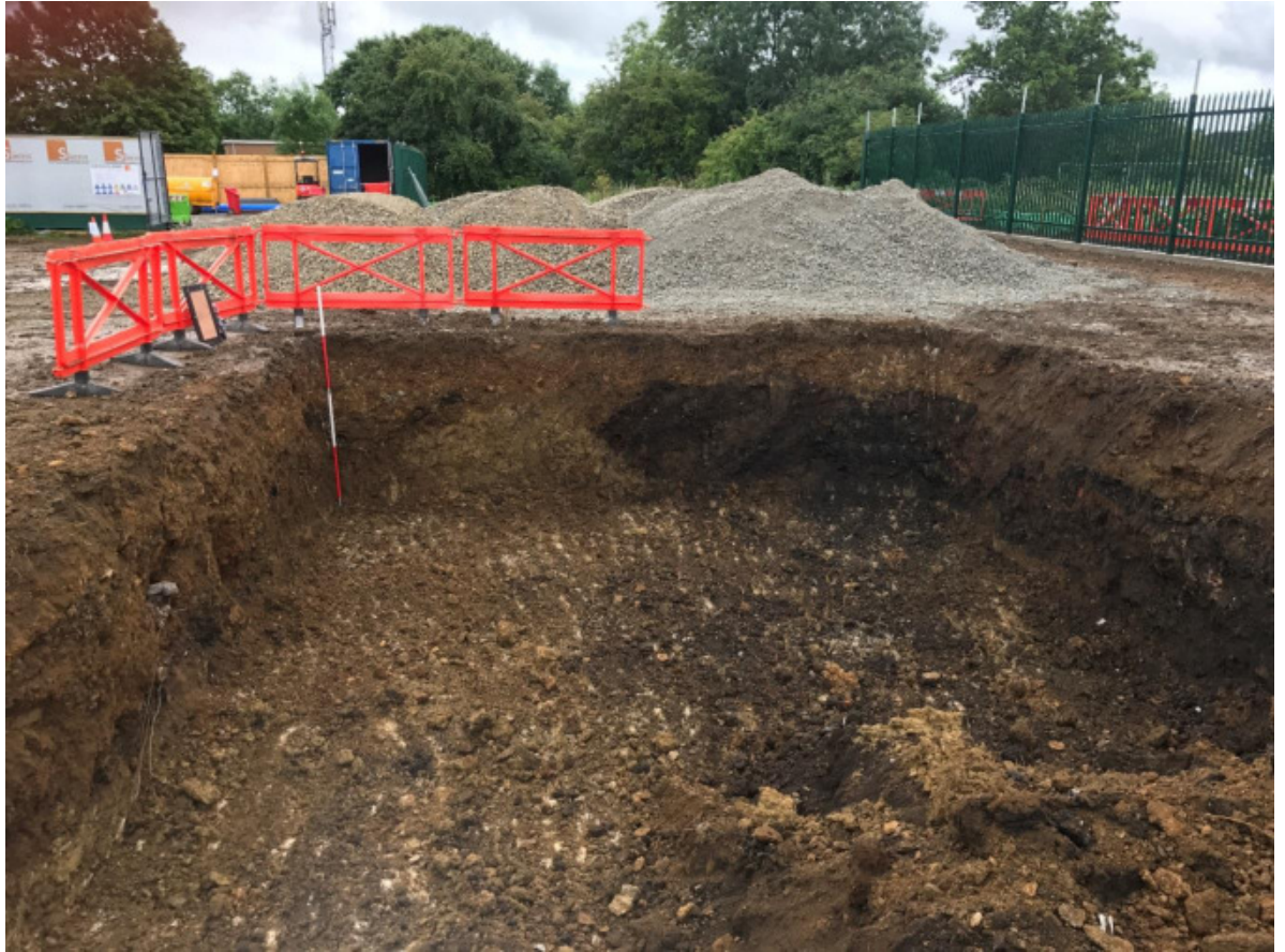
Plate 7: North-west facing section of Trench 6 (Transformer C2MT), looking south-east.
