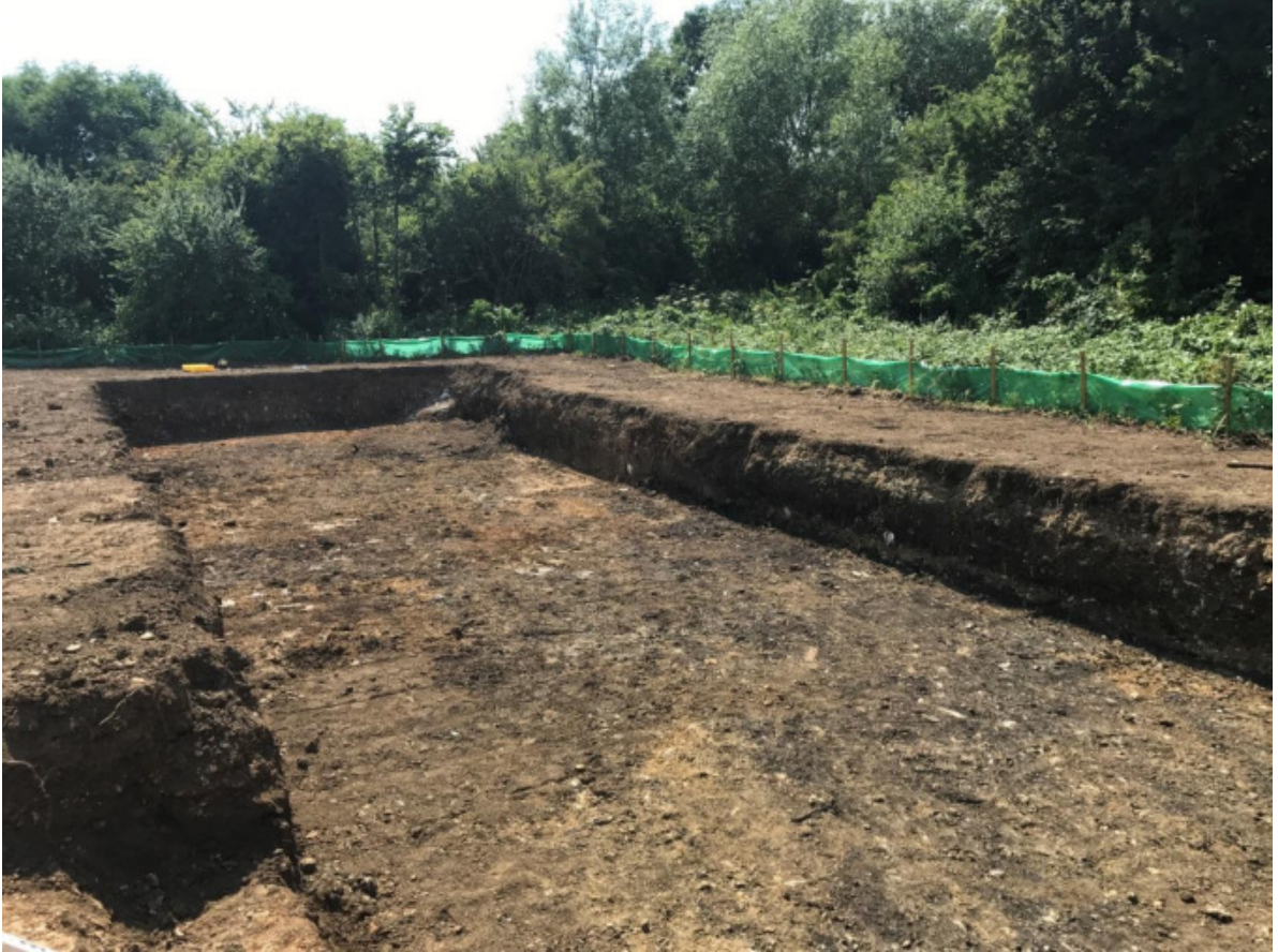
Plate 2: View of Trench 1 (the Switch House), looking south-east.
