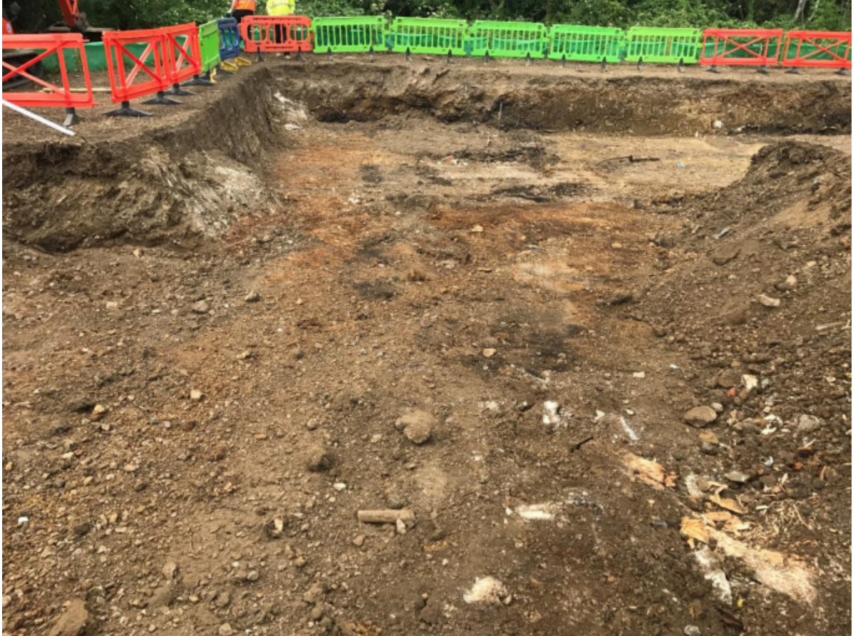
Plate 3: View of the Ditch 108 continuing into Trench 2 (the access road), looking east.
