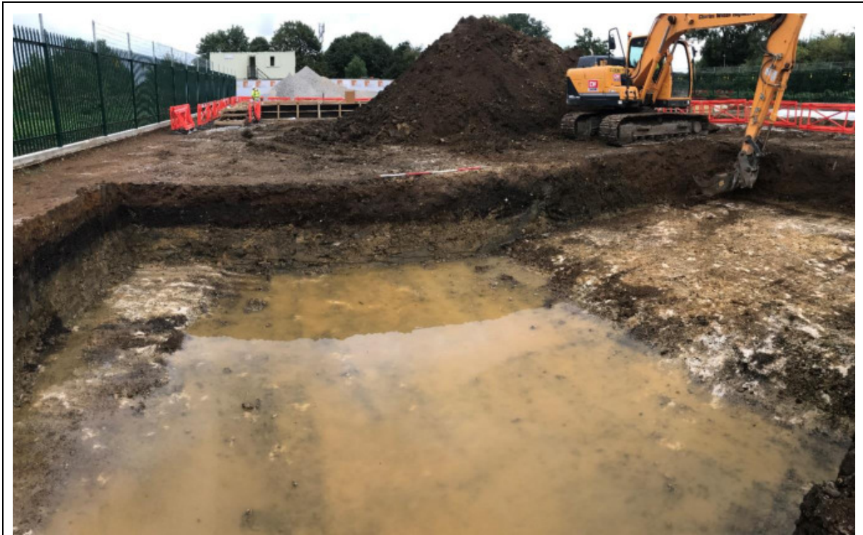
Plate 5: View of excavated Trench 5 (Transformer A1MT), looking east.
