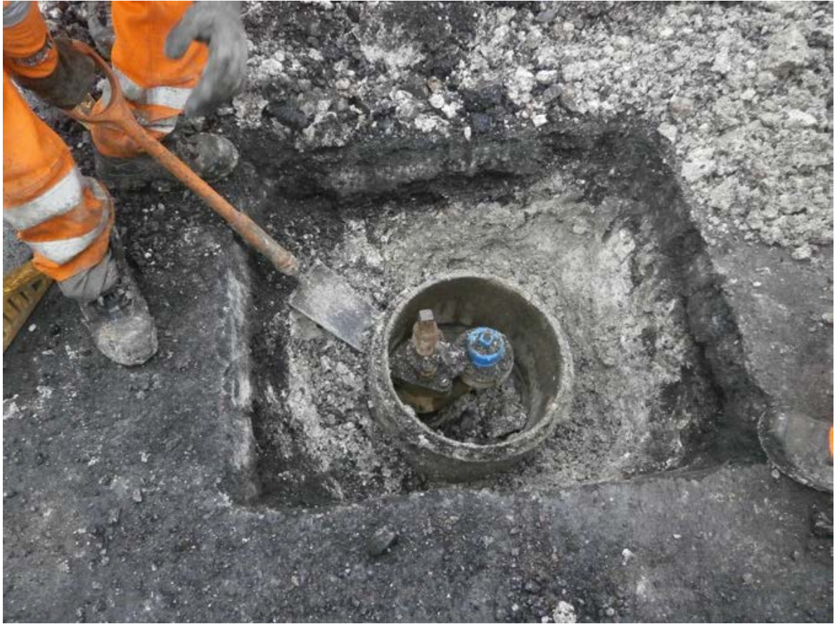
Plate 2: View of Trench 1 showing the modern concrete chamber (1004) and existing water hydrant (1005).
