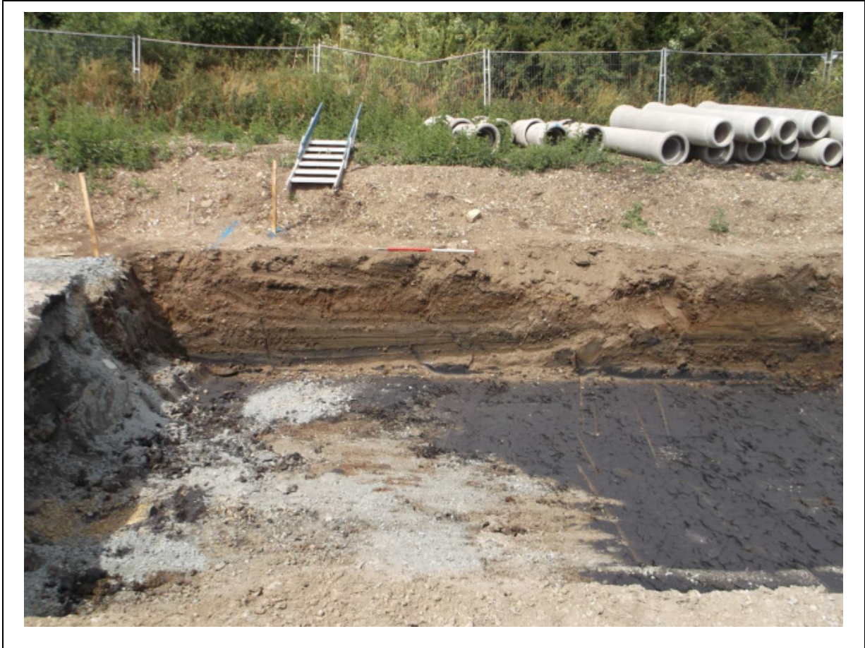
Plate 1: South facing section 1014 of Trench 23 (1 of 6, west end), looking north
