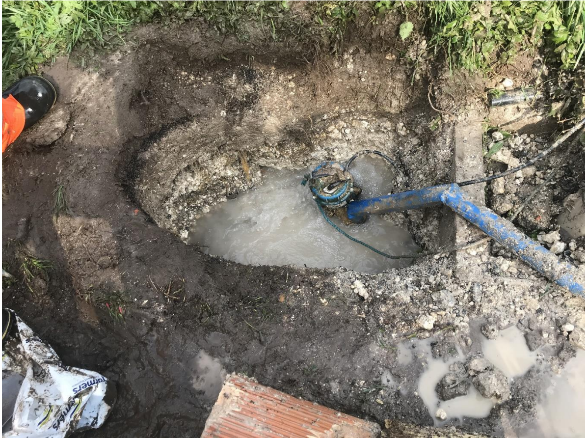
Plate 2: View of Trench 1 during hand excavation works.
