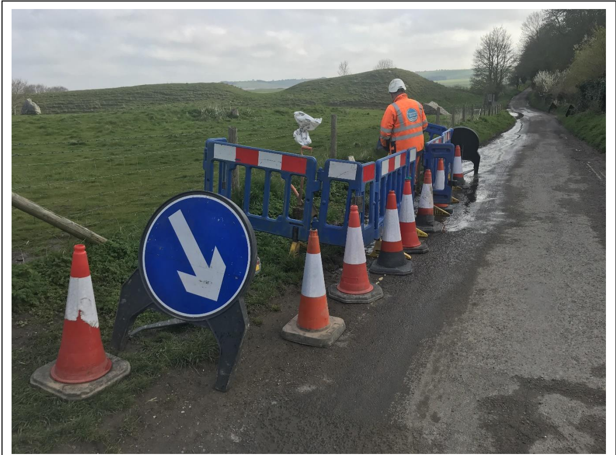
Plate 1: General view of Trench 1 taken along Green Street looking east with Avebury Henge in the background.
