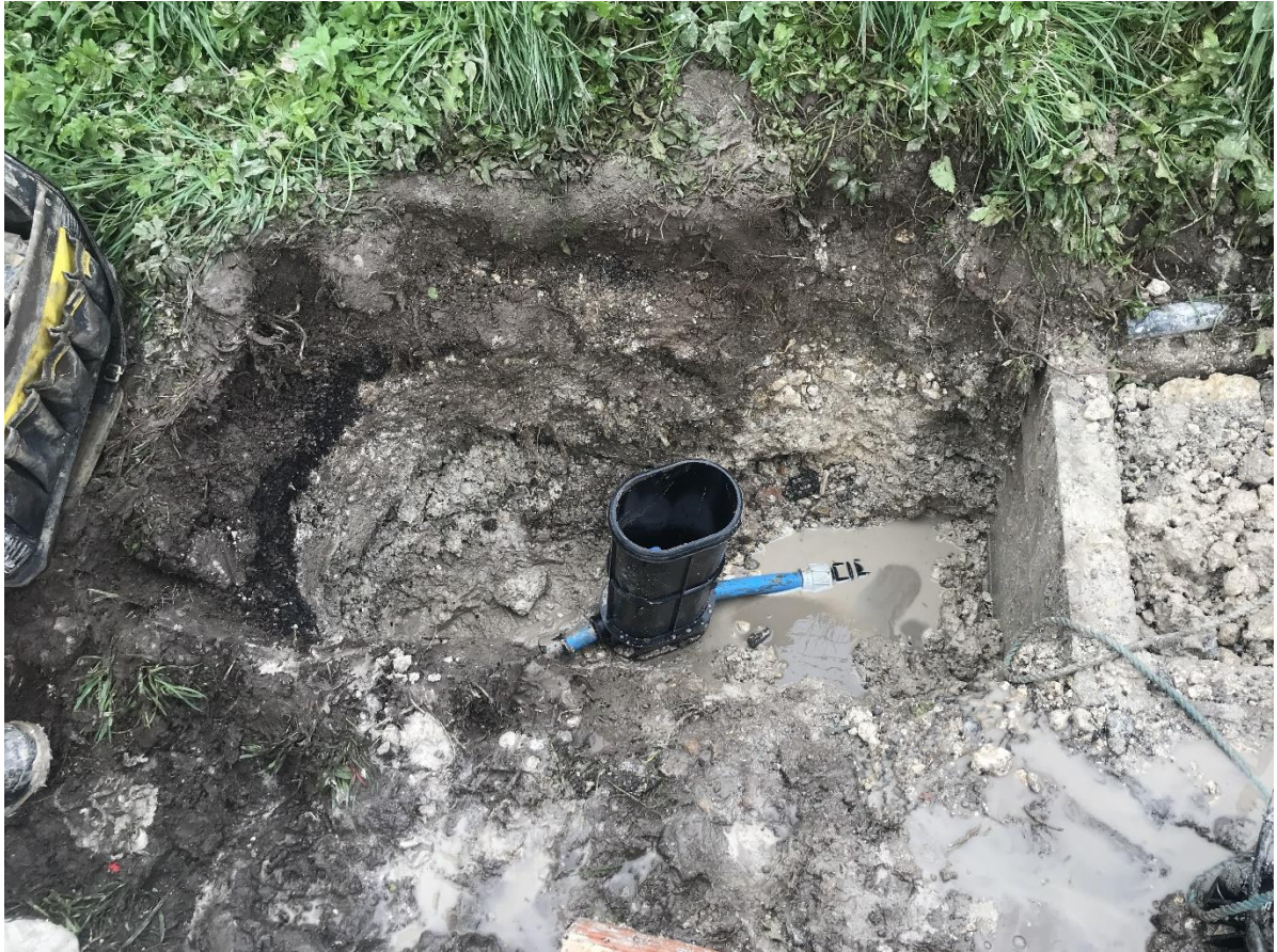
Plate 3: View of Trench 1 post-excitation with new pipe and box installed.
