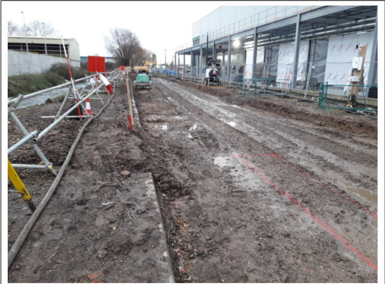
Plate 1: General view of the Northern Access, looking north-east
