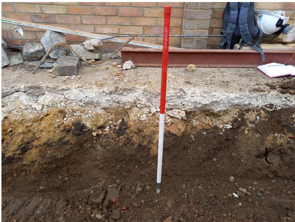
Plate 2: North-west facing view on site prior to Foundation Trench 2 excavation.
