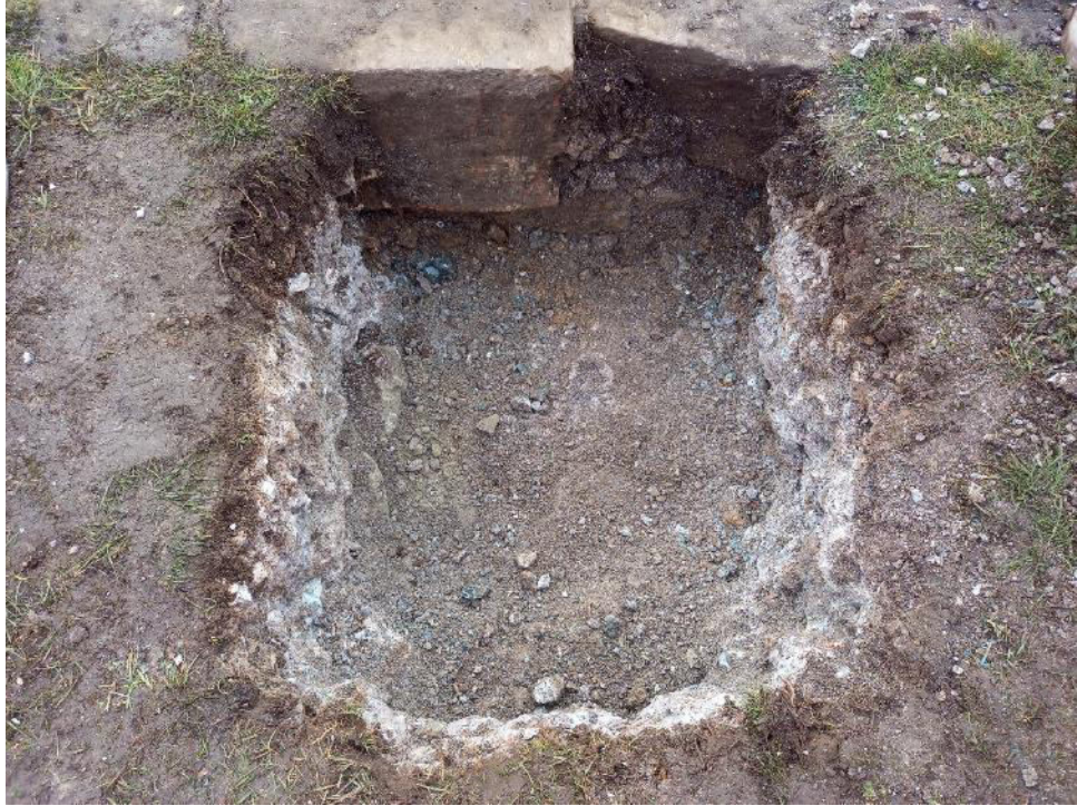
Plate 7: South facing view of Mooring Point 3.
