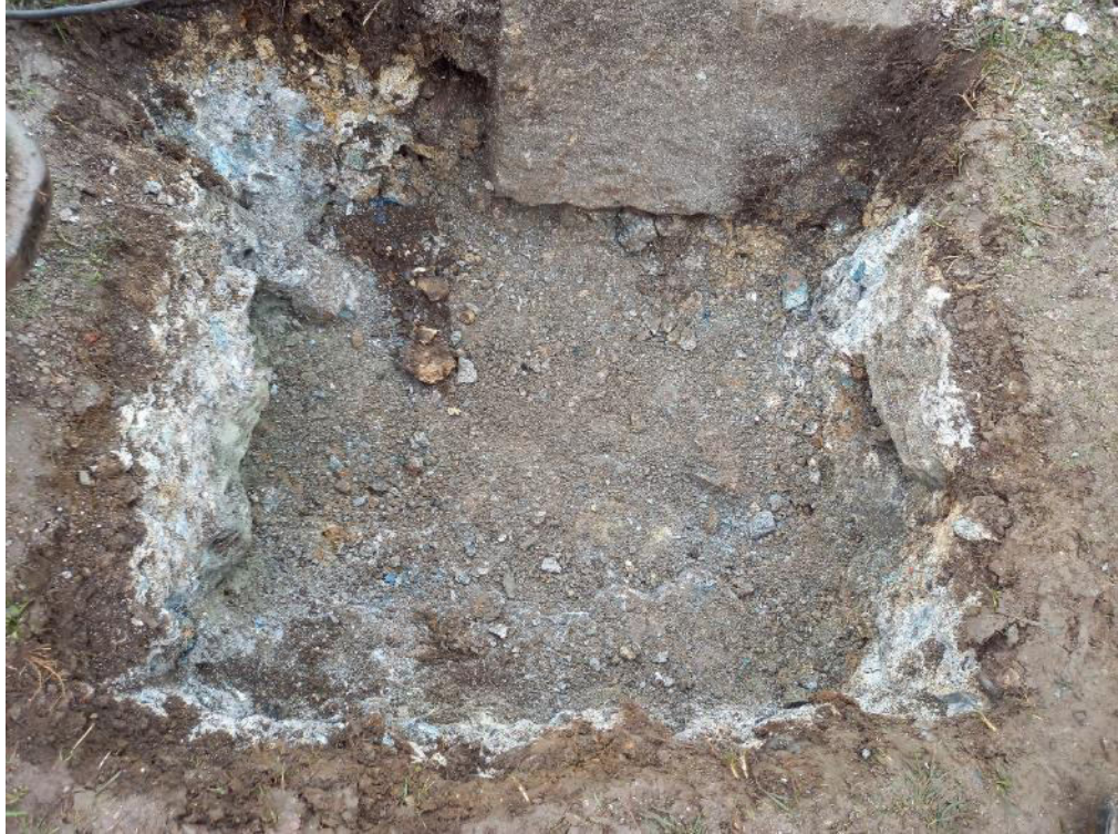
Plate 5: South facing view of Mooring Point 1.
