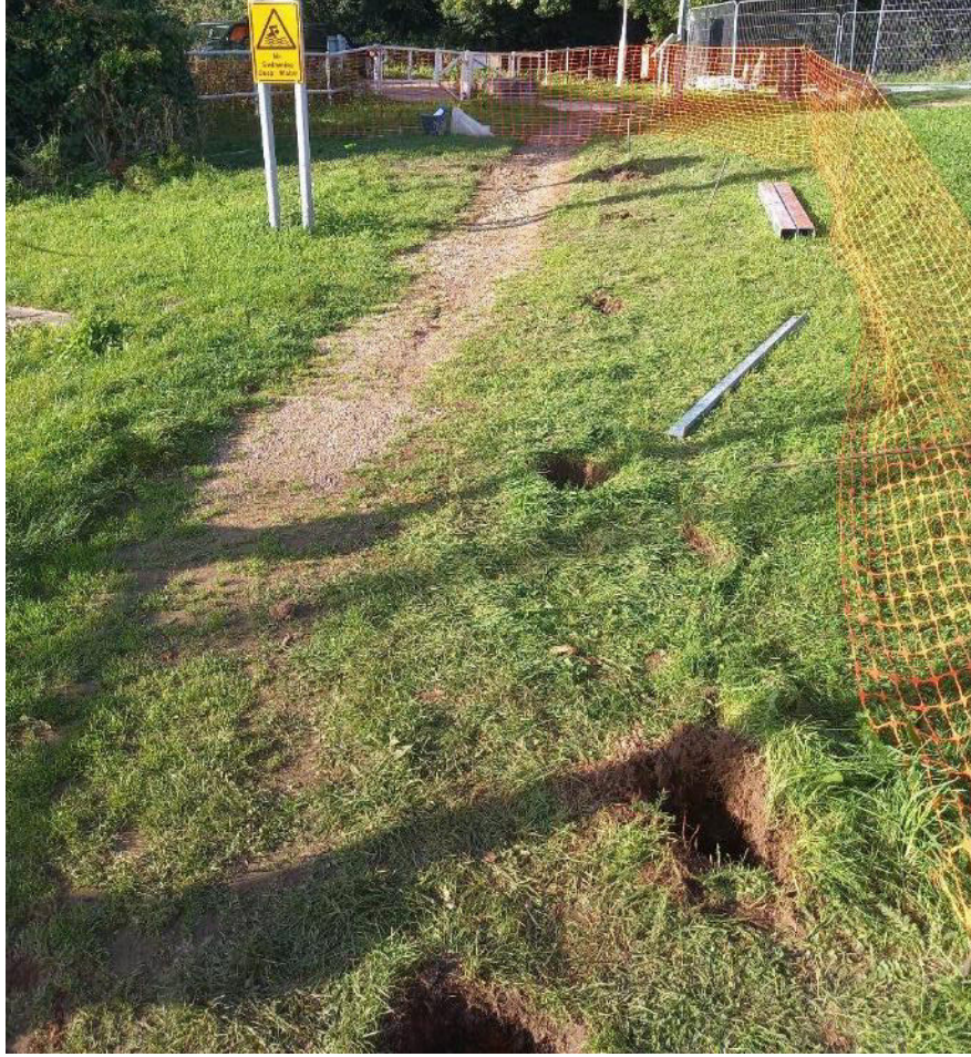
Plate 13: North facing view of postholes at eastern end of the fence.
