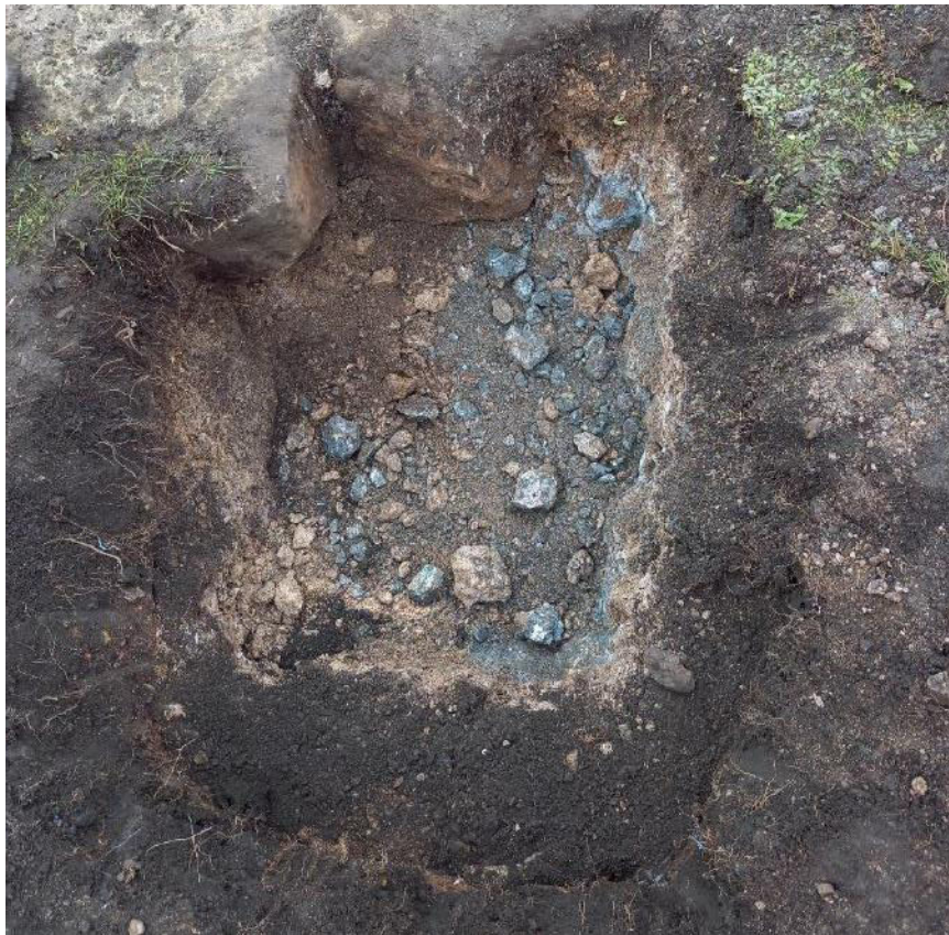
Plate 8: South facing view of Mooring Point 4.
