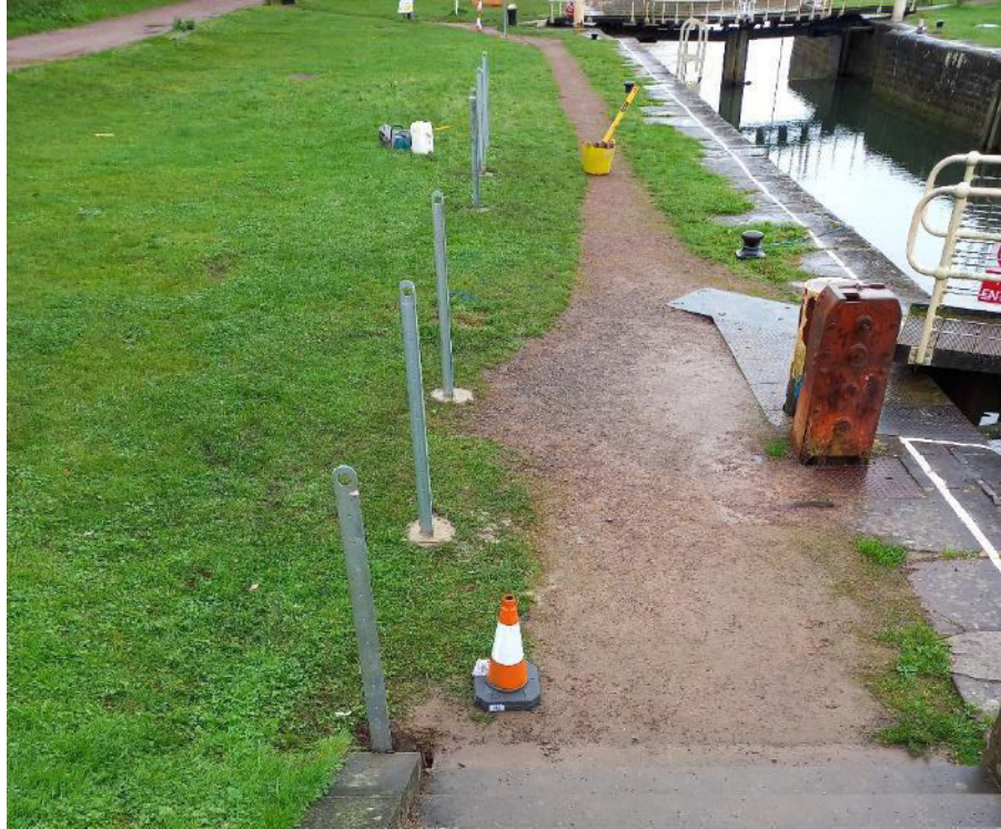
Plate 16: East facing view of central part of the fence line.
