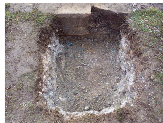
Plate 7: South facing view of Mooring Point 3.
