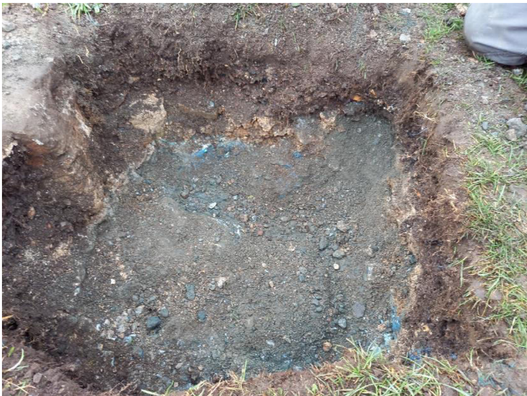
Plate 10: West facing view of Mooring Point 6.
