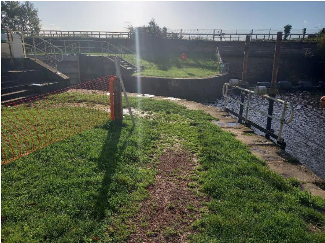
Plate 12: South facing view of proposed fence line.
