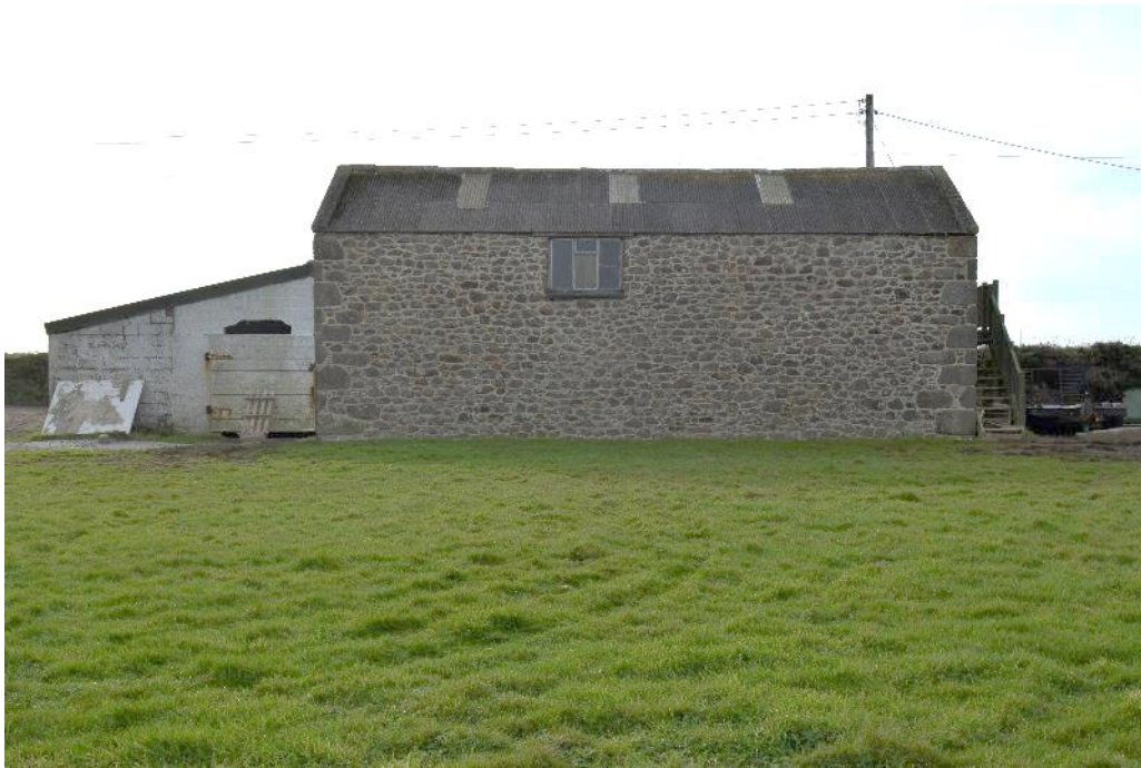
Figure 10: Rear Elevation (Archive ref: BOTA1017_023)
