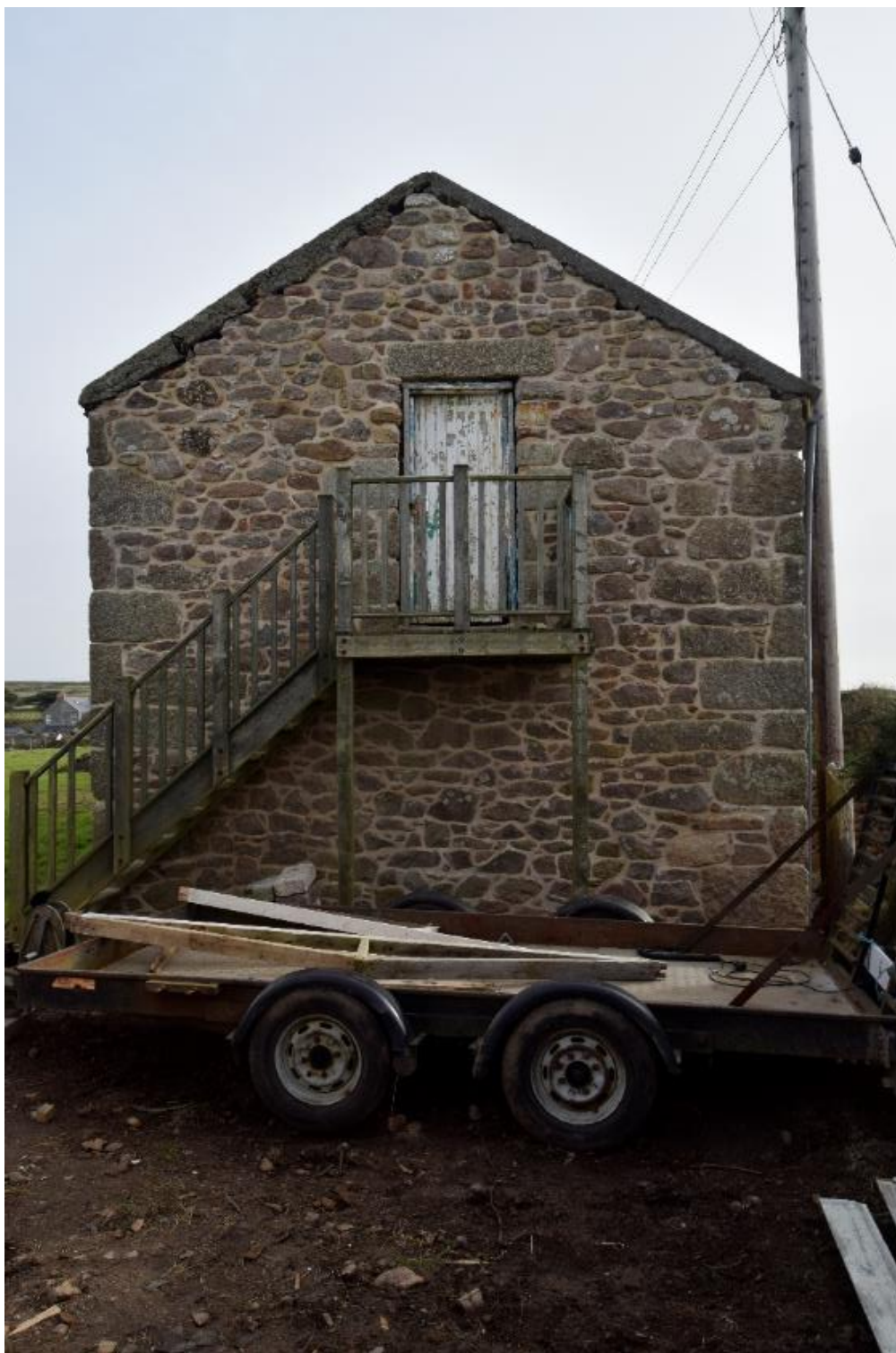
Figure 11: West gable of the building (BOTA1017_0024)
