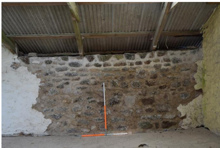
Figure 15: showing the interior of the rebuilt section of the south elevation.
