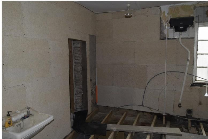
ii) Building 3, Bathroom 2. Showing like for like mortice and tenon jointed carpentry repair.
