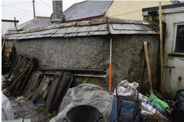
iii) Cob Wall: Cut by Rear Kitchen
