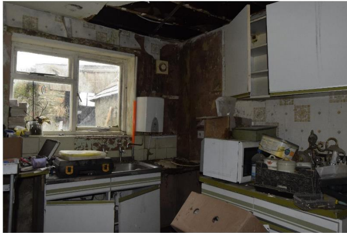
i) Rear Kitchen: Interior facing N
