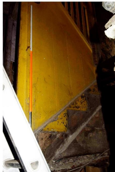
Beyond the door lies a narrow corridor within a rear lean to extension to Building 1 which houses a currently abandoned dog leg service stair case of later 19th century style which runs in two flights. iii) left: a straight flight with winder from first floor to attic storey iv) right: a straight flight from the rear of Building 4 to the first floor.
