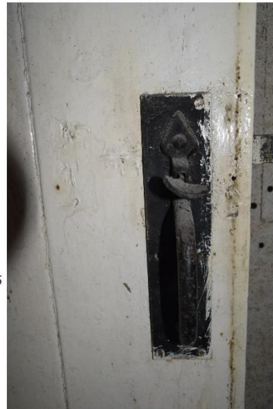
i) Building 1: (left) First floor corridor, access door to attic stairs. ii) (right) this simple plank door can be dated by its hinges and 'norfolk latch' to the later nineteenth century (see Gloucestershire example dated to 1885 in Hall 2005,57).
