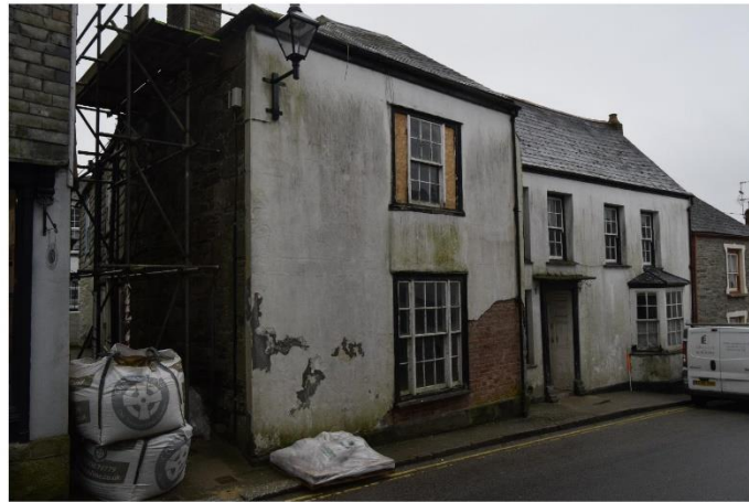
i) Building 1 SE Front Elevaton
