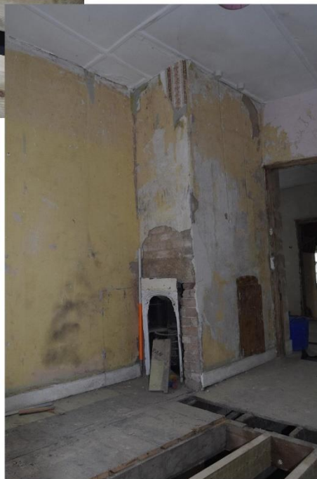
iii) Building 3, Bathroom 2. re-opened hearth in central chimney to be retained with reclaimed fire inset.
