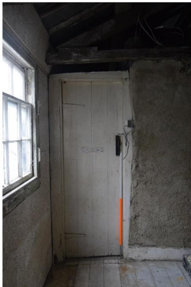
i) Building 1: (left) First floor corridor, access door to attic stairs. ii) (right) this simple plank door can be dated by its hinges and 'norfolk latch' to the later nineteenth century (see Gloucestershire example dated to 1885 in Hall 2005,57).
