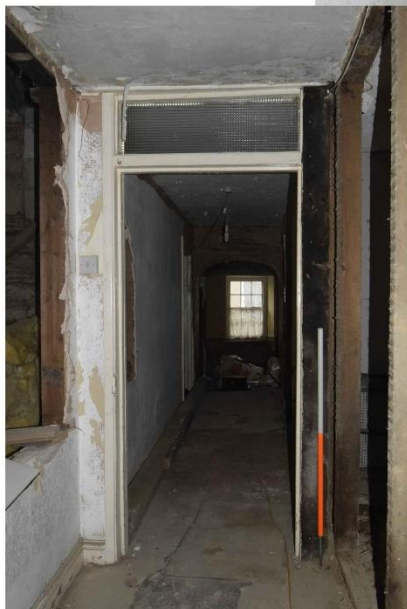
ii) Right: Building 3 rear service passage looking SE, showing mid C20 plasterboard finish to studs / blockwork
