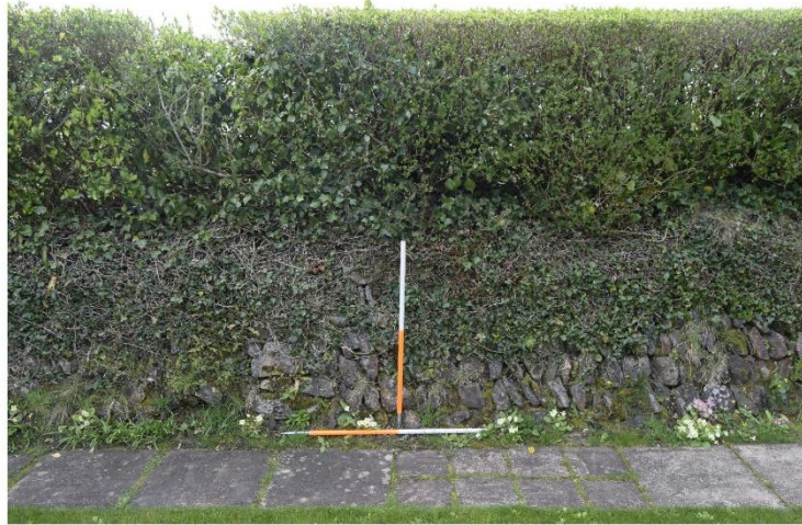
iv) Southern boundary of site (from site). Modern Cornish Hedge with evergreen hedge
