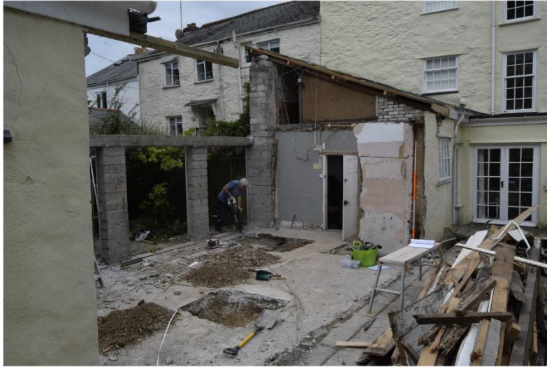
i) Looking south across the site following demolition of modern fabric.
