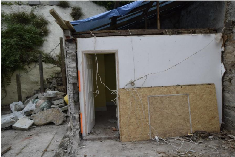
i) Looking north east towards retained wall at edge of site. This wall is a historic timber stud wall faced with blockwork to its south western face.
