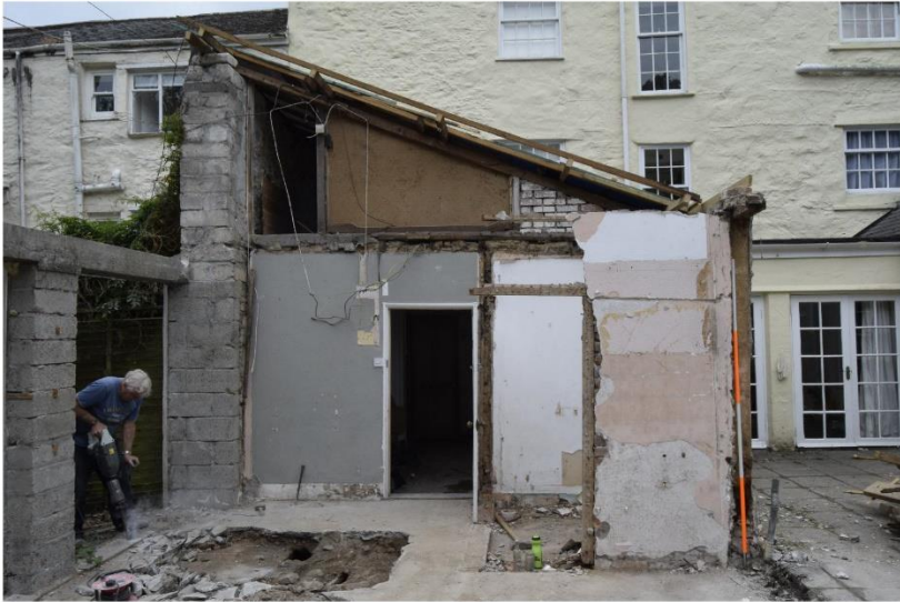
oii)(below) Wall G (nearest camera) is butt-jointed to 'F' and of timber and brick infill construction, faced in modern plaster.
