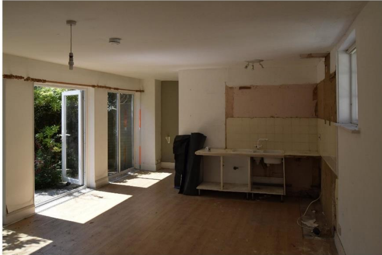
i) Looking SW across the main space consented for demolition.
