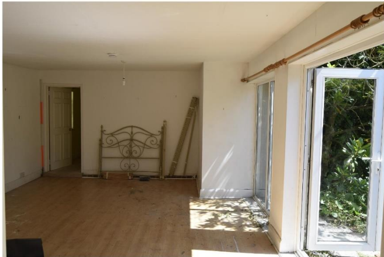
ii) Looking NE across the main space consented for demolition
