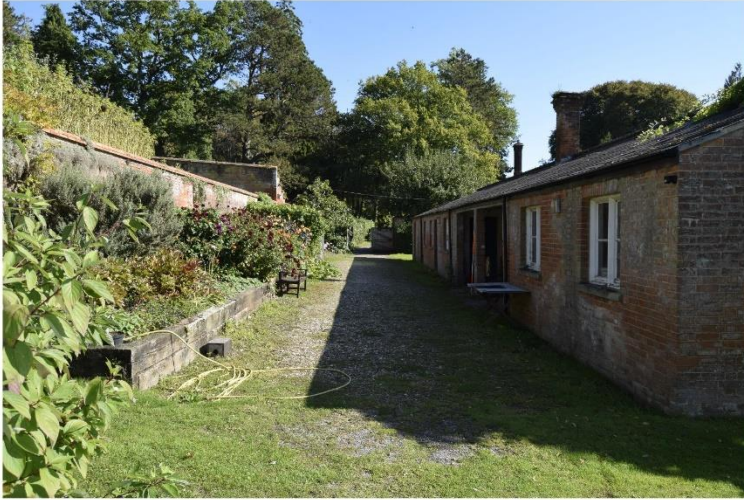
i) Enclosure D - eastern side. Offices
