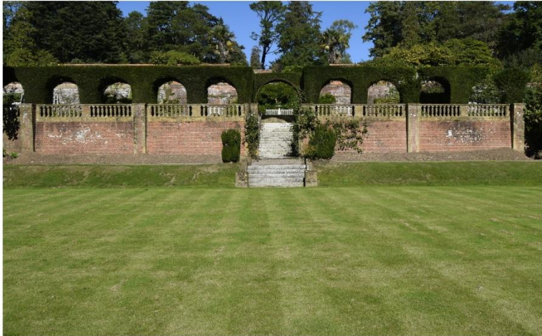
i) Enclosure A from the lawn below showing the steps establishing the central axis of the complex. Note that the upper terraces are not visible from outside the garden.
