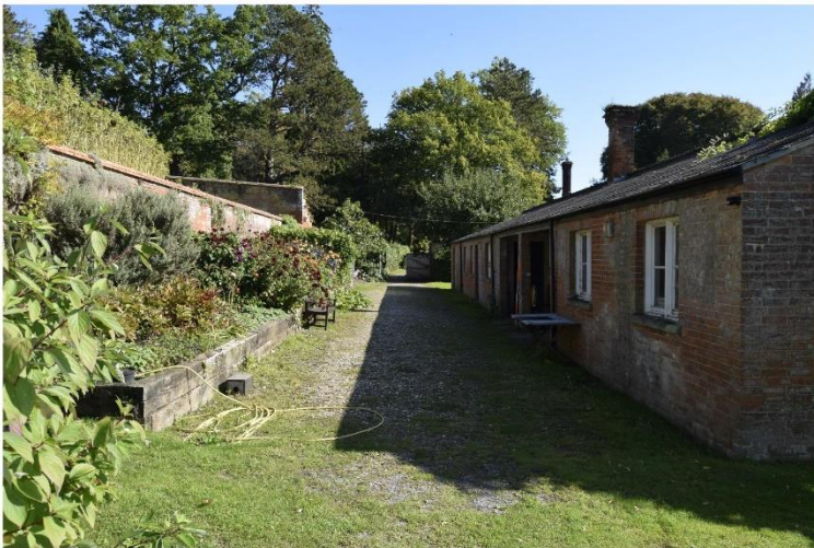
ii) Enclosure D Western Side - Bothies and cold frame
