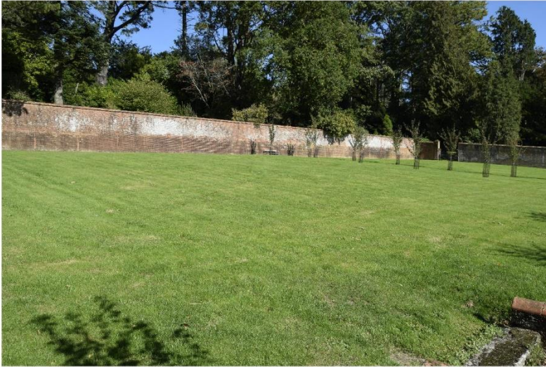
i) Looking NE across enclosure F. The proposal would introduce two single storey cabins set closely parallel to the wall to rear. Note widened entrance in east wall.
