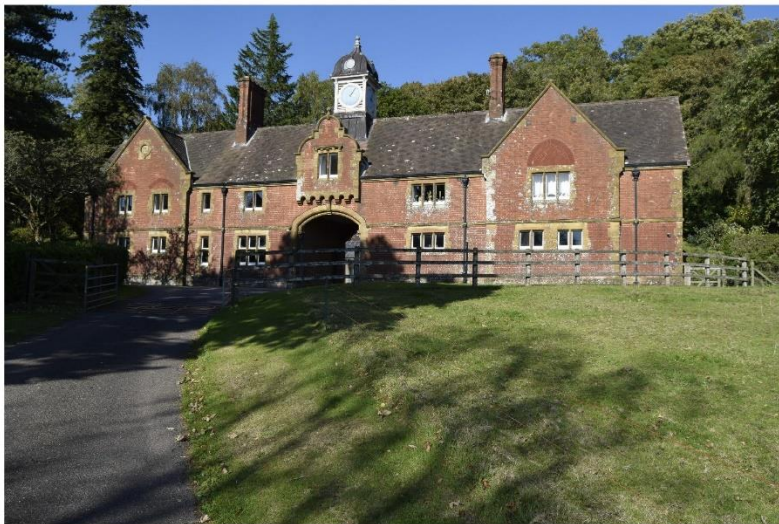
ii) Sidbury Manor Stables, South Front
