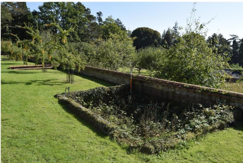
iii) Water tank set against southern wall of Enclosure F
