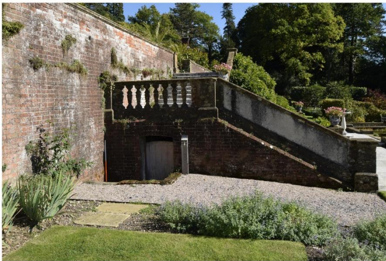
ii) Access to furnace room
