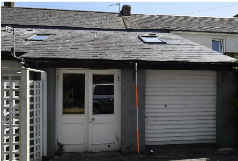
ii) The southern range. Front elevation is timber framed.
