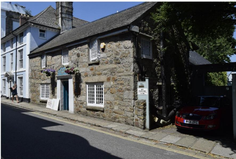
ii) 52 Chapel Street, elevation to street.
