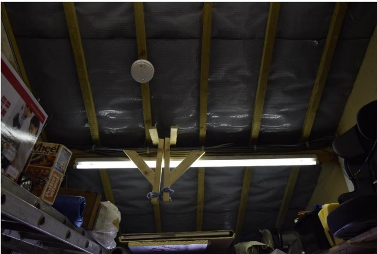
ii) The roof is a modern common rafter structure
