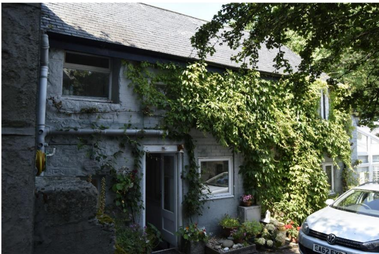
ii) 52a Chapel Street - converted rear ranges of main building.
