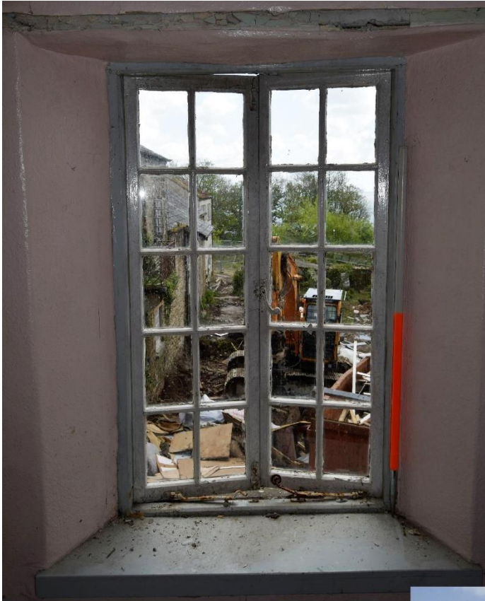
Left - typical pattern of 1930s casements within the stable range (the other side of the window shown on the cover illustration.
