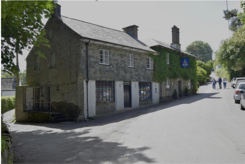
i) Western (principal) and northern (gable) elevation
