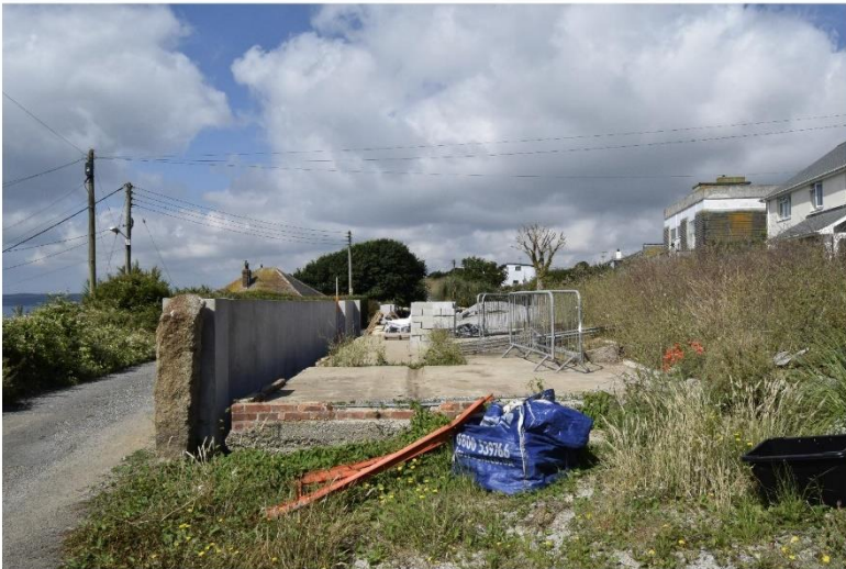
ii) Site from the east
