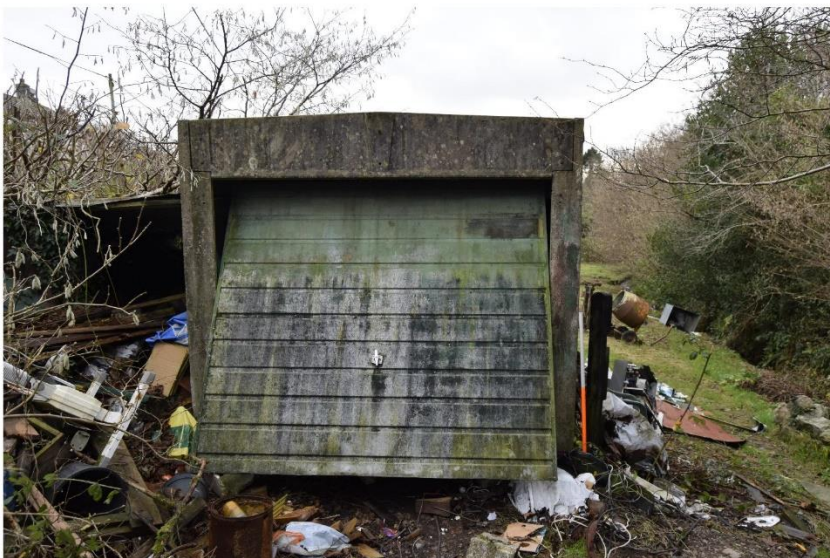
iii) Modern concrete panel garage at north of site
