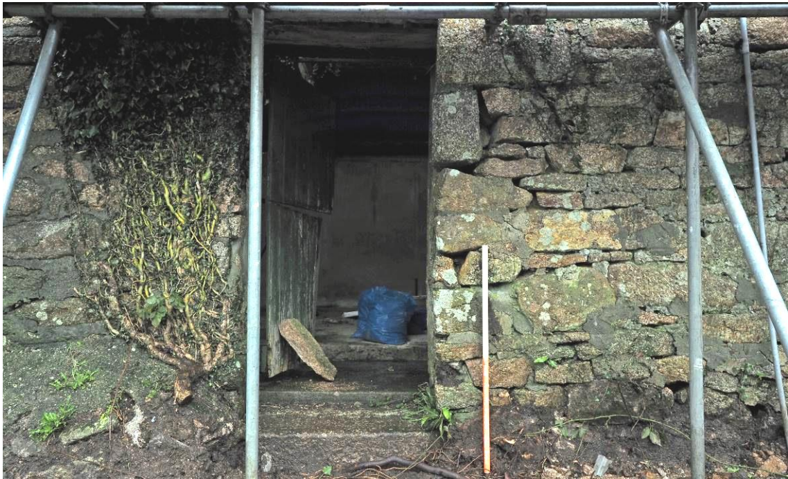
Fig 11: South elevation: Original left-hand window opening remodelled as doorway
