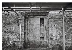
Frame 23: East doorway
