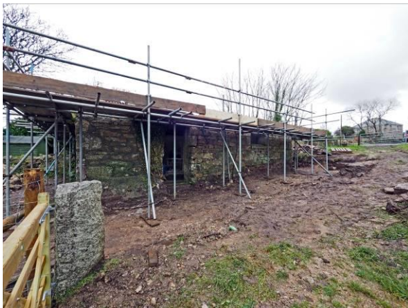
Fig 22: Building from SW + BC chapel beyond
