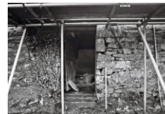
Frame 19: S doorway
