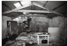
Frame 3: From east
