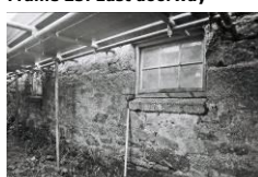
Frame 28: North wall from NW
