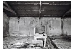
Frame 9: From south
