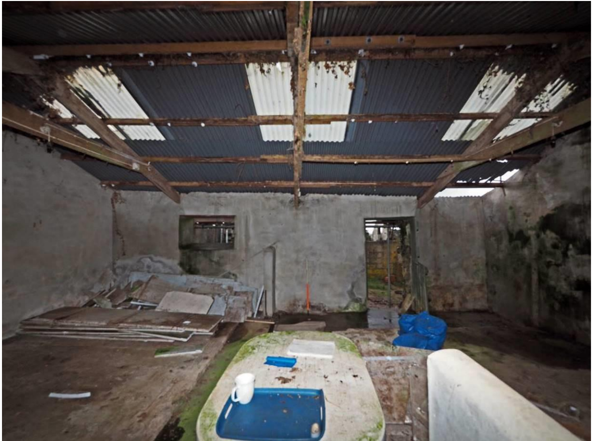
Fig 24: Interior from north
