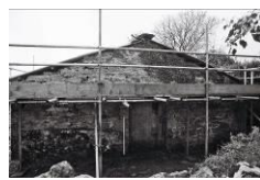
Frame 22: From east
