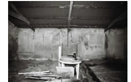
Frame 10: From south
