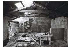
Frame 4: From east
