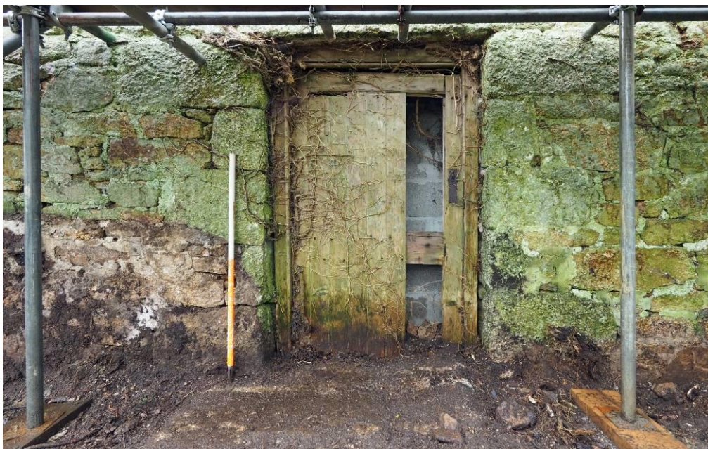
Fig 15: East elevation: Blocked original doorway
