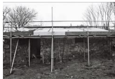
Frame 18: From south
