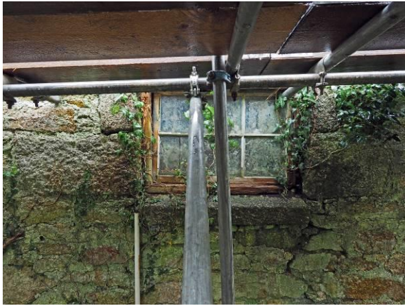
Fig 18: Rear original left-hand window opening
