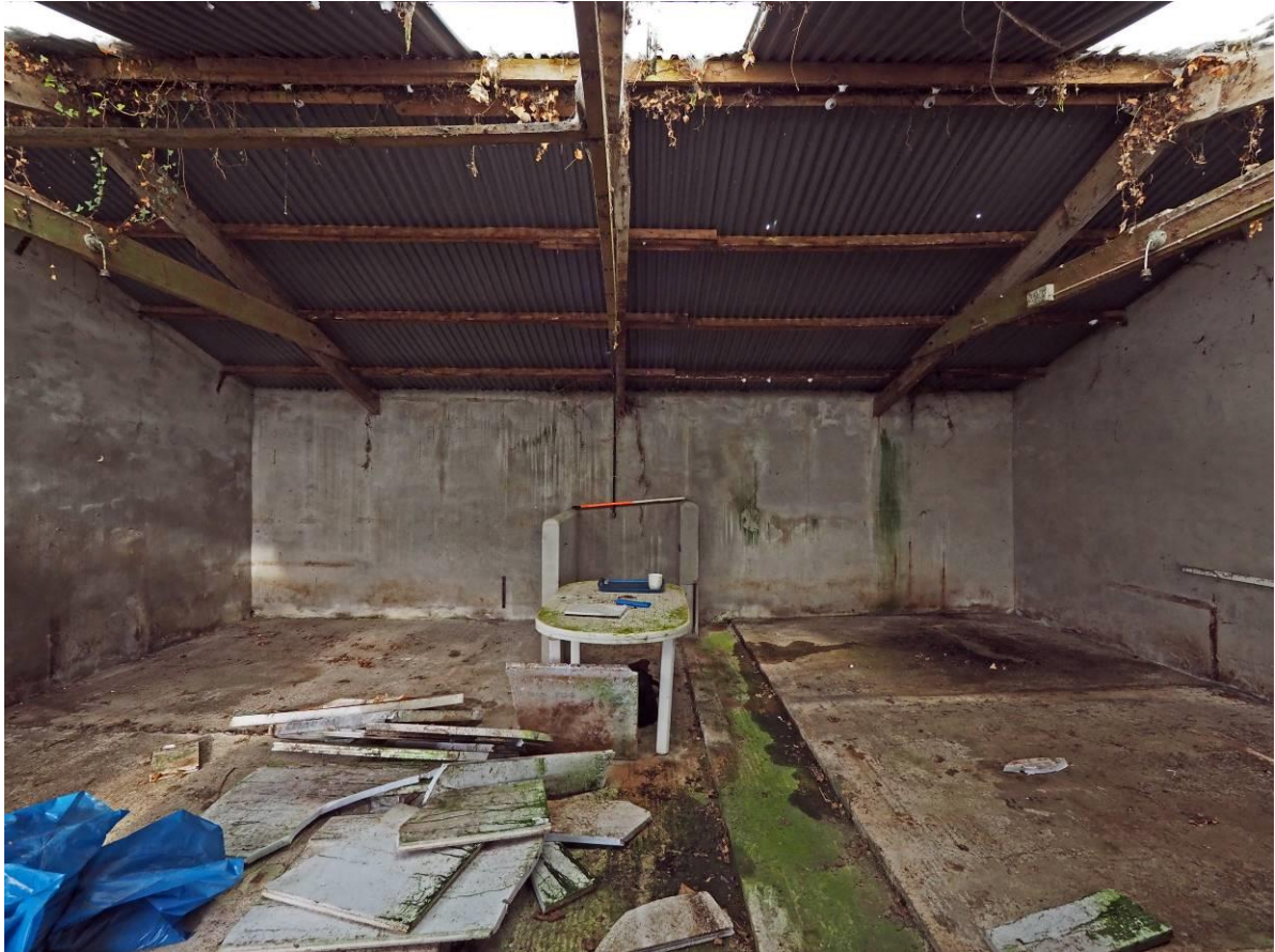
Fig 26: Interior from south
