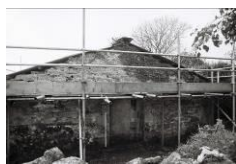
Frame 21: From east
