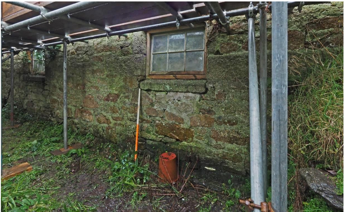
Fig 17: Rear elevation from NW
