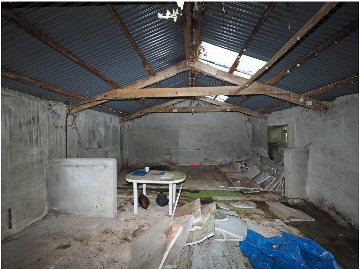
Fig 27: Interior from west
