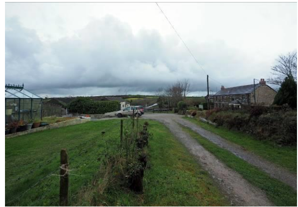
Fig 31: Farmstead from east
