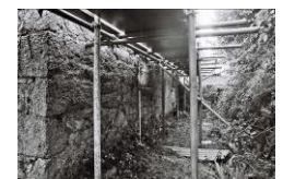
Frame 25: North wall from NE
