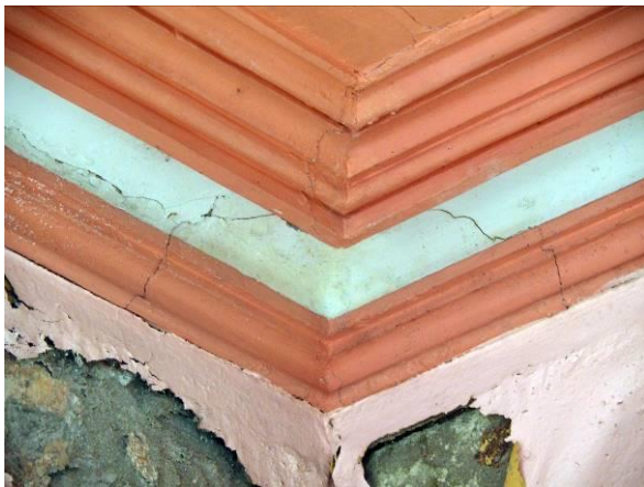
Fig 40: Ceiling cornice to SW corner
