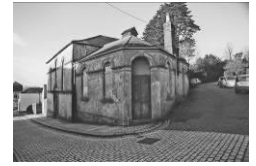
Frame 5: Former BC from NE
