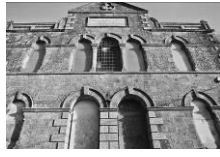
Frame 2: From south
