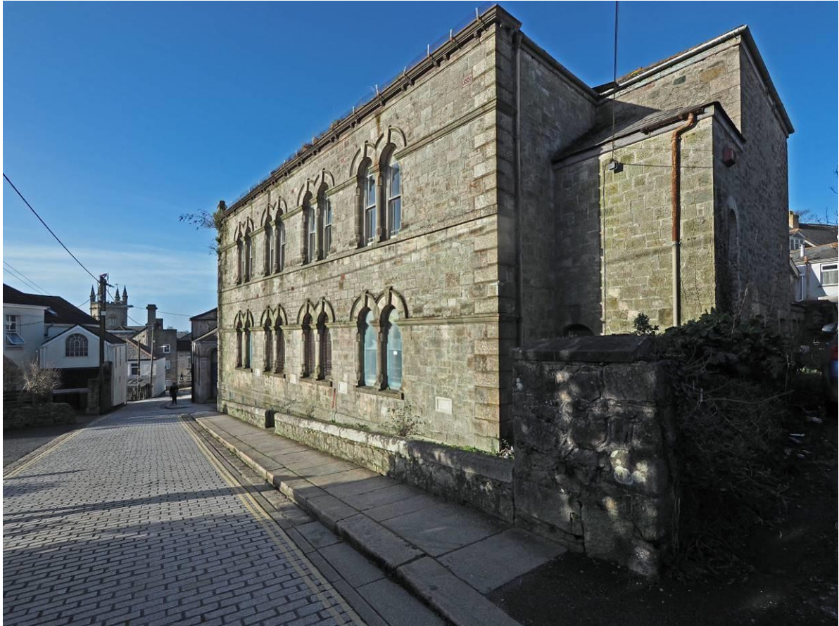
Fig 15: Subject building from NNE
