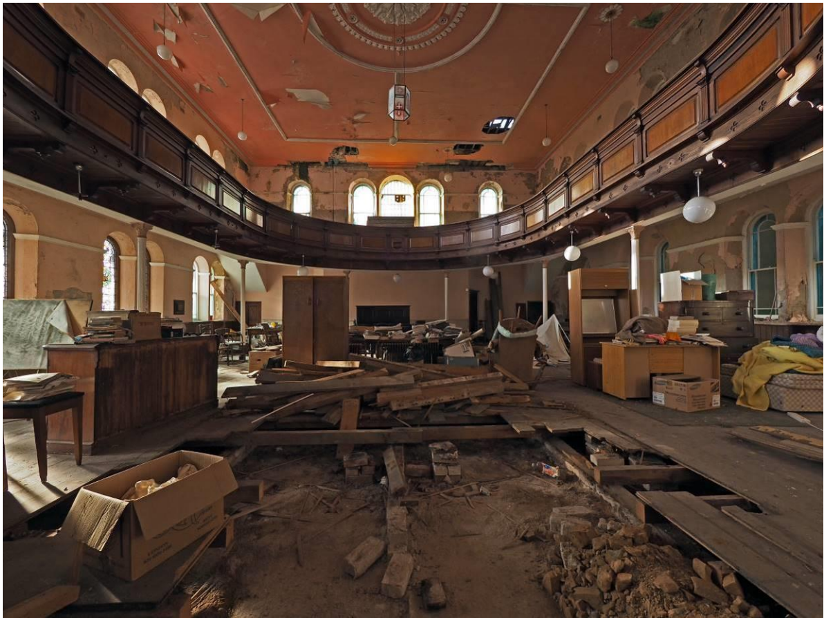
Fig 17: Interior from north
