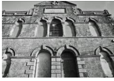
Frame 1: From south
