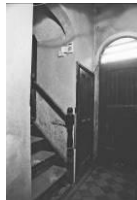
Frame 33: NE stair hall
