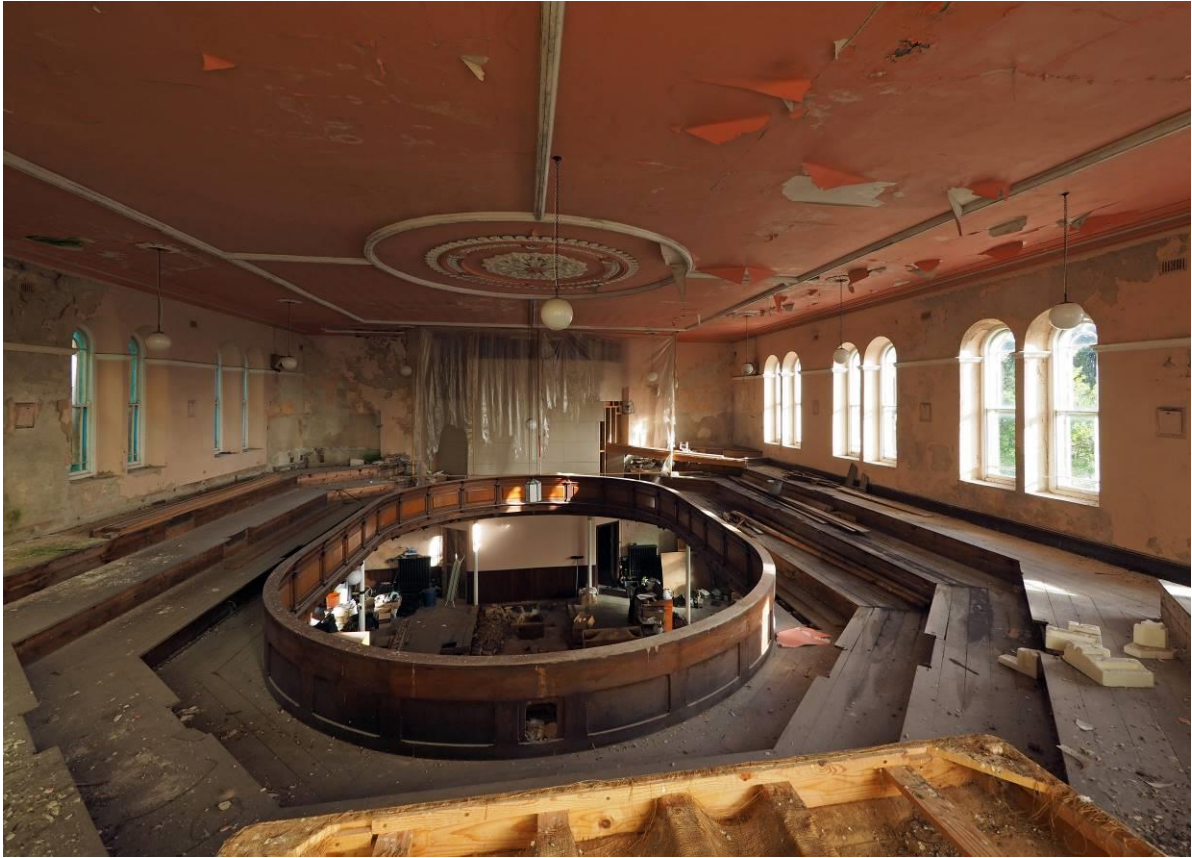
Fig 21: Gallery from south
