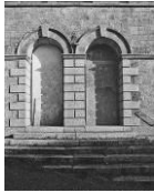
Frame 11: From south
