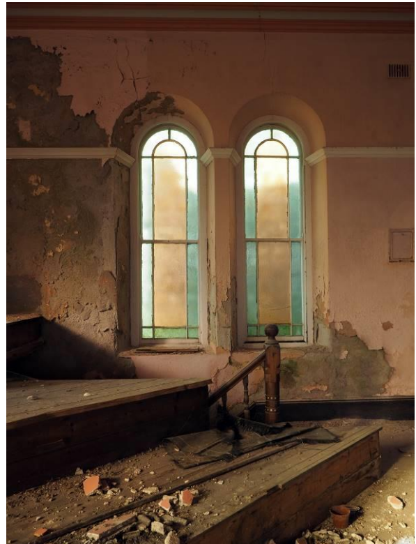
Fig 33: west wall by SW corner
