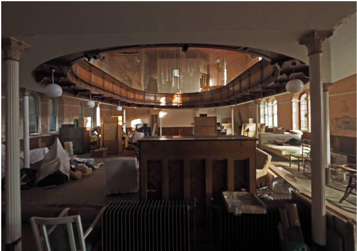
Fig 18: Interior from south
