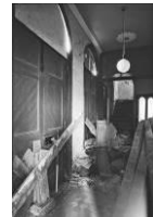
Frame 34: S entrance lobby
