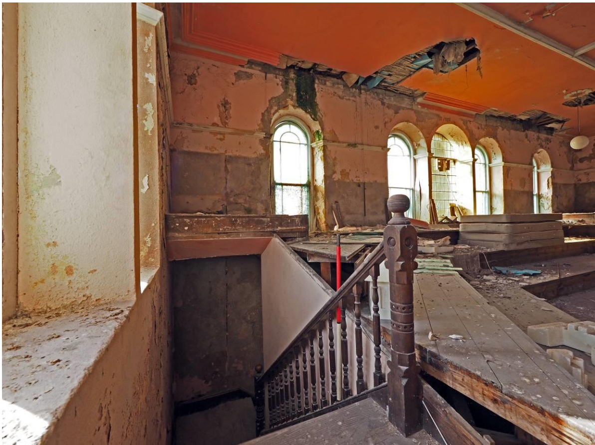
Fig 30: SE stairs from NE
