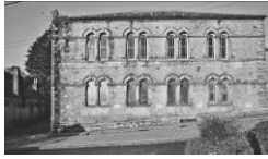
Frame 6: From east
