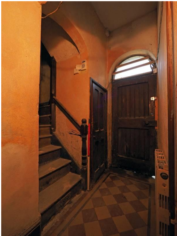
Fig 36: NE entrance hall and stairs
