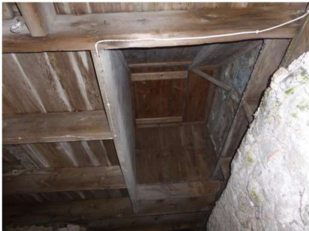
iv) hoist hatch in the floor joists above Space 1
