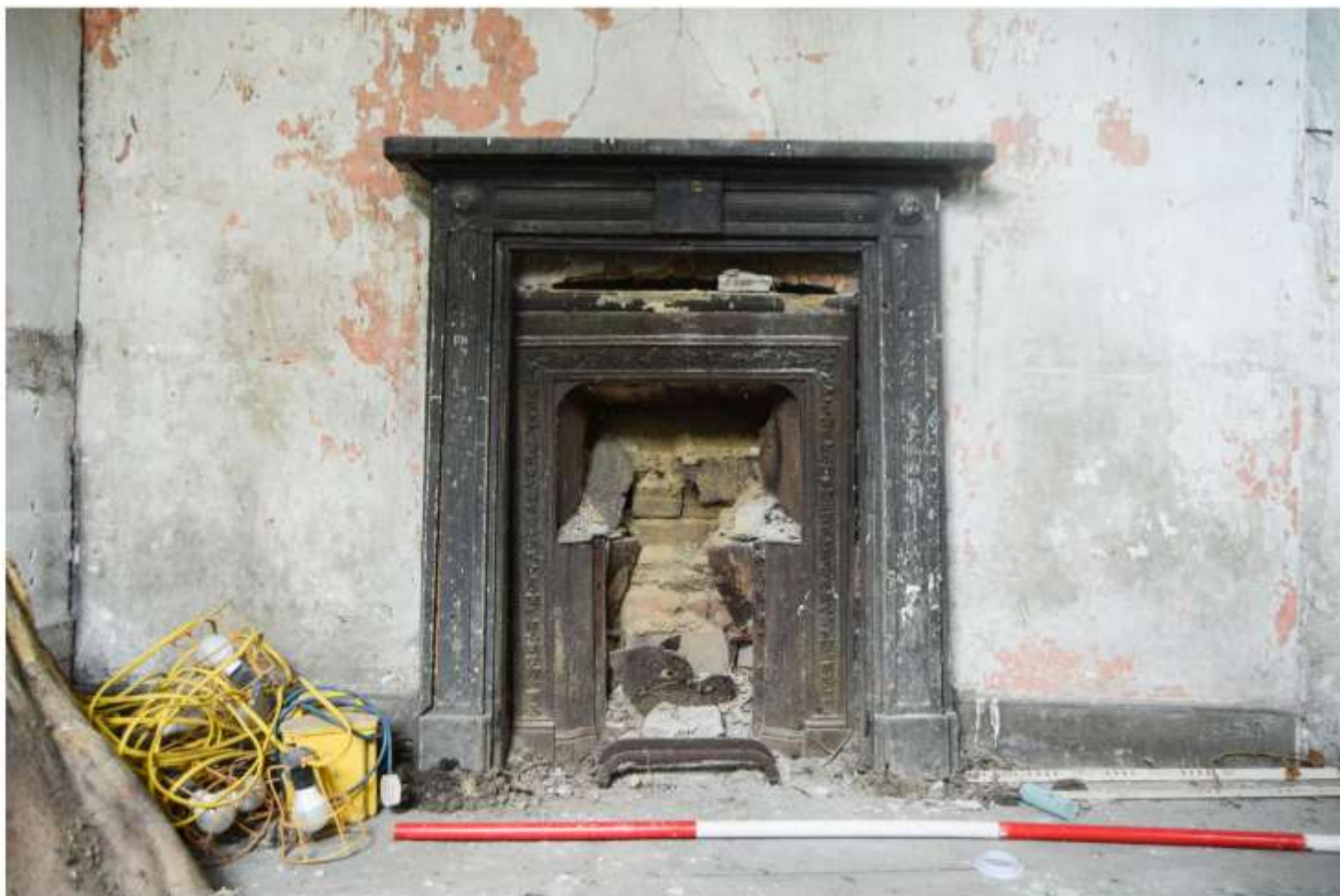
iv) Timber fire surround, Victorian cast iron insert
