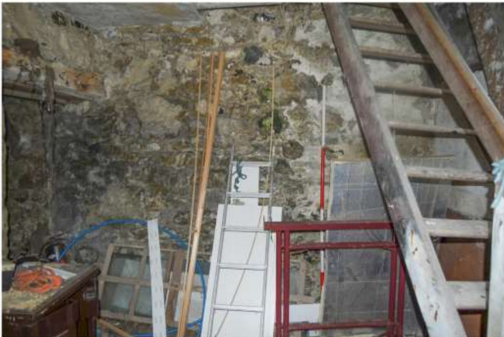
iv) Space 2, south wall
