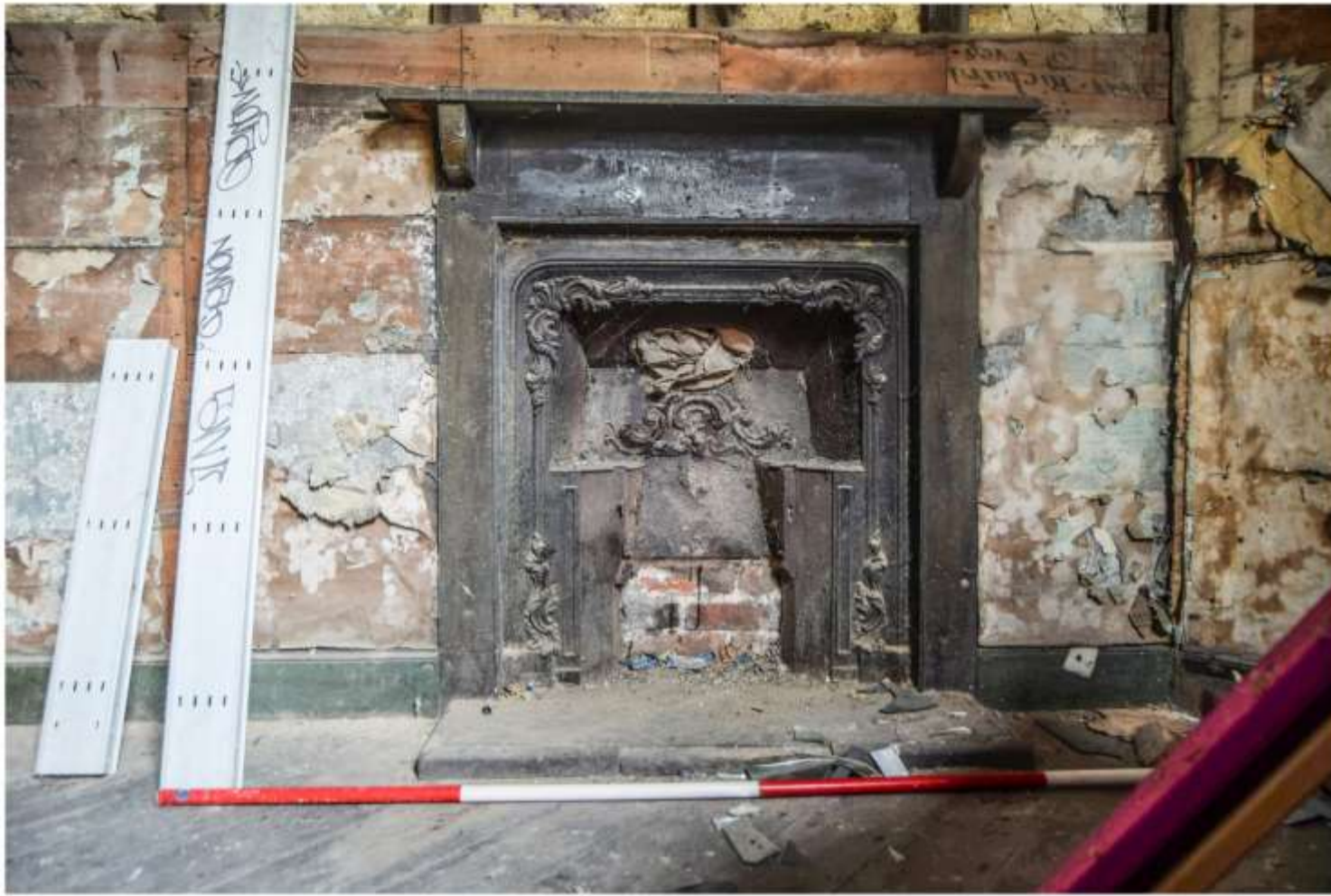
i) Timber fire surround, Victorian cast-iron insert. 2m scale.
