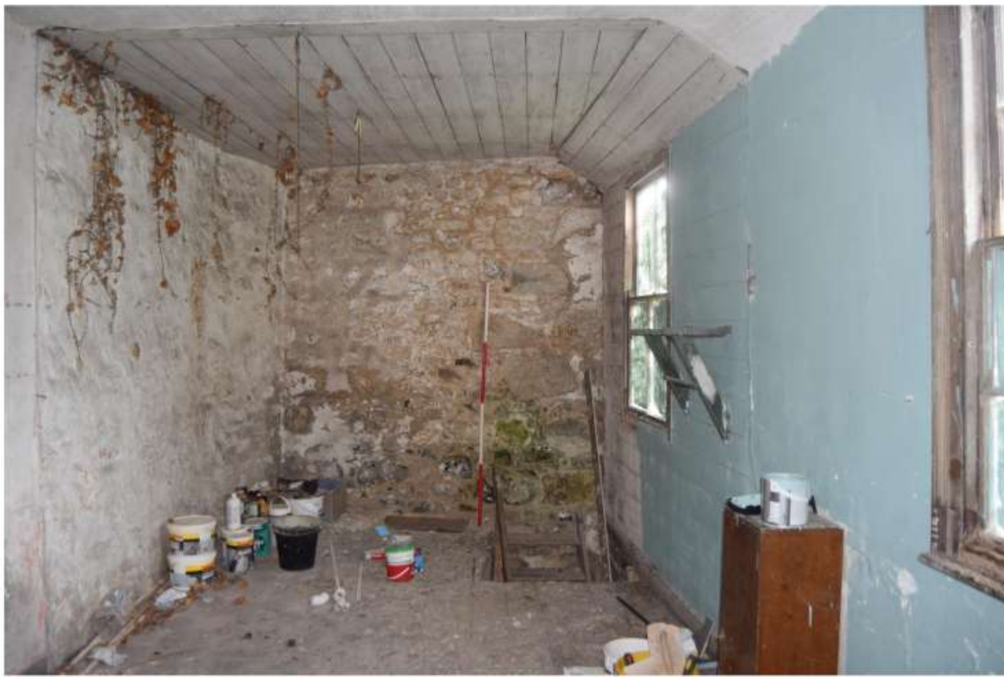
i) room 5 looking west
