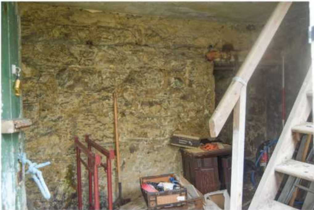
iii) Space 2, south wall
