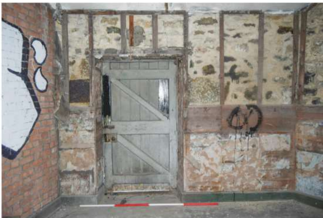
iii) East wall and loading door LLOY1022_0301.jpg 2m scale
