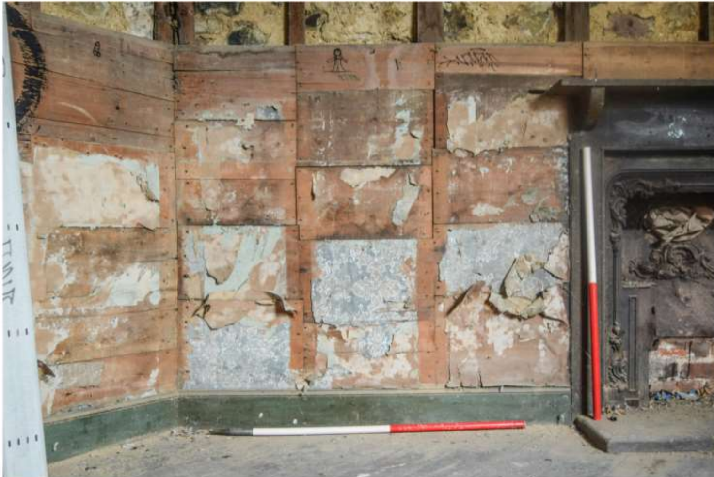
ii) Detail of south wall to left of fireplace. Reused fish-crate timber dry lining and 2 phases of wallpaper
