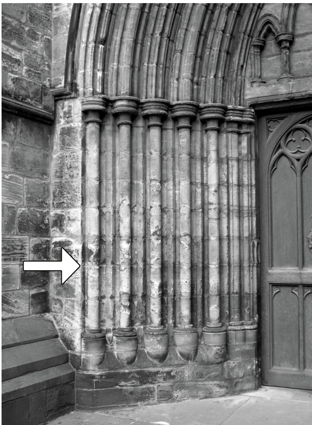
Illus 17 Example of moulded stonework seen in the west doorways of Glasgow Cathedral © Richard Fawcett
