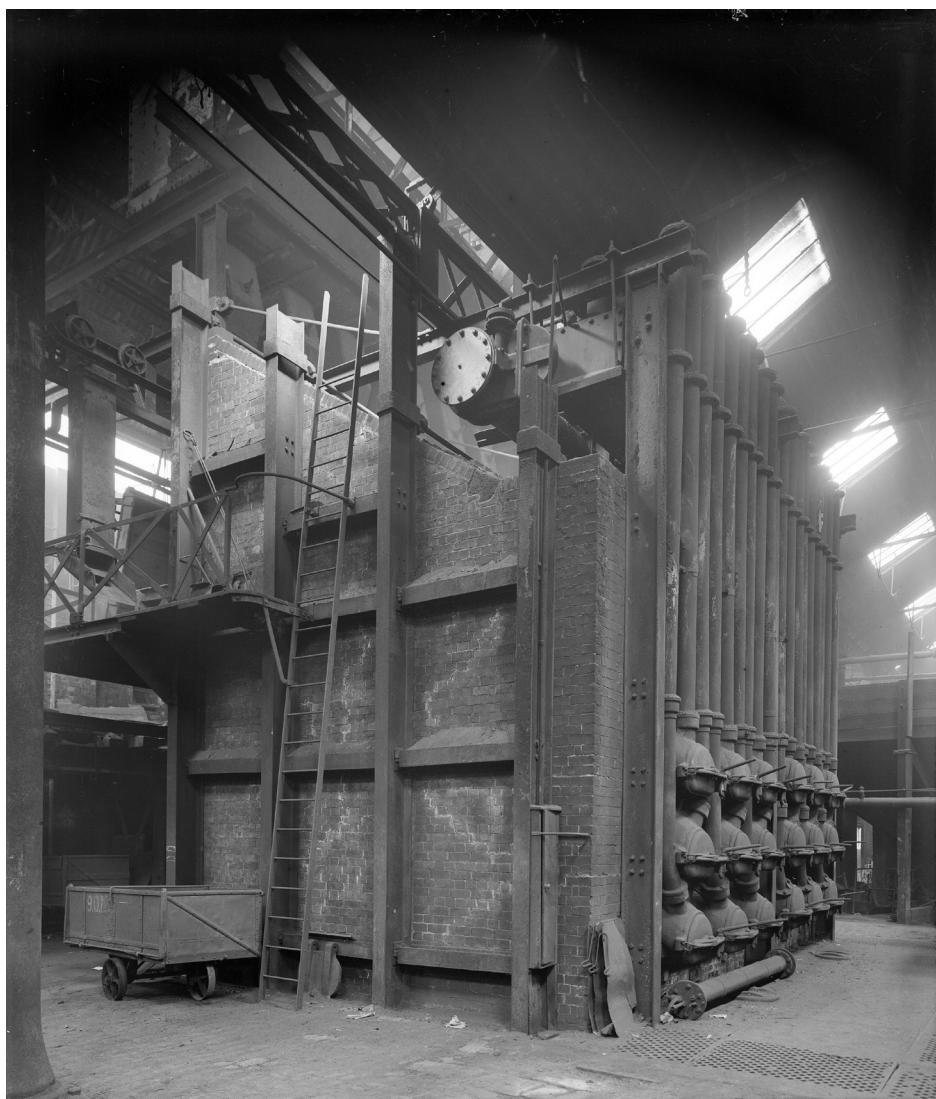
Illus 10 New Street Gasworks retort bench prior to demolition (© HES)
