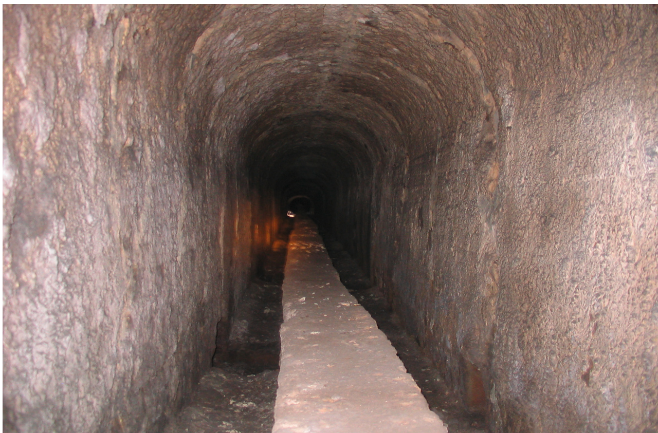
Illus 66 View through the central flue running through the retort benches
