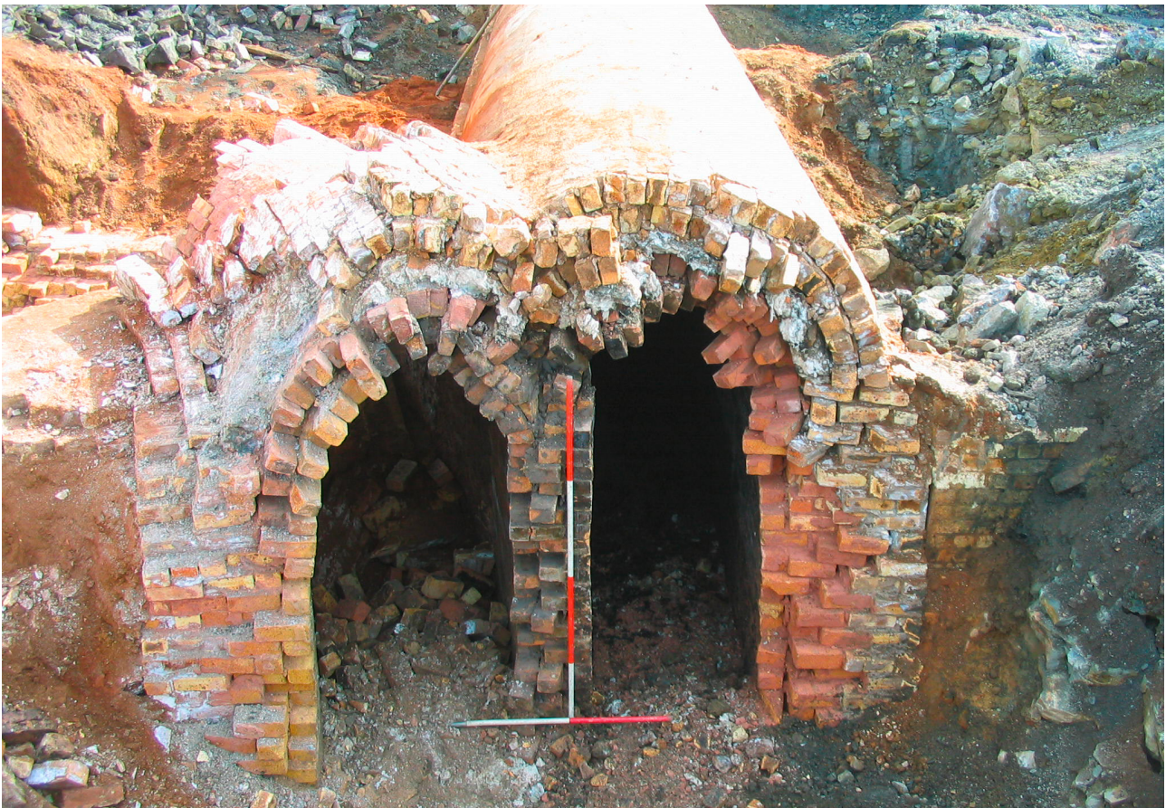
Illus 73 Section through flues (J0312) and (J0313) as they join from the north
