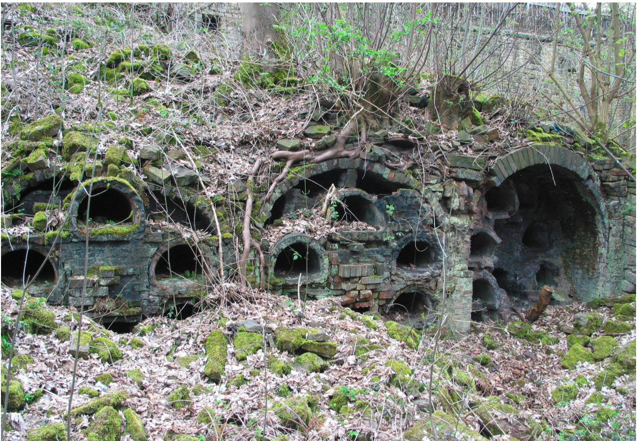
Illus 87 Ceramic retorts at the abandoned gasworks site at Shaw Lodge Mill, Halifax
