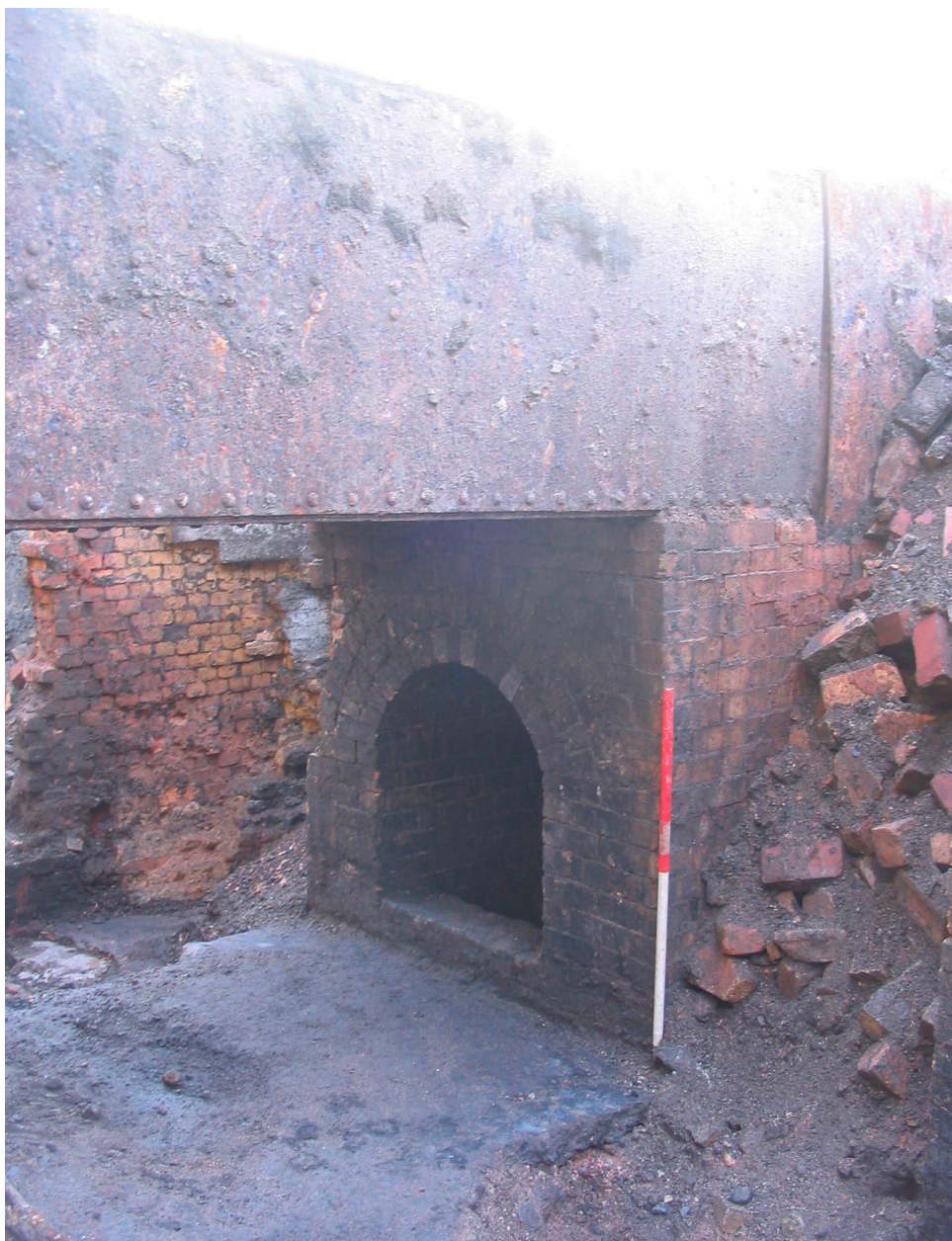
Illus 68 View of the lower flue and support (C0027) from the north-east
