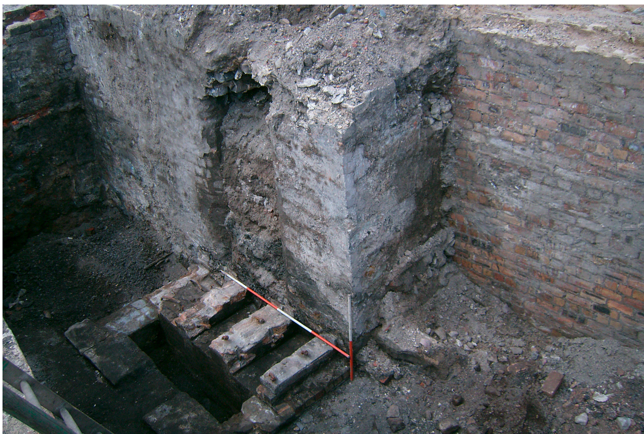
Illus 53 Wall (N0135) from the south-east
