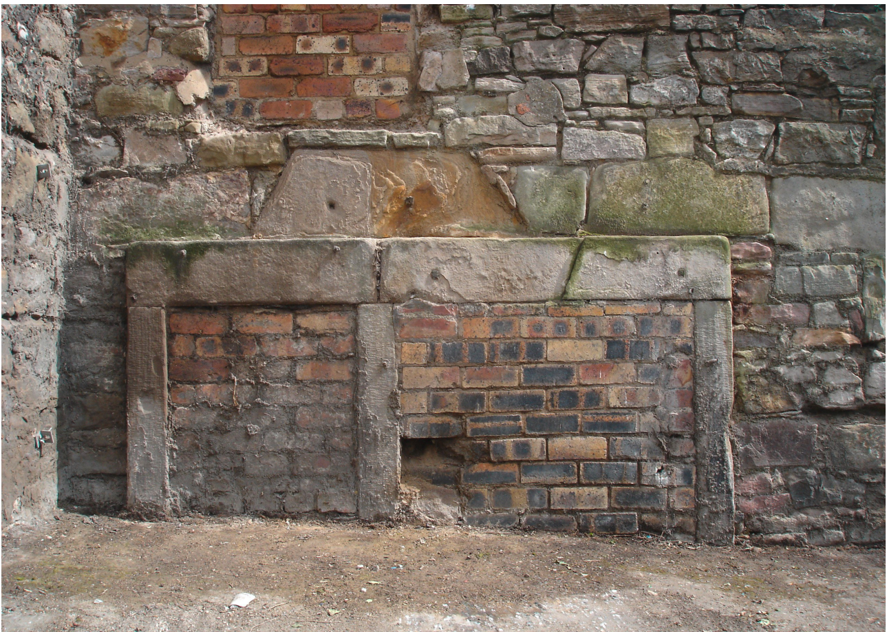
Illus 136 Detail of the range and fireplace, west-facing elevation
