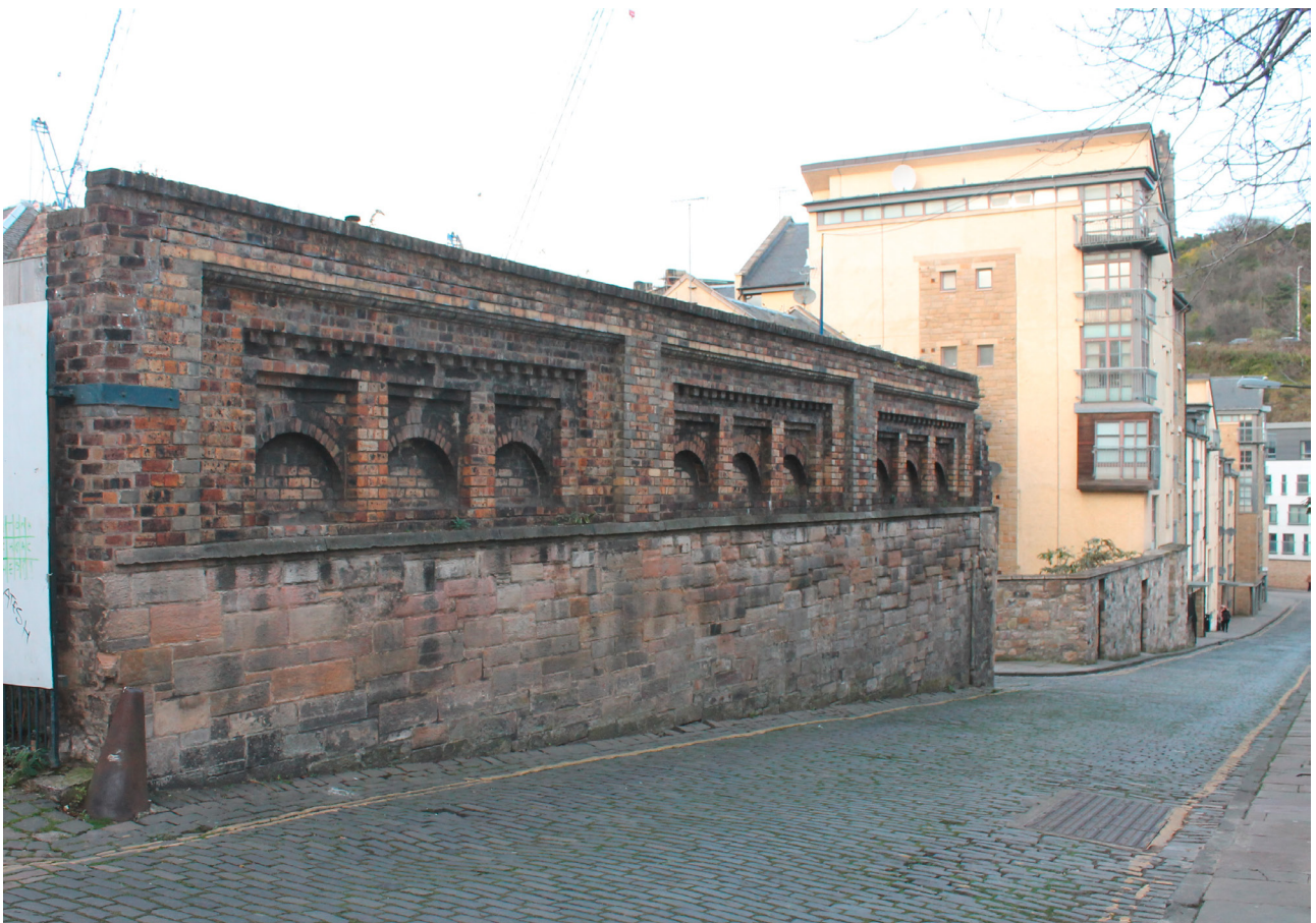
Illus 25 Blind openings in eastern external wall of Gasworks on Tolbooth Wynd
