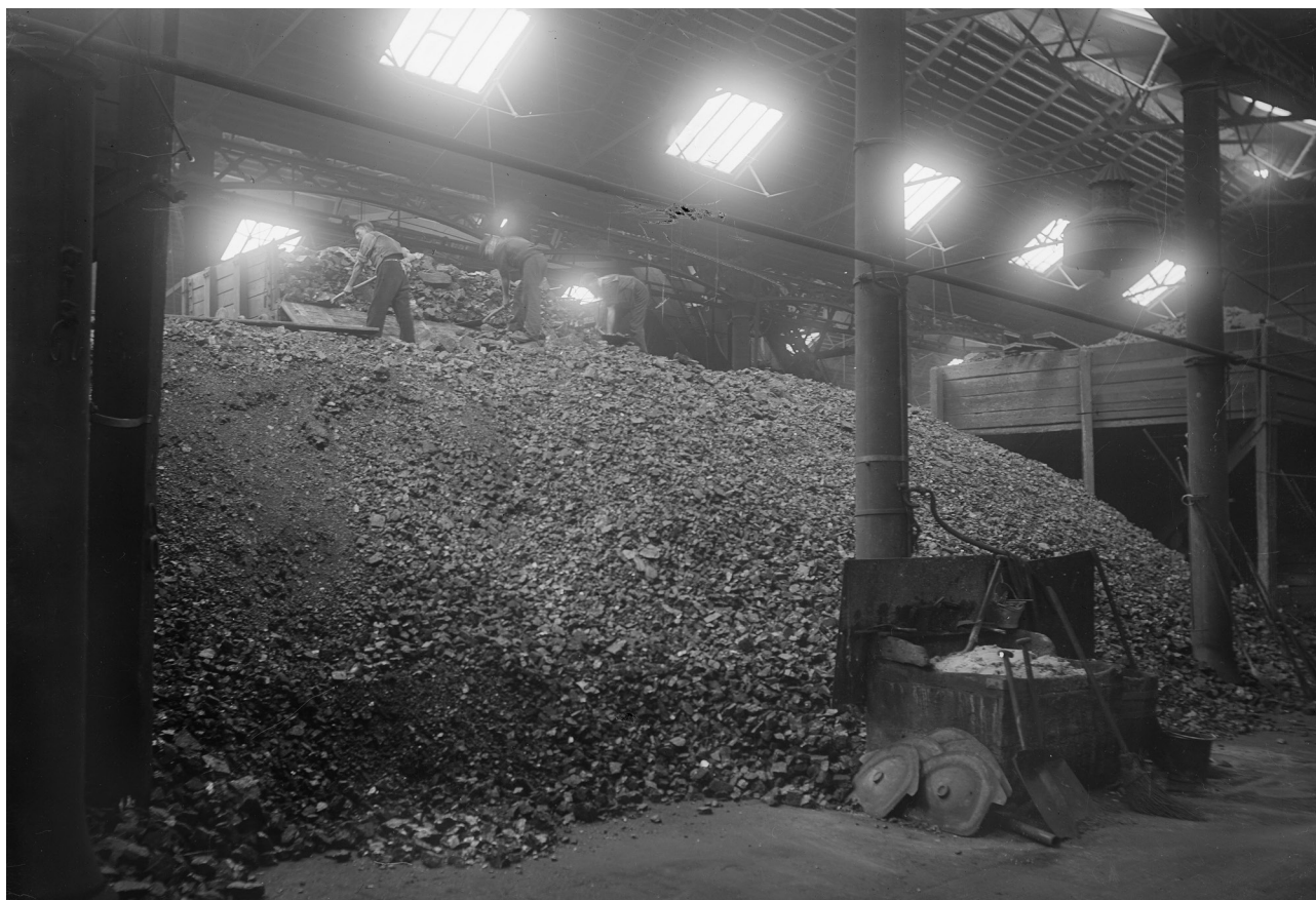
Illus 21 The coal shed in operation prior to demolition (© HES)
