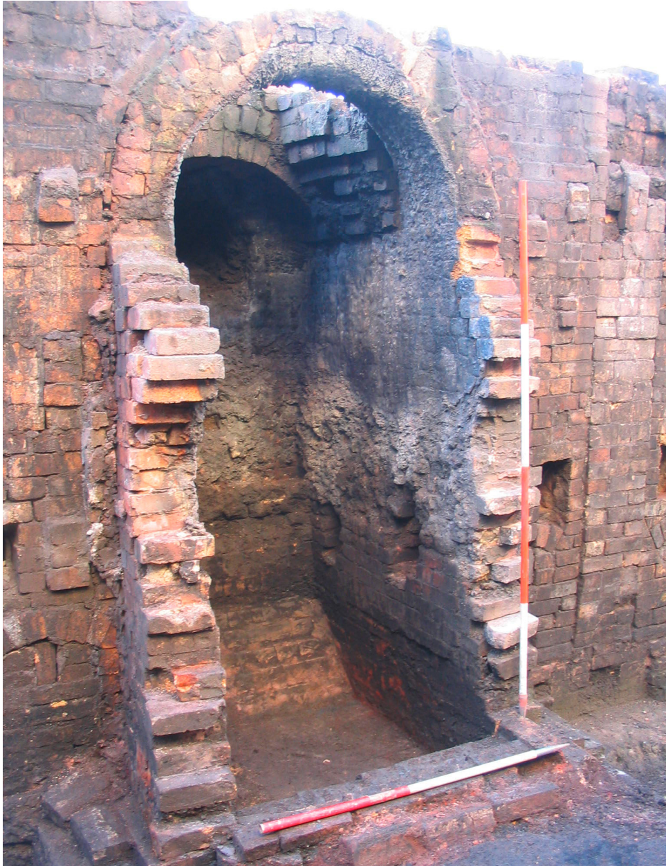
Illus 63 Detail of one of the furnace ovens showing the sloped base
