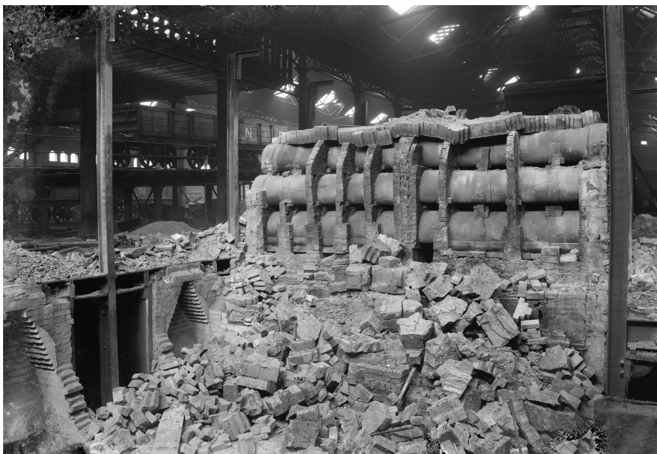
Illus 15 Removal of the horizontal retorts in 1911 (© HES)
