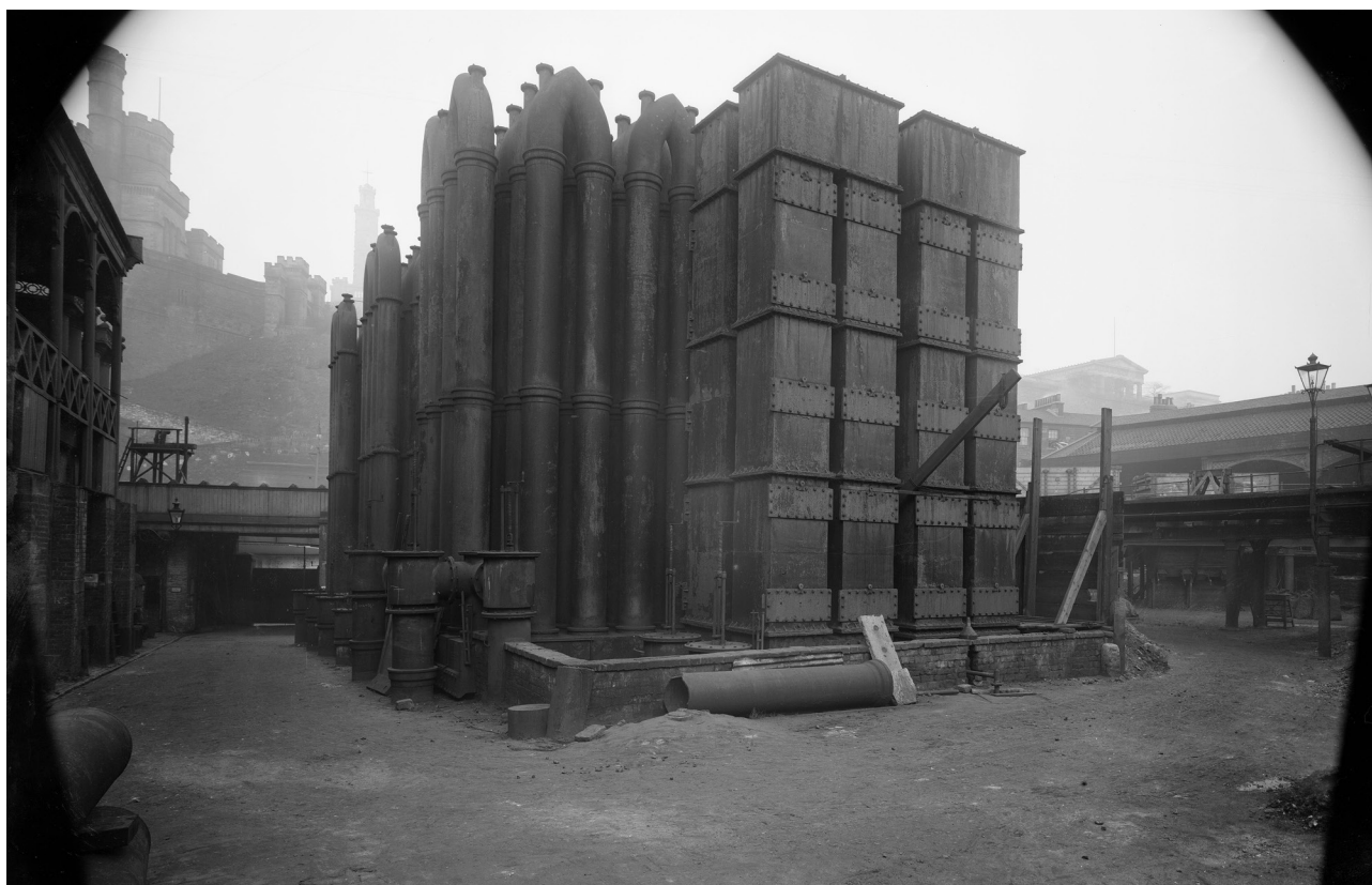
Illus 22 Above-ground piping of the New Street condensers prior to demolition (© HES)
