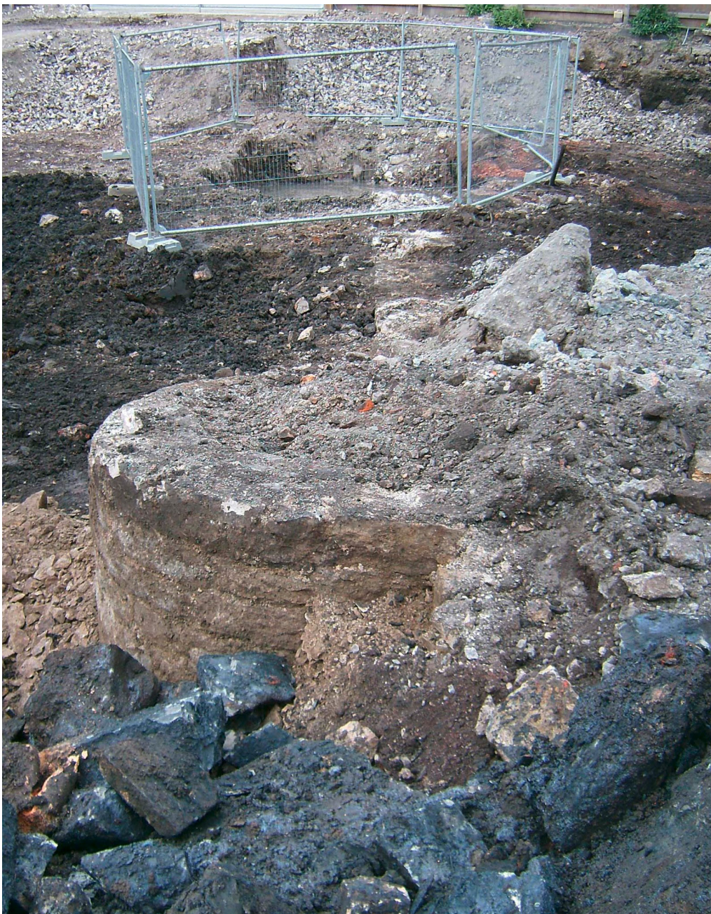
Illus 39 Detail of stone buttress (R046), taken from the south
