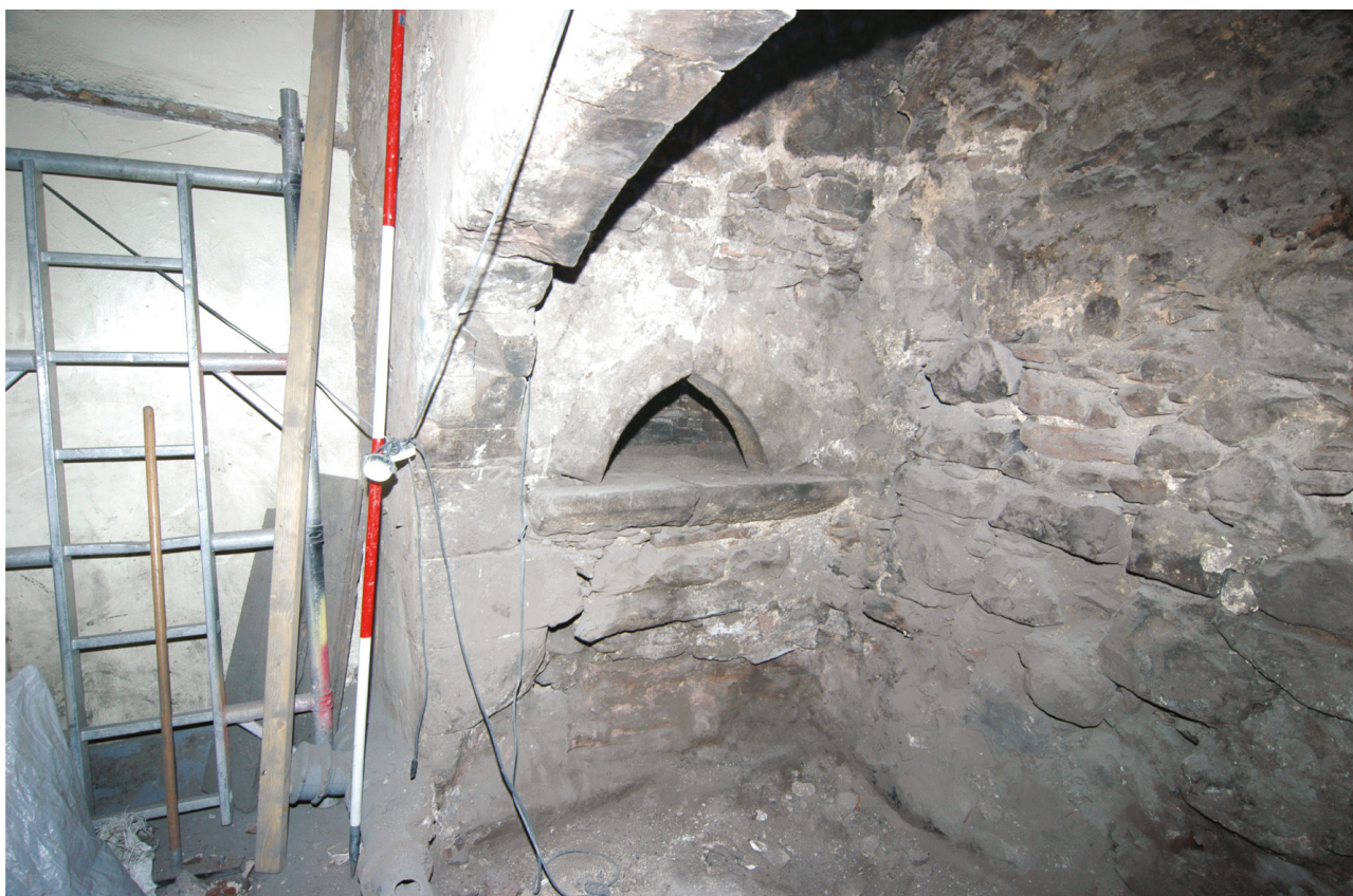
Illus 33 The flue-less bread oven within the interior of the G12 fireplace. (© CFA Archaeology Ltd)
