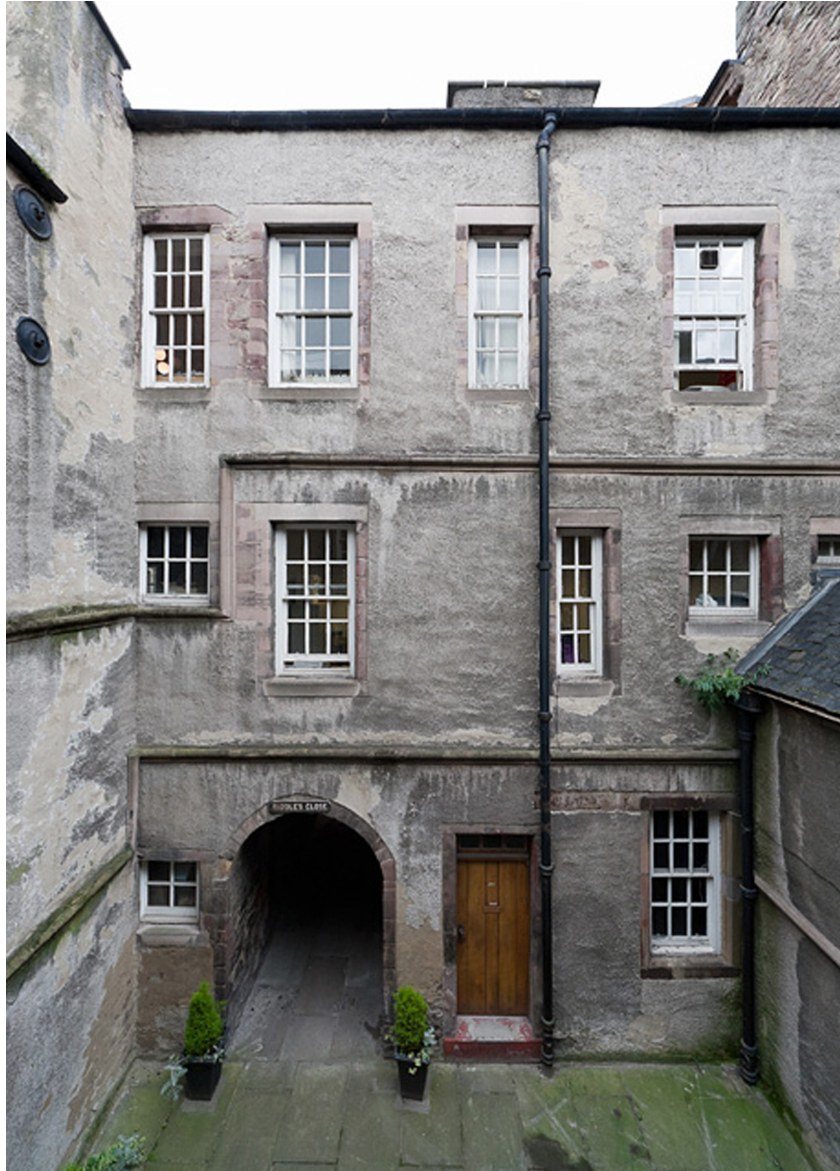
Illus 20 Courtyard, south-facing elevation. (© Scottish Historic Buildings Trust)
