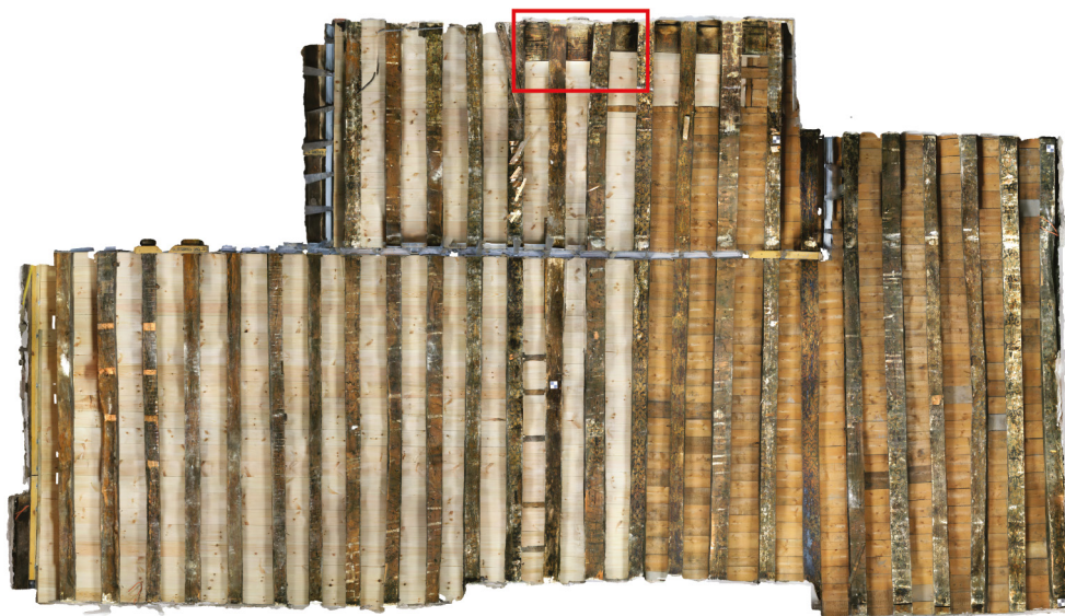
Illus 40 A colour orthophotograph of the painted beam and board ceiling in Room F03, North Block. Inset: the only surviving painted board on the ceiling of Room F03. (© CFA Archaeology Ltd)
