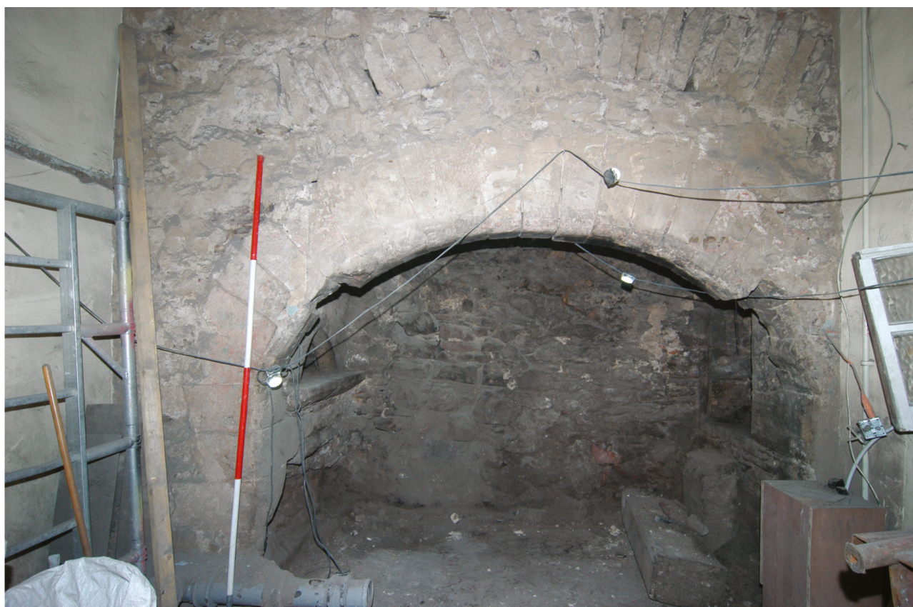
Illus 32 The G12 fireplace after the removal of the later insertions. (© CFA Archaeology Ltd)
