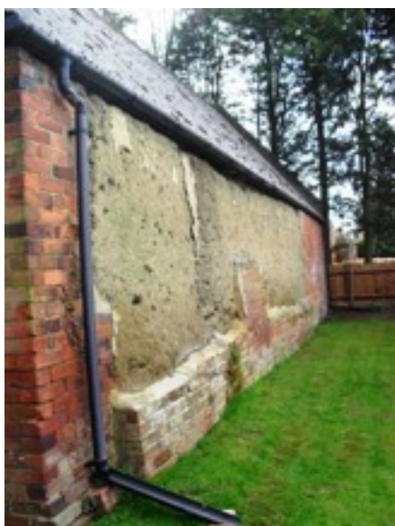
Fig.14 External mud wall of barn
