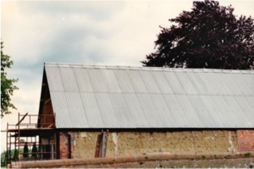
Fig. 21. The 1992 repair work nearing completion
