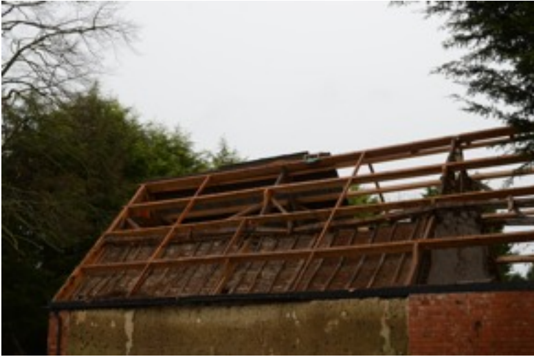
Fig. 22 Demolition of the barn for development December 2015.
