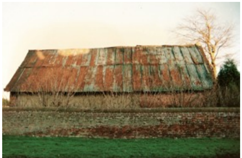
Fig. 17 From the road showing the corrugated iron roof and mud wall.
