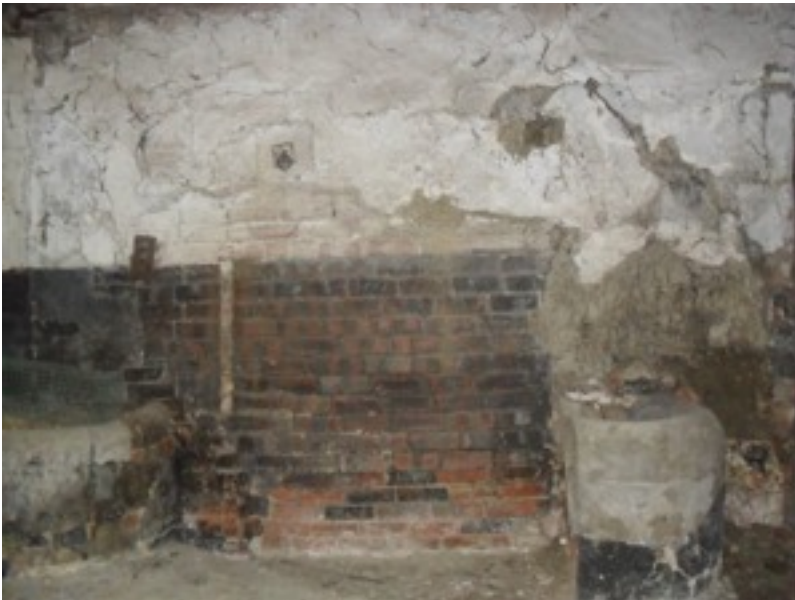
Fig. 21. Barn interior March 2014
