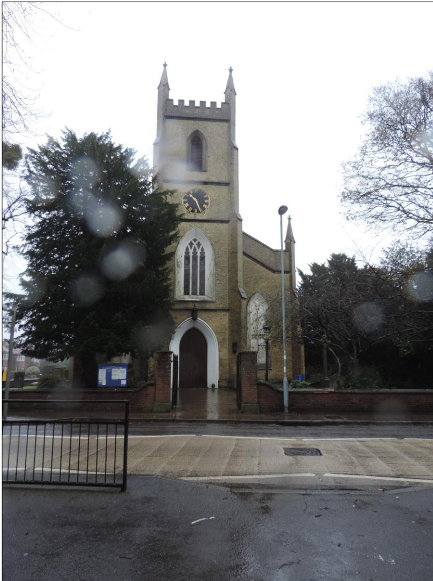
Photo 1 South-west access to Shirley Parish Church (St James)
