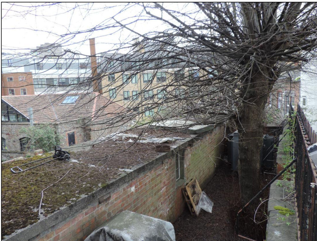
Photo 2 SE facing view of Project Site.
