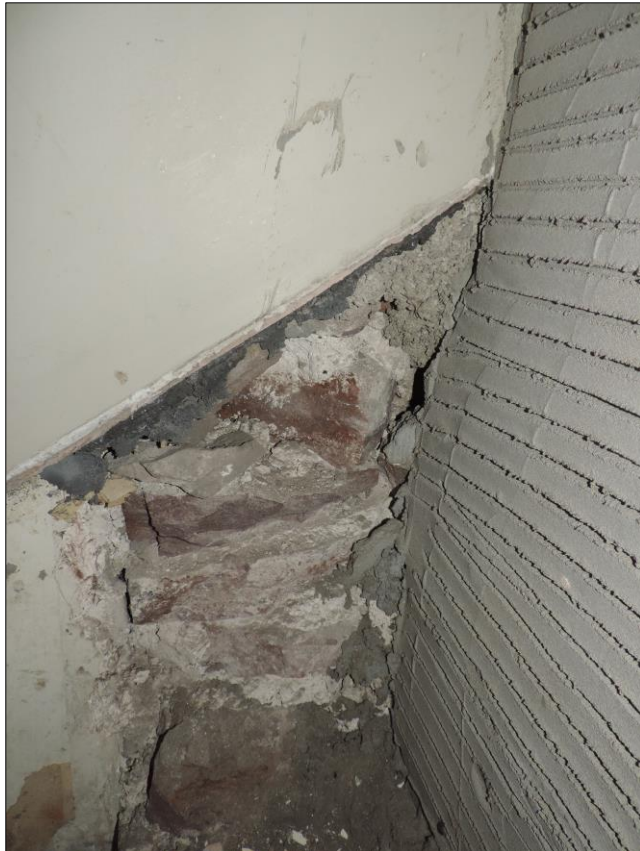
Photo 7 Southwest facing view of random Rubblestone fabric of 18 th century property.
