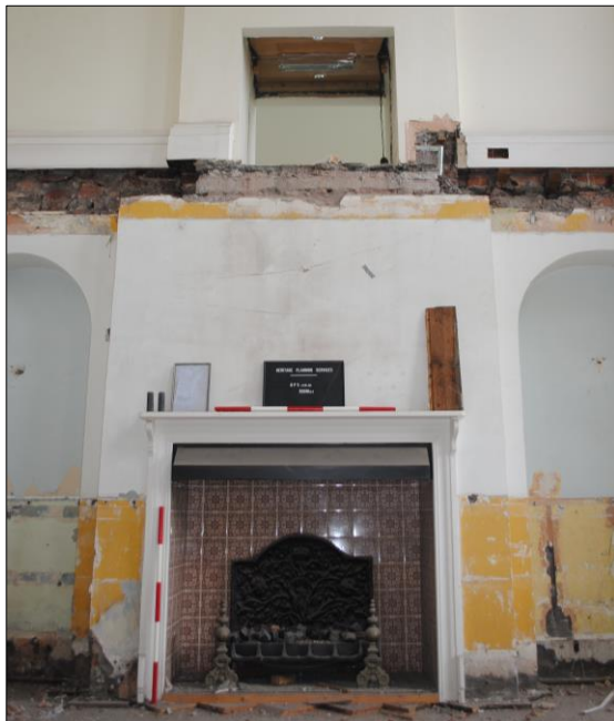
Photo 18 Southeast view of fireplace (scales 2 x 1m)
