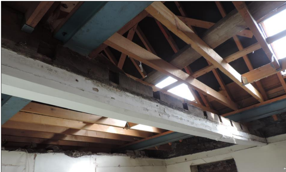
Photo 3 Detail of early chamfered beam beneath modern roof.
