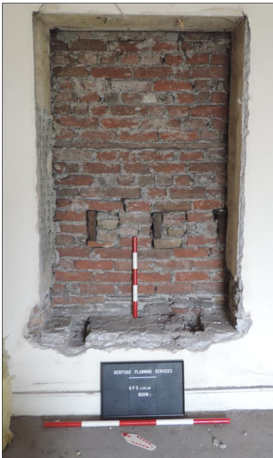
Photo 1 c. 1790 / 1800 Northwest bricked up window, northeast facing view (Scale 1 x 1m & 1 x 500mm).
