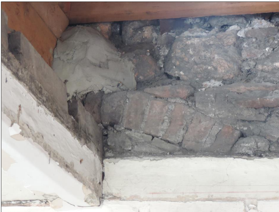
Photo 4 Detail of arch with beam slot and beam.
