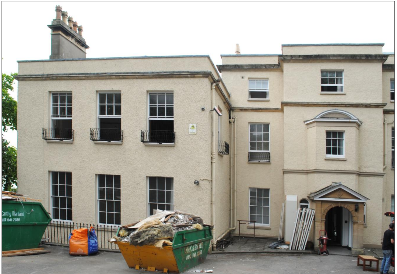
Photo 19 Northeast elevation of The Grove, with modern sand and cement render and paint finish.
