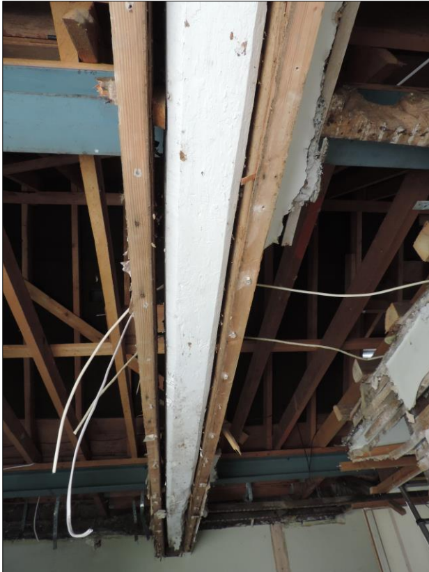
Photo 5 Detail of roof beam set into northeast wall
