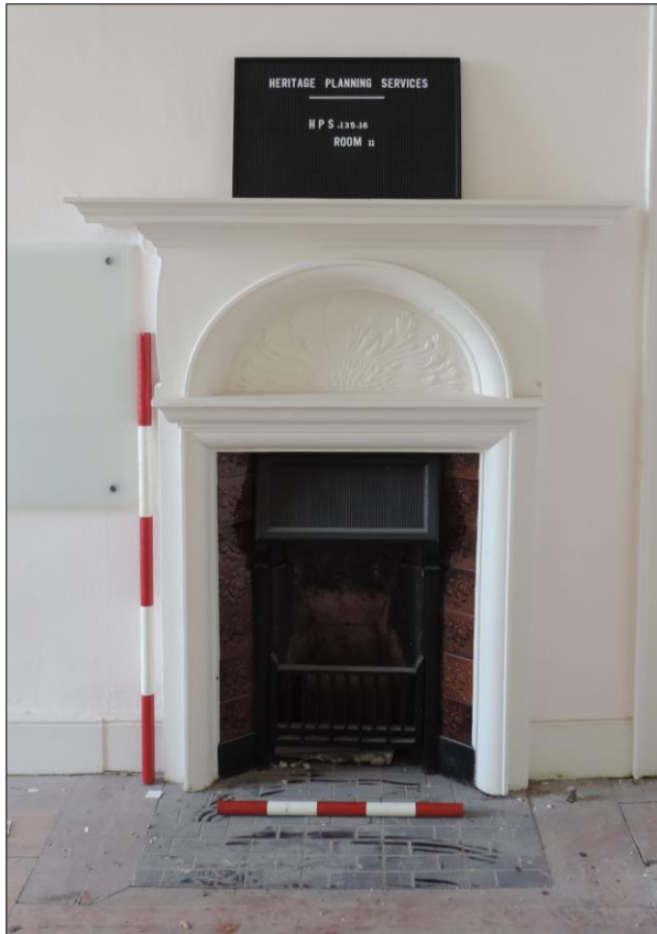
Photo 8 Modern fireplace surround, Room 11.
