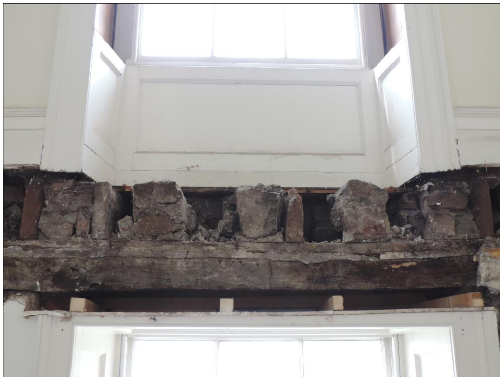
Photo 15 Southwest facing view of early 18 th century Limestone rubble joist pockets.
