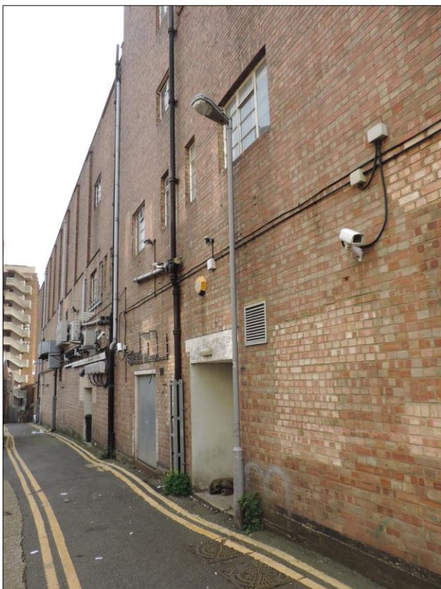
Photo 3 Restricted view of northwest facing elevation from Lancret's Path.
