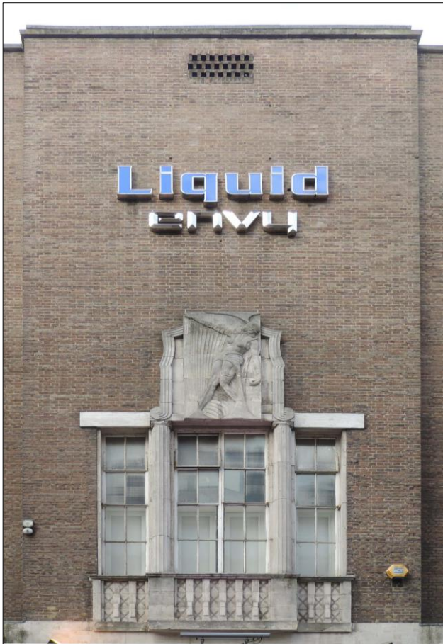
Photo 2 East facing elevation of the former Union Cinema, first floor detail.
