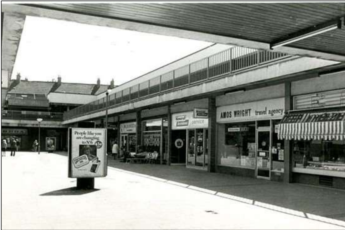
Figure 10 Duckworth Square Shopping centre c.1977.
