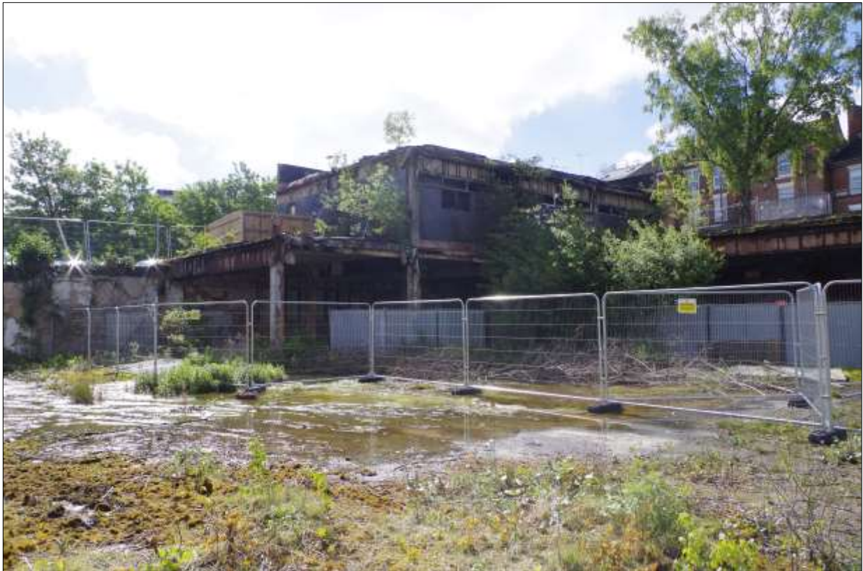
Photo 4 Southeast facing view toward part demolished structures bordering Macklin Street.
