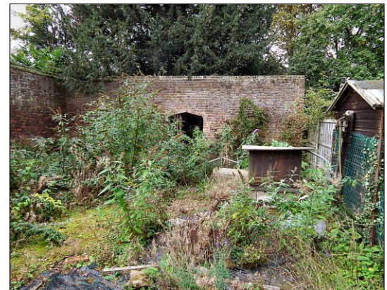
Photo 10. Interior of the walled garden, looking west. No scale.
