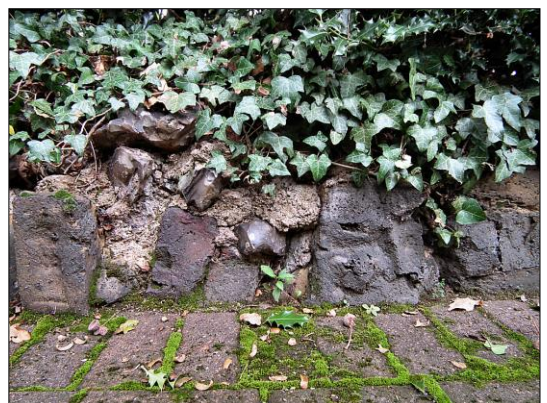
Photo 9. Detail of the low retaining wall, looking east.
