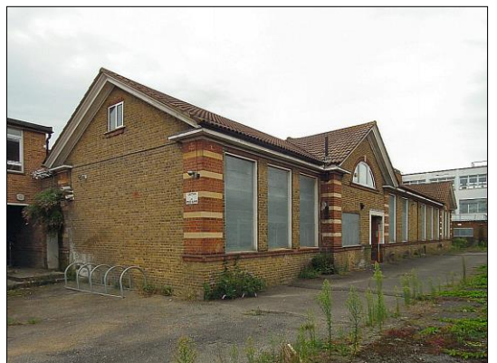
Photo 4. North and west faces of Block F.1, with parts of F.2 (left) and F.3 (far right).
