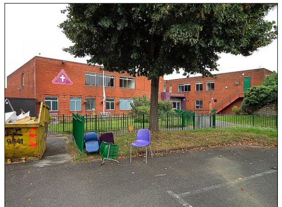
Photo 5. Blocks E (left) and D (right), looking NE from the visitor car park off Old Dover Road.
