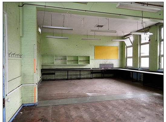
Photo 7. Interior view of a classroom, looking south. Scale 2m.
