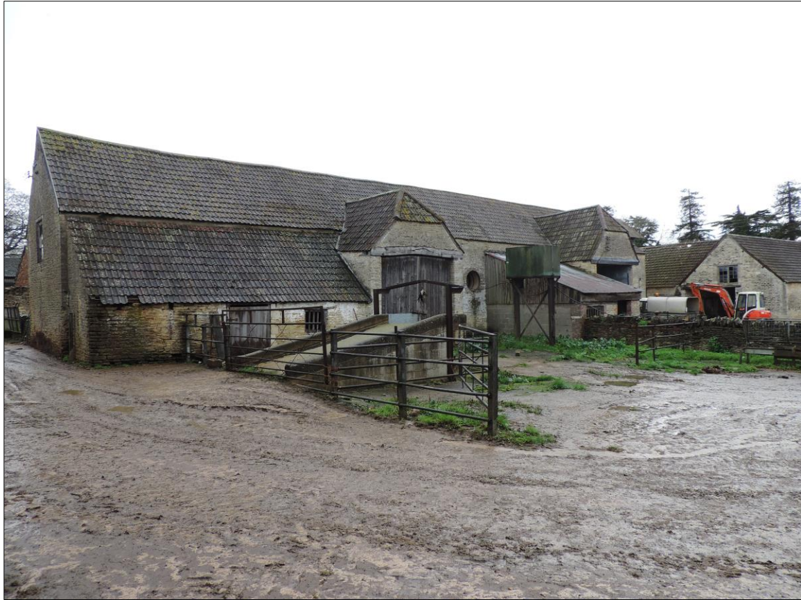
Photo 1 SSE facing view of the threshing barn
