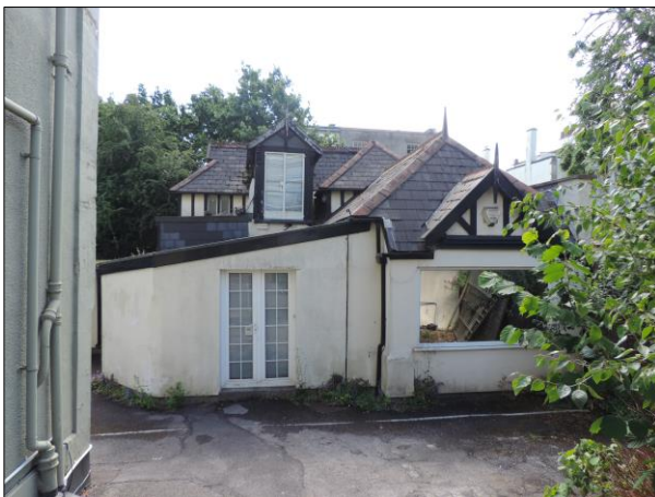
Photo 5 Southeast facing view of the Coach House from driveway. Enclosed courtyard with mono pitch roof is evident to the left.
