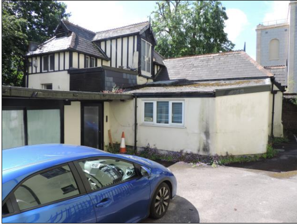
Photo 6 SSE facing view of Coach House from yard / parking bay. The timber framed hayloft dormer and pitched ventilation add to the decorative effect.
