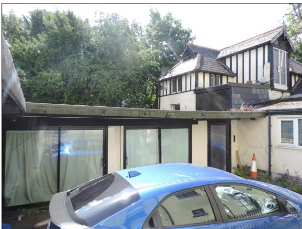
Photo 3 SSE facing view of lean to abutting the Coach House.
