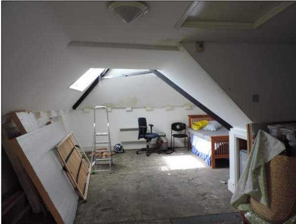
Photo 10 Converted loft space. Southwest facing view with original skylight location visible to the rear left of the shot.
