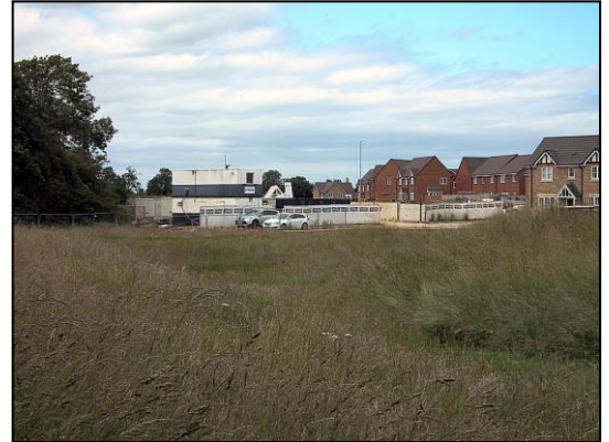
Photo 4. View of the construction compound on Area B, looking north.
