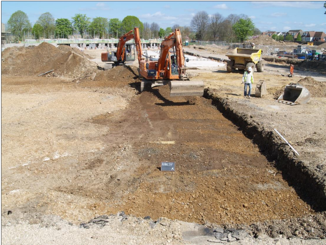
Photograph 17 North facing view of ground reduction
