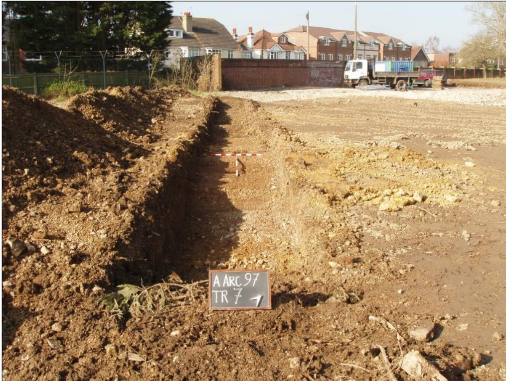
Photograph 12: Trench 7 NW Facing View (Scales 1 x 1m & 1 x 2m)
