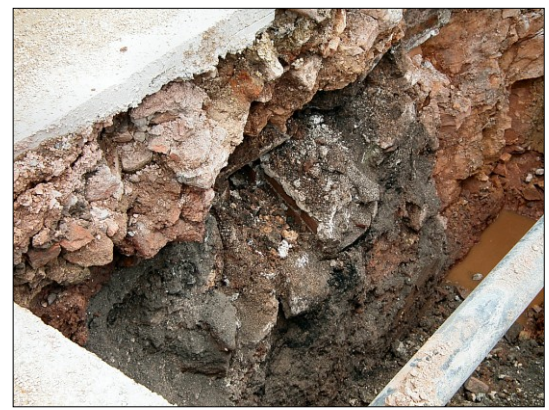
Photo i. Truncated brick-lined culvert in north facing section, looking southwest.
