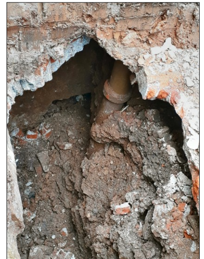
Photo c. Vertical ceramic pipe in chamber, looking west.
