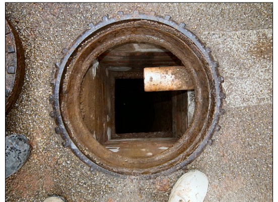
Photo f. Detail of the well access hatch.
