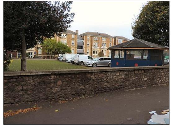
4.7. It was evident the land on the north side of the wall was raised above the level of the driveway, indicating the wall has a retaining function.
